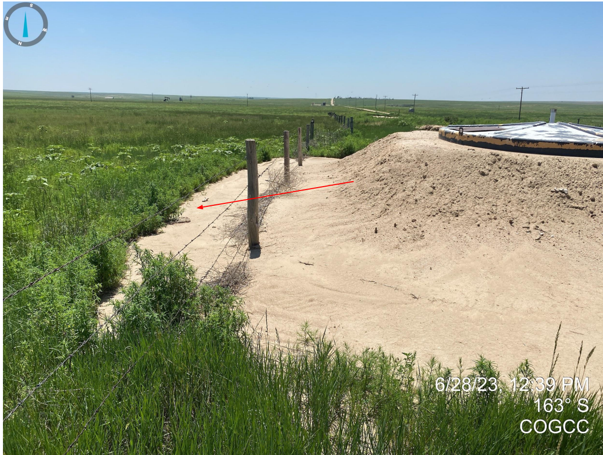
Photo 11. Soils around partially buried tank do not appear to be stabilized with evidence of off-location sediment transport. Additional maintenance or BMPs are required to come into compliance with Rule 1002.f.
