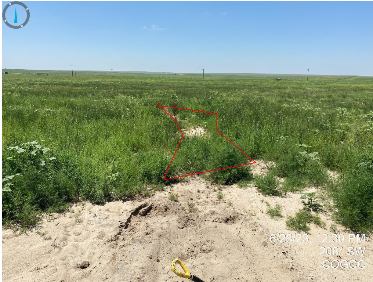
Photo 4. See comments in Photo 1. Additionally, rill erosion was observed on the northwest guy line anchor; soil do not appear to be properly stabilized.
