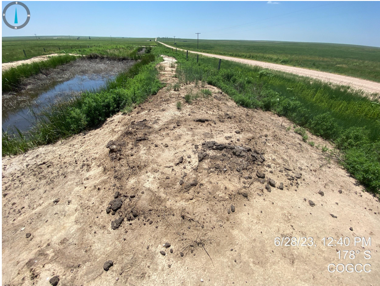
Photo 13. Stained soil observed on pit walls/berms will need to be properly cleaned up.
