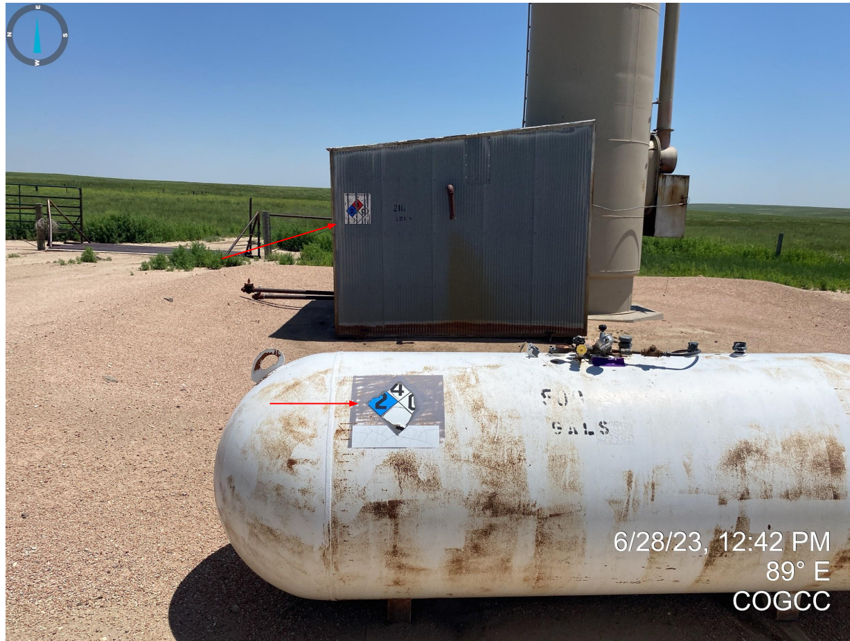
Photo 16. NFPA placards are peeling, faded, cracked, and/or not legible.
