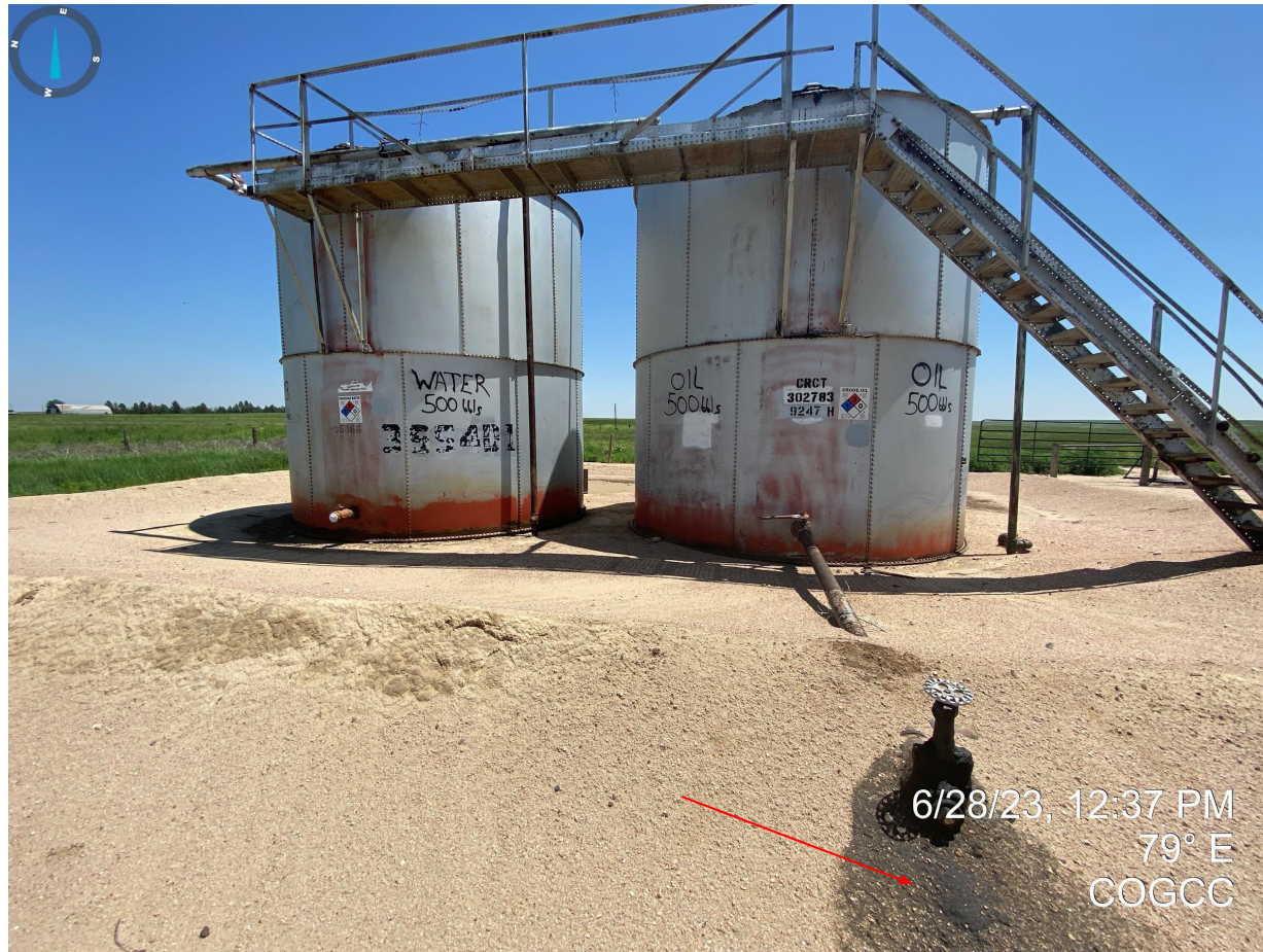
Photo 10. Stained soil around loadout line.
