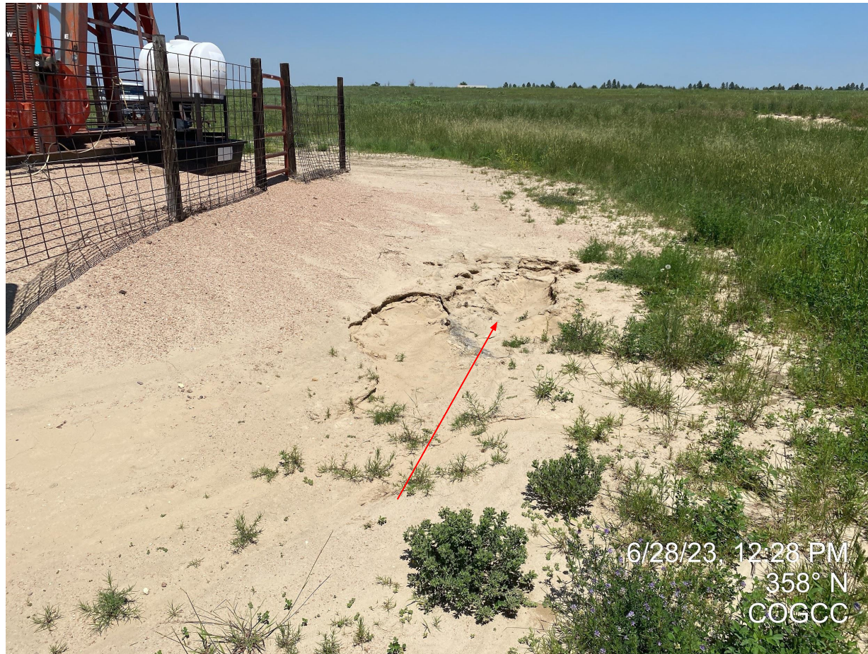
Photo 6. Unstabilized production areas will require maintenance and/or additional BMPs (roadbase, etc).
