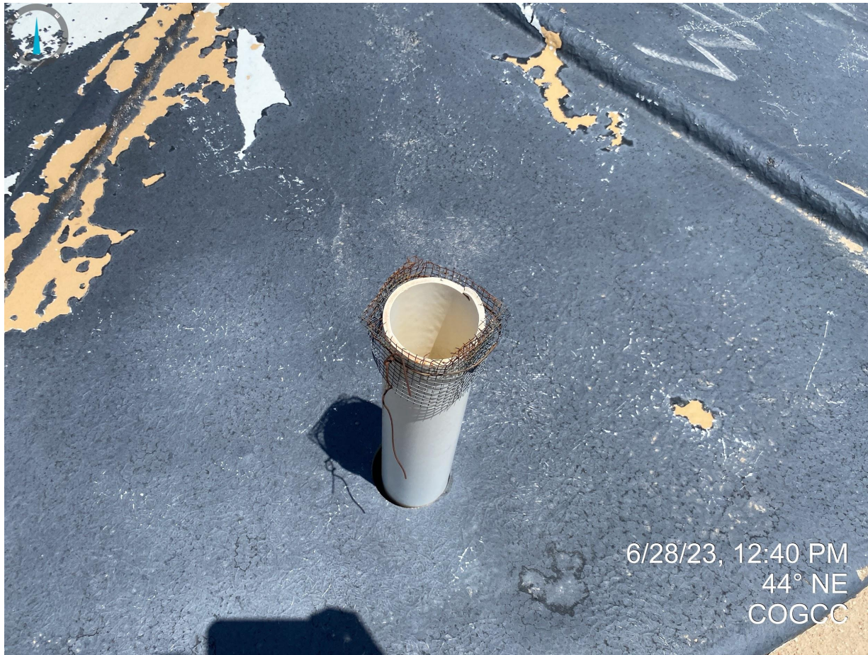
Photo 18. Wildlife protection equipment needs replacement/repair on partially buried tank.
