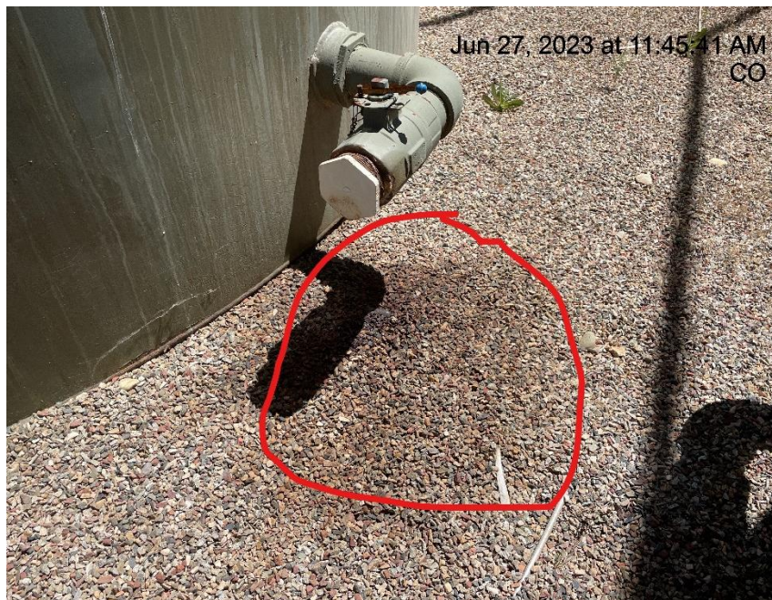
Photo # 2120 Stained gravel in secondary containment
