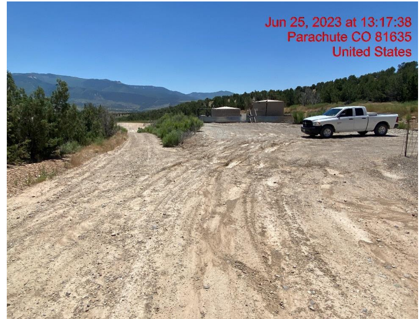
Insufficient Vehicle Tracking BMPs at Location Entrance/Exit – Photo #04818
