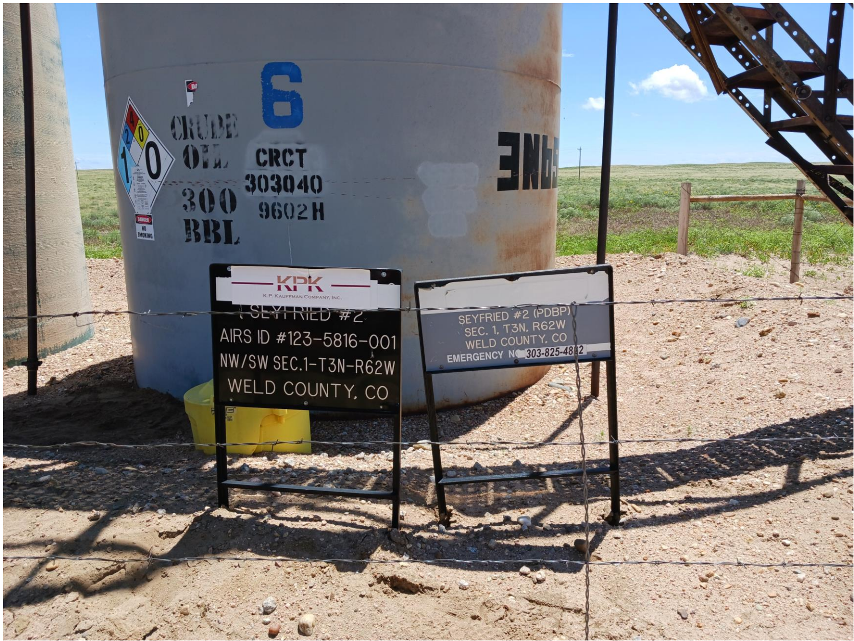
Figure #1 Tank labels have been installed;
