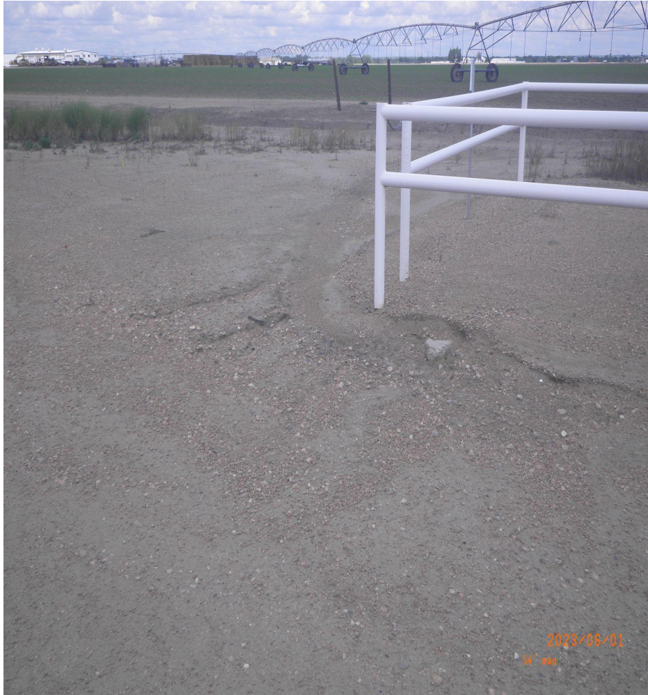
Photo 3. Rill erosion located on south eastern edge of the tank battery.
