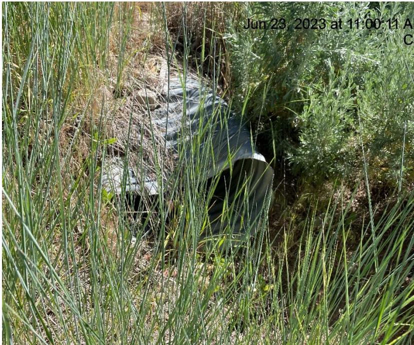
Photo # 1673 Culvert needs maintenance/culvert crimped/reduced capacity
