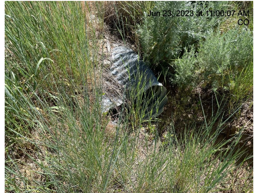
Photo # 1672 Culvert needs maintenance/culvert crimped/reduced capacity
