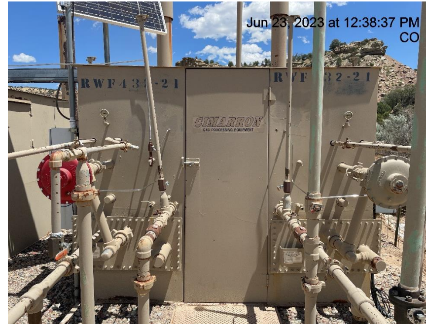
Photo # 1733 Meter calibration info not conspicuously posted
