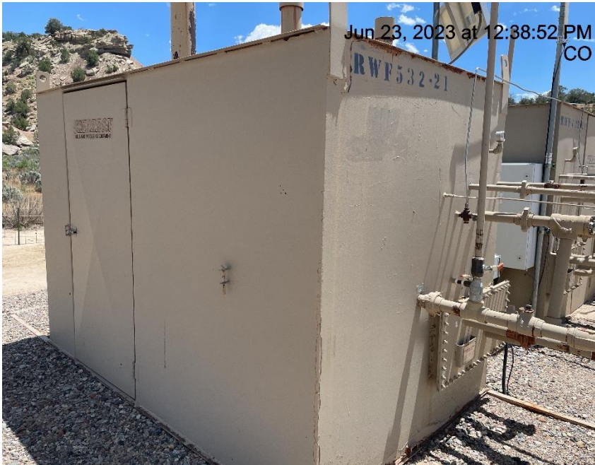
Photo # 1734 Meter calibration info not conspicuously posted
