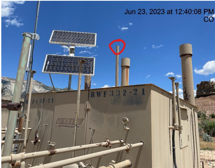
Photo # 1737 Open ended pipe on top of separator unit
