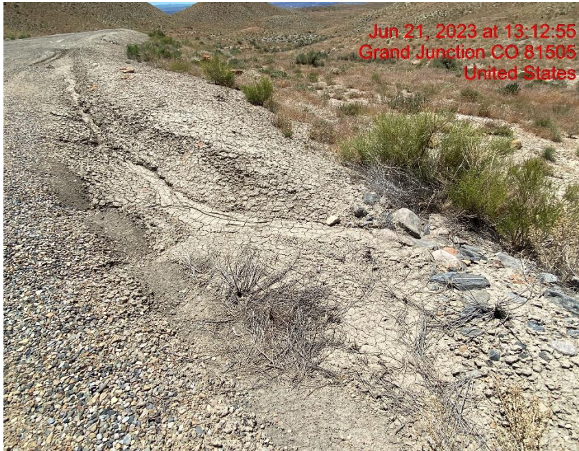
Rill Erosion on Access Road/Rip Rap BMP Needs Maintenance – Photo #04706
