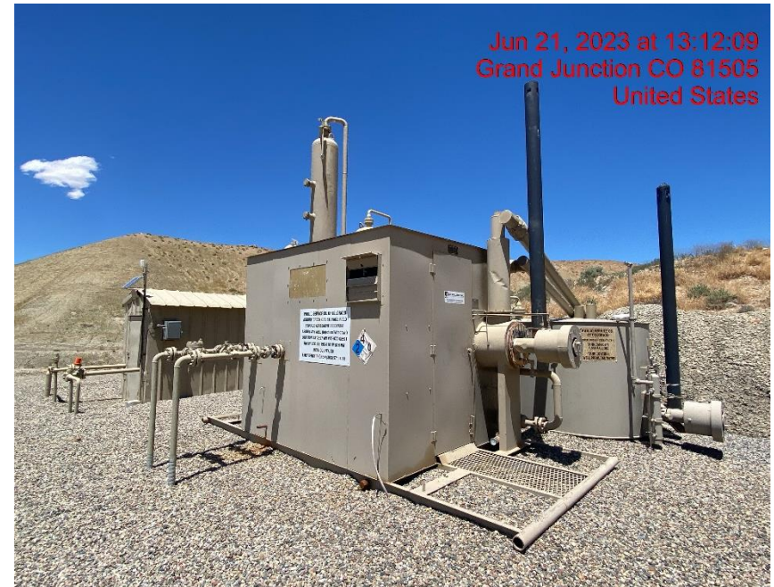
Separator/Dehydrator/Produced Water Tank – Photo #04703
