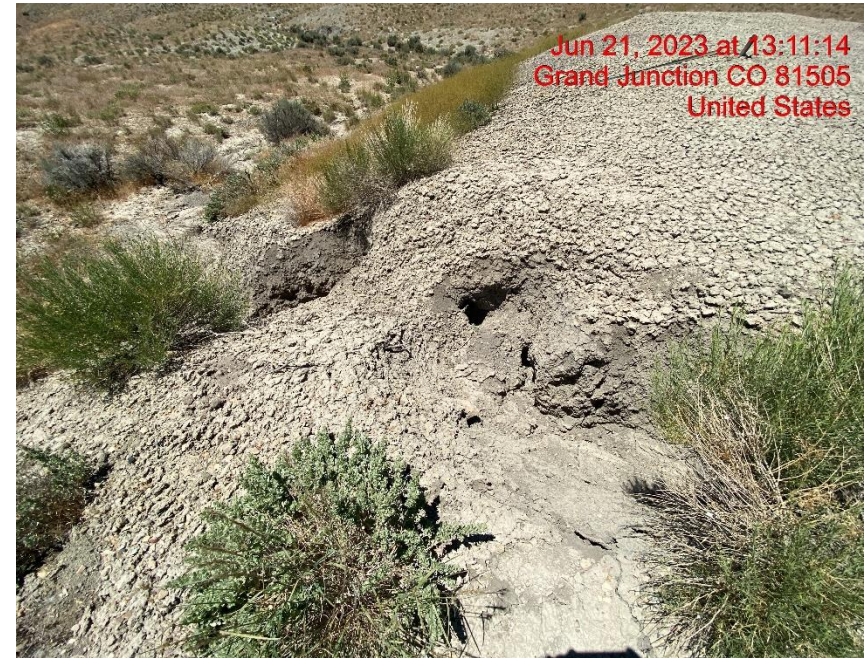
Sediment Trap Washed Out & Needs Maintenance – Photo #04700
