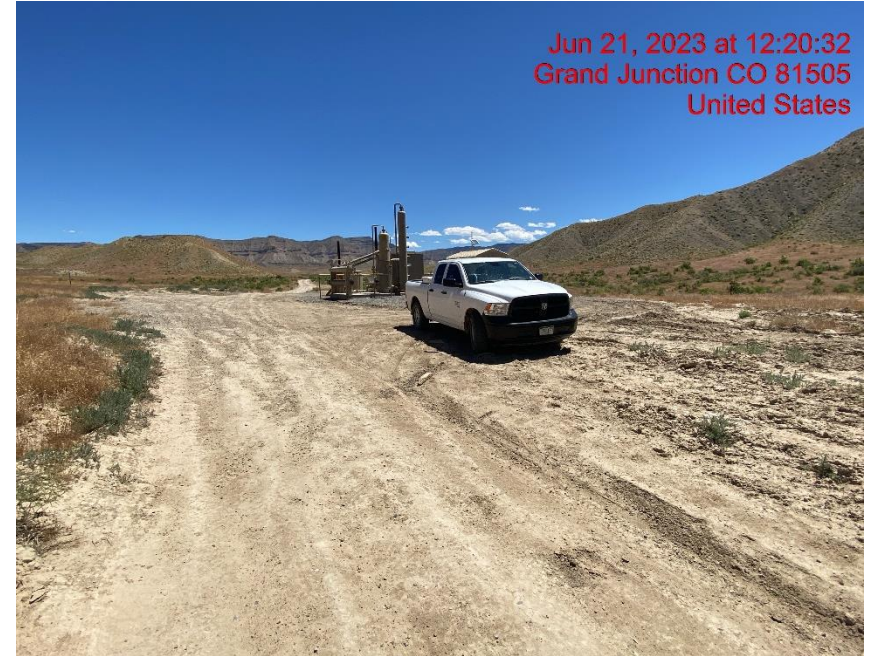
Insufficient Vehicle Tracking BMPs at Location Entrance/Exit – Photo #04669
