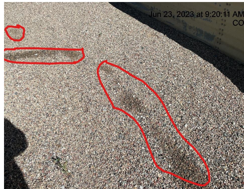
Photo # 1509 Stained gravel in secondary containment
