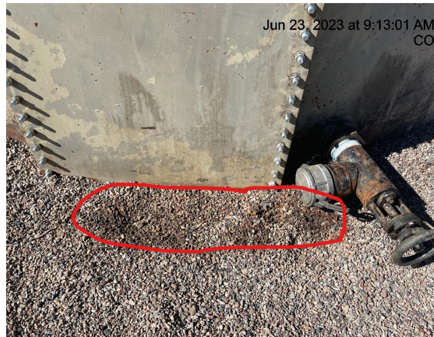
Photo # 1500 Stained gravel in secondary containment
