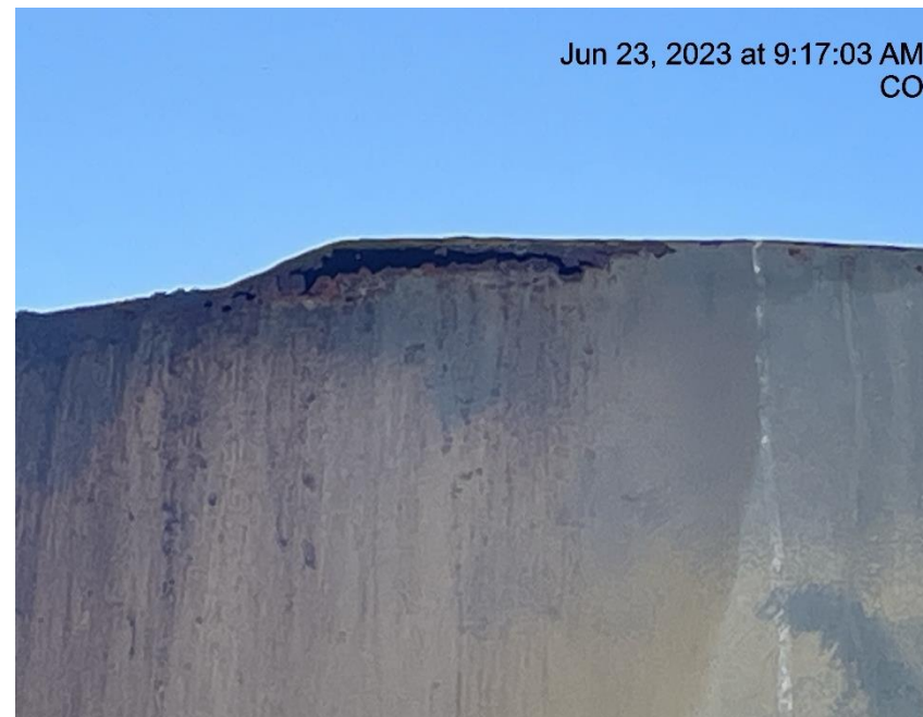
Photo # 1504 Hole in production tank/tank corrosion
