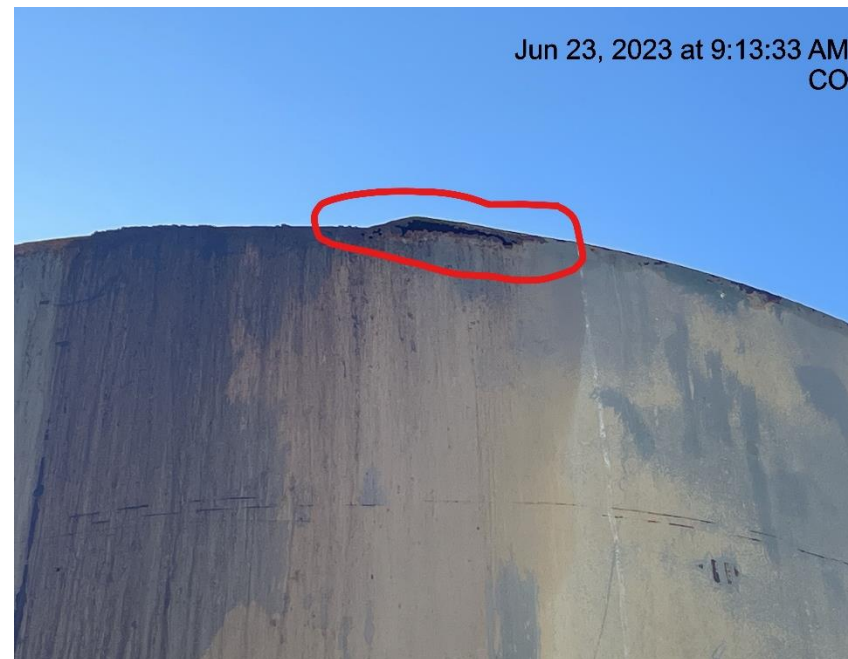
Photo # 1501 Hole in production tank/tank corrosion
