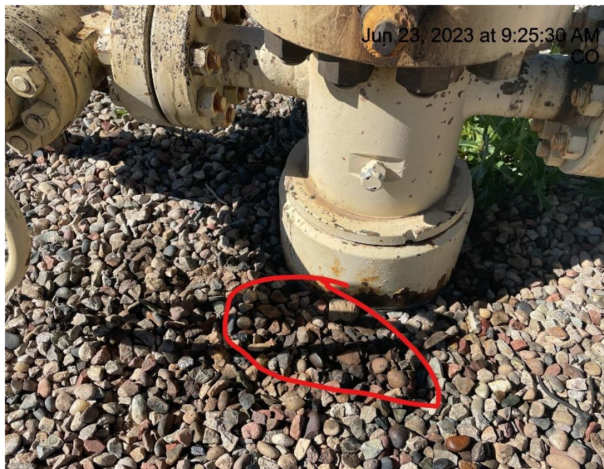
Photo # 1521 Stained soils & gravel (Couey 31-7 wellhead)
