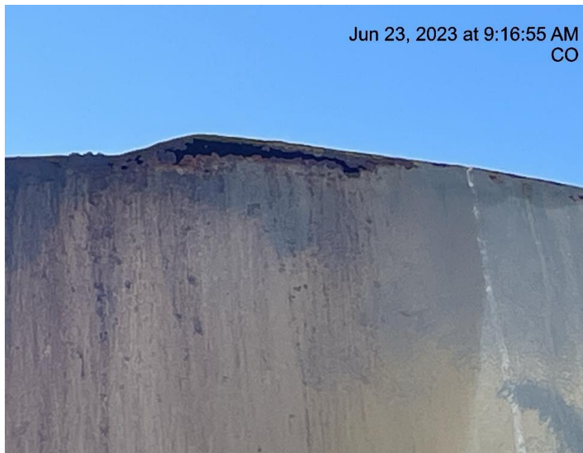
Photo # 1503 Hole in production tank/tank corrosion
