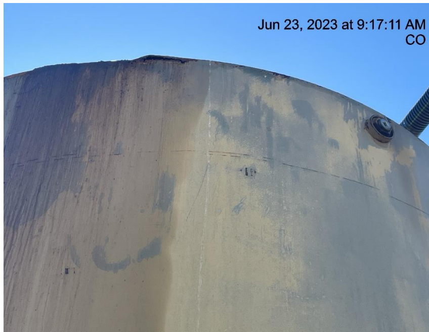
Photo # 1505 Hole in production tank/tank corrosion
