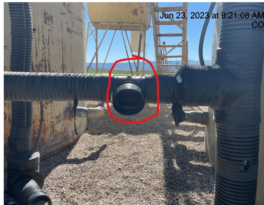
Photo # 1515 Flowline heating insulation open ended
