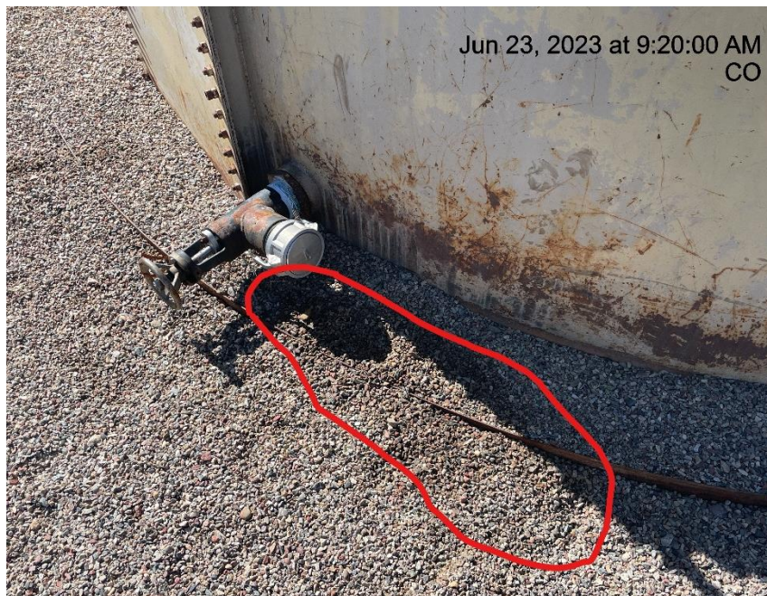
Photo # 1507 Stained gravel in secondary containment
