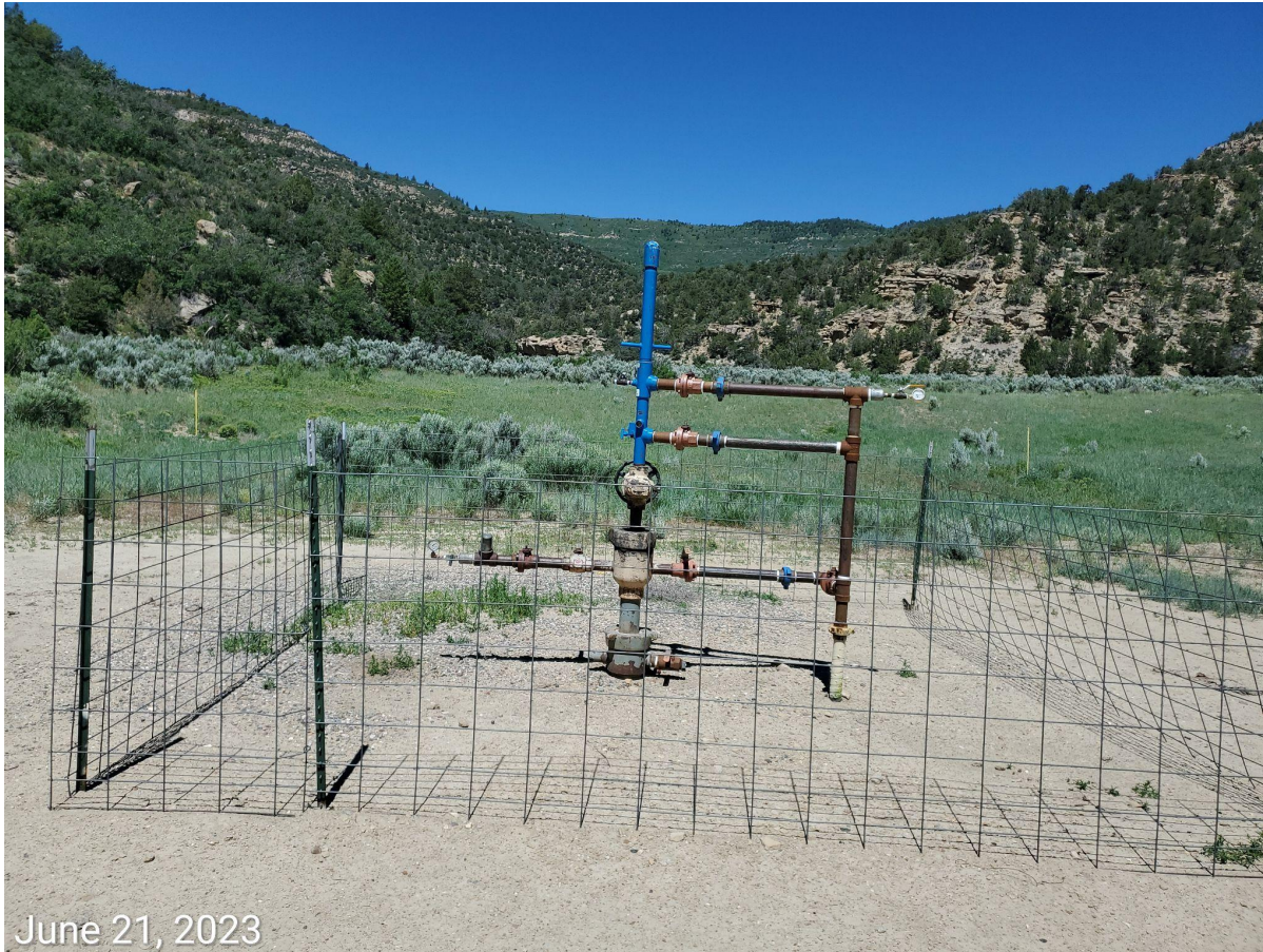
Photo 3: Wellhead signage remains missing.
