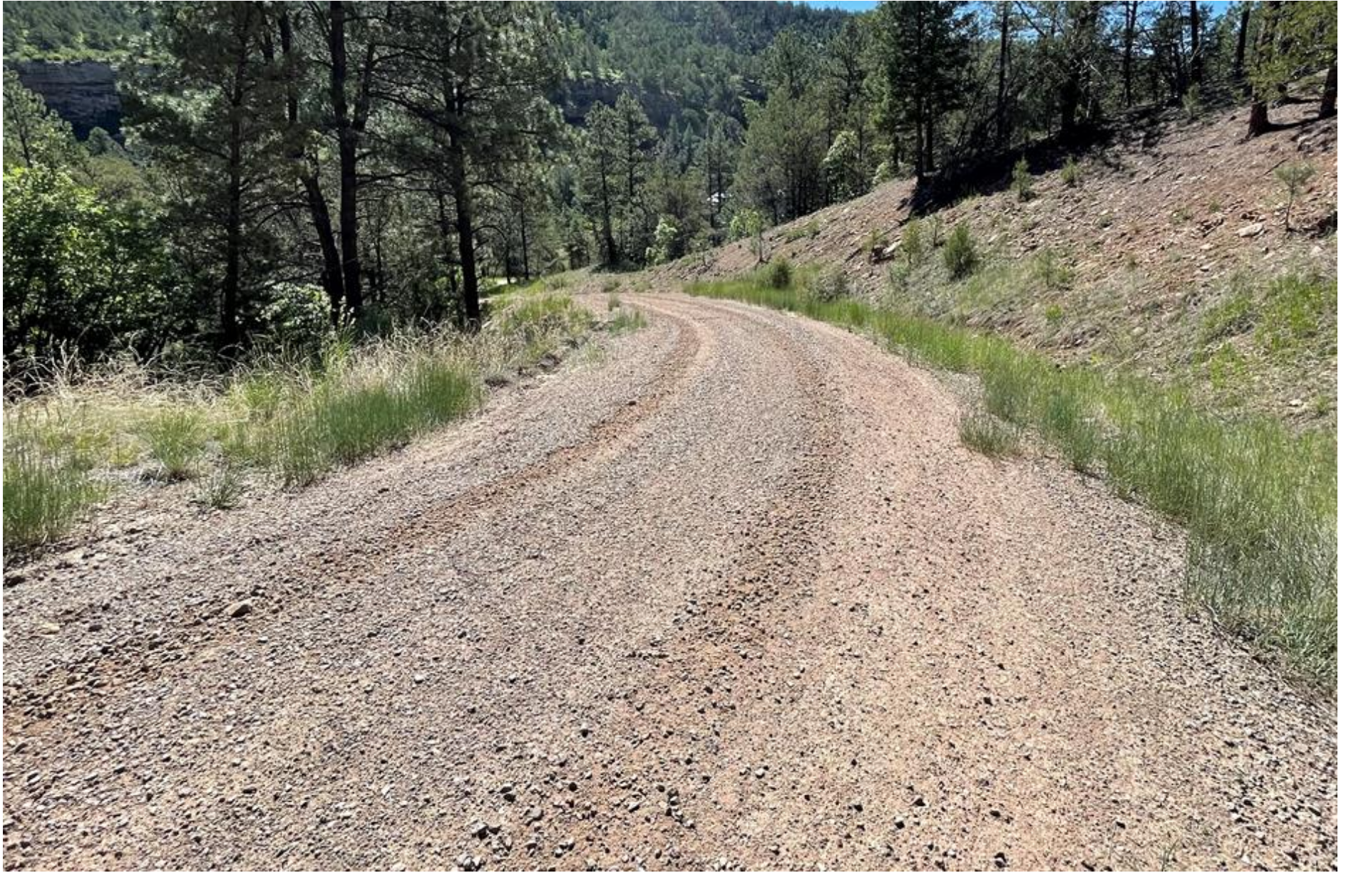
PHOTO 1: THE RILLING/STORMWATER DAMAGE ON THE ACCESS ROAD HAS BEEN REPAIRED AND GRADED.
