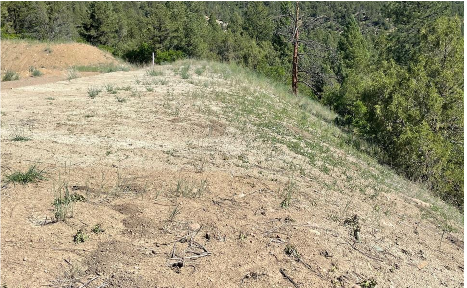
PHOTO 3: THE FILL SLOPE HAS BEEN REDEFINED, TRACKED, AND HYDRO SEEDED TO PROMOTE STABILIZATION AND VEGETATIVE GROWTH. THE LOCATION HAS ALSO BEEN TREATED FOR ALL NOXIOUS WEEDS AND WILL BE FURTHER MONITORED THROUGHOUT THE GROWING SEASON.
