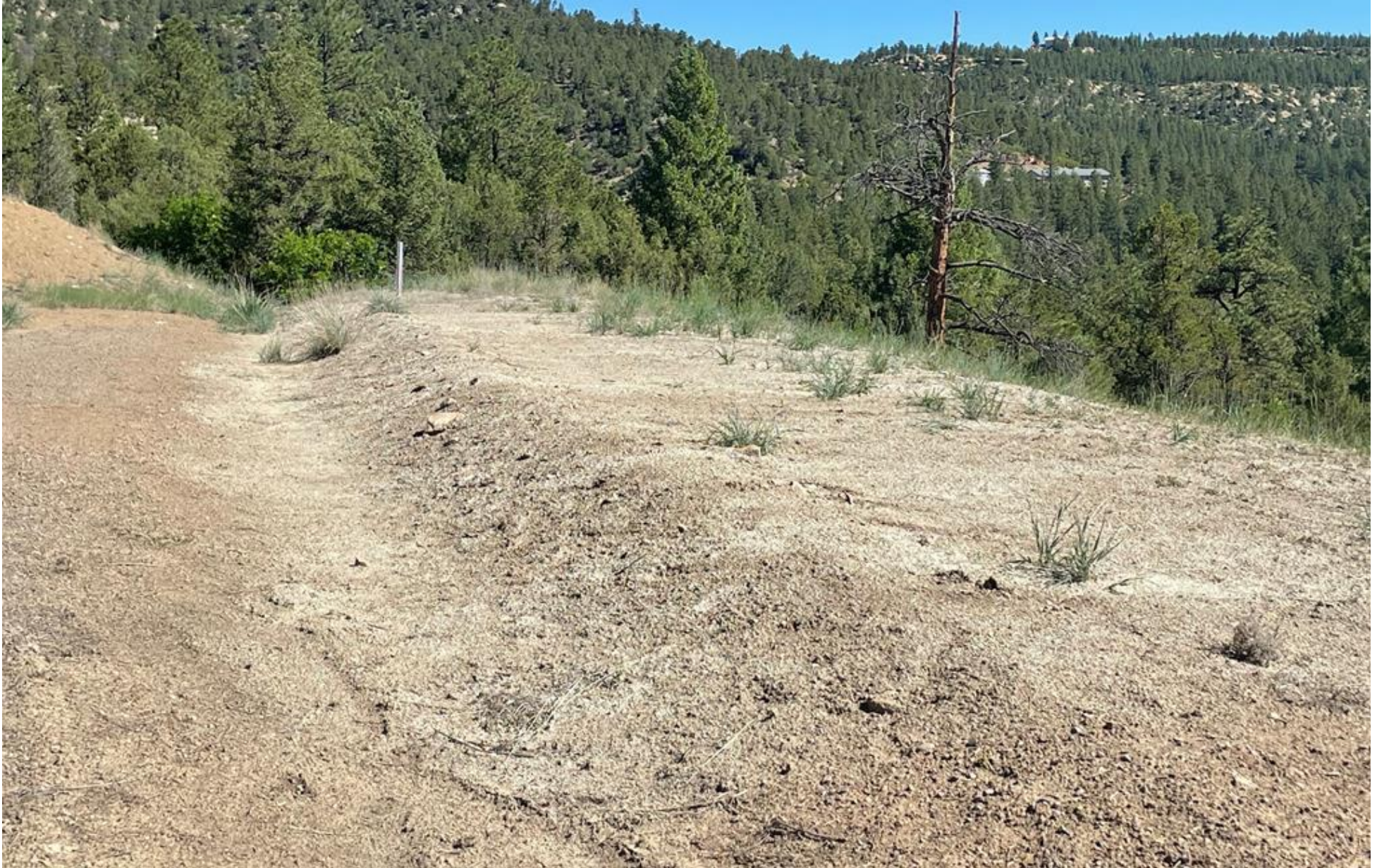
PHOTO 2: THE FILL SLOPE HAS BEEN REDEFINED, TRACKED, AND HYDRO SEEDED TO PROMOTE STABILIZATION AND VEGETATIVE GROWTH. THE LOCATION HAS ALSO BEEN TREATED FOR ALL NOXIOUS WEEDS AND WILL BE FURTHER MONITORED THROUGHOUT THE GROWING SEASON.
