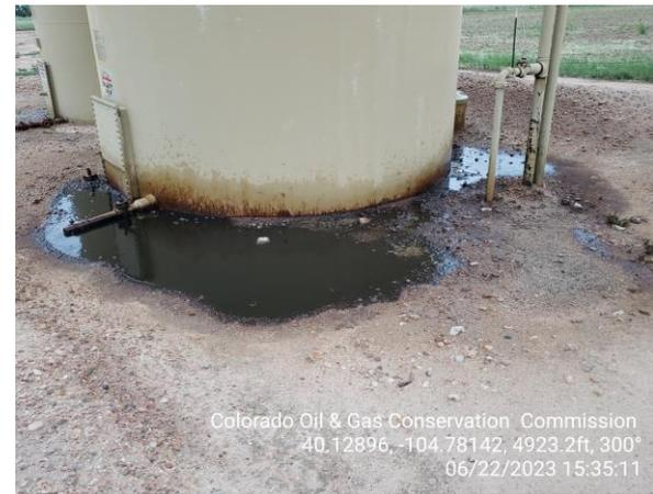
**Photo 9 Spill on the east side of the East Crude tank.**
