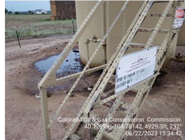
Photo 7 Spill on the east side of the East Crude tank.
