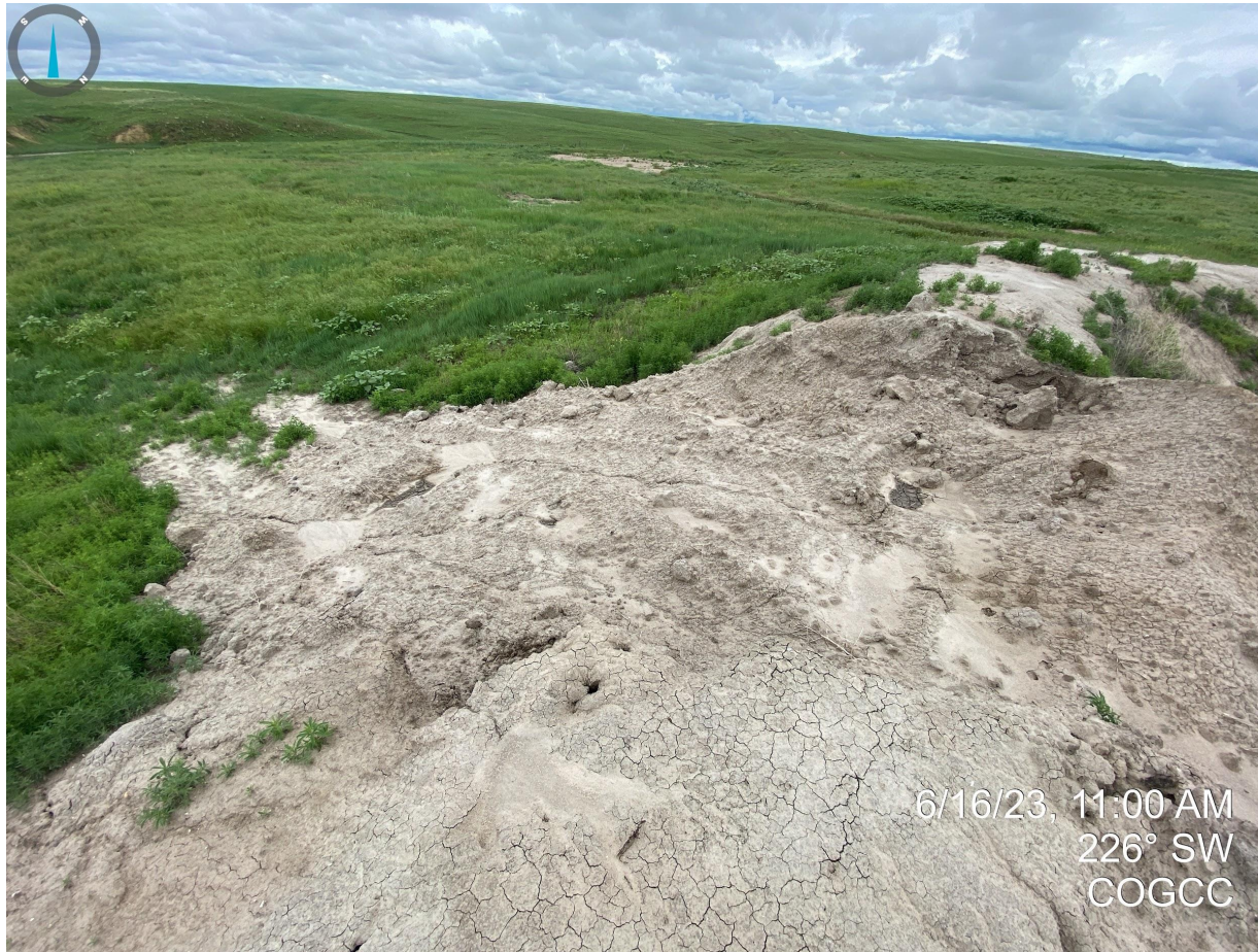
Photo 5. Southern pit wall, There is evidence of recent equipment tracking on the outside of the berm; the material has been left unconsolidated and is beginning to migrate into the surrounding areas. Additional stormwater BMPs are required to stabilize and contain the material from migrating into adjacent areas, especially if the material is impacted.
