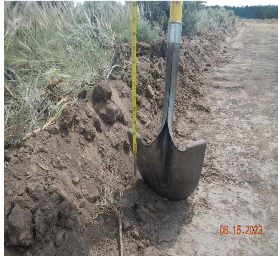
Photo 10. Northeast corner of the location facing southwest. It appears topsoil was being salvaged around 6-8" in some areas and less in other areas but salvaging was still ongoing.
