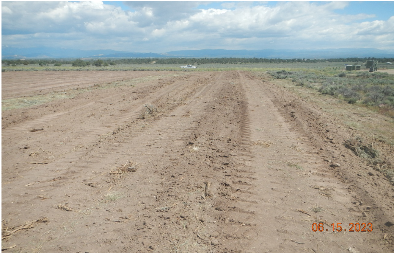
Photo 6. Standing on the topsoil pile facing north. There are no perimeter stormwater controls installed. Stormwater controls should have been installed prior to construction.
