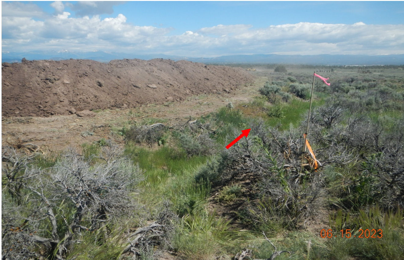
Photo 4. Southeast side of the location facing north. There are no perimeter stormwater controls installed. Topsoil is being paced near the drainage swale shown at red arrow which runs along the edge of the disturbance.
