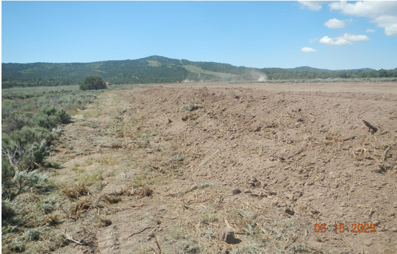
Photo 5. Northeast side of the location facing south. There are no perimeter stormwater controls installed. Stormwater controls should have been installed prior to construction. Topsoil is being stripped and stockpiled along the east side of the location.
