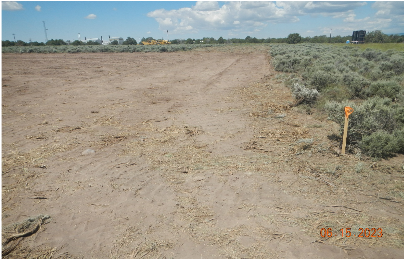
Photo 7. Northeast side of the location facing west. There are no perimeter stormwater controls installed. Stormwater controls should have been installed prior to construction. This is the downhill gradient slope of the location.
