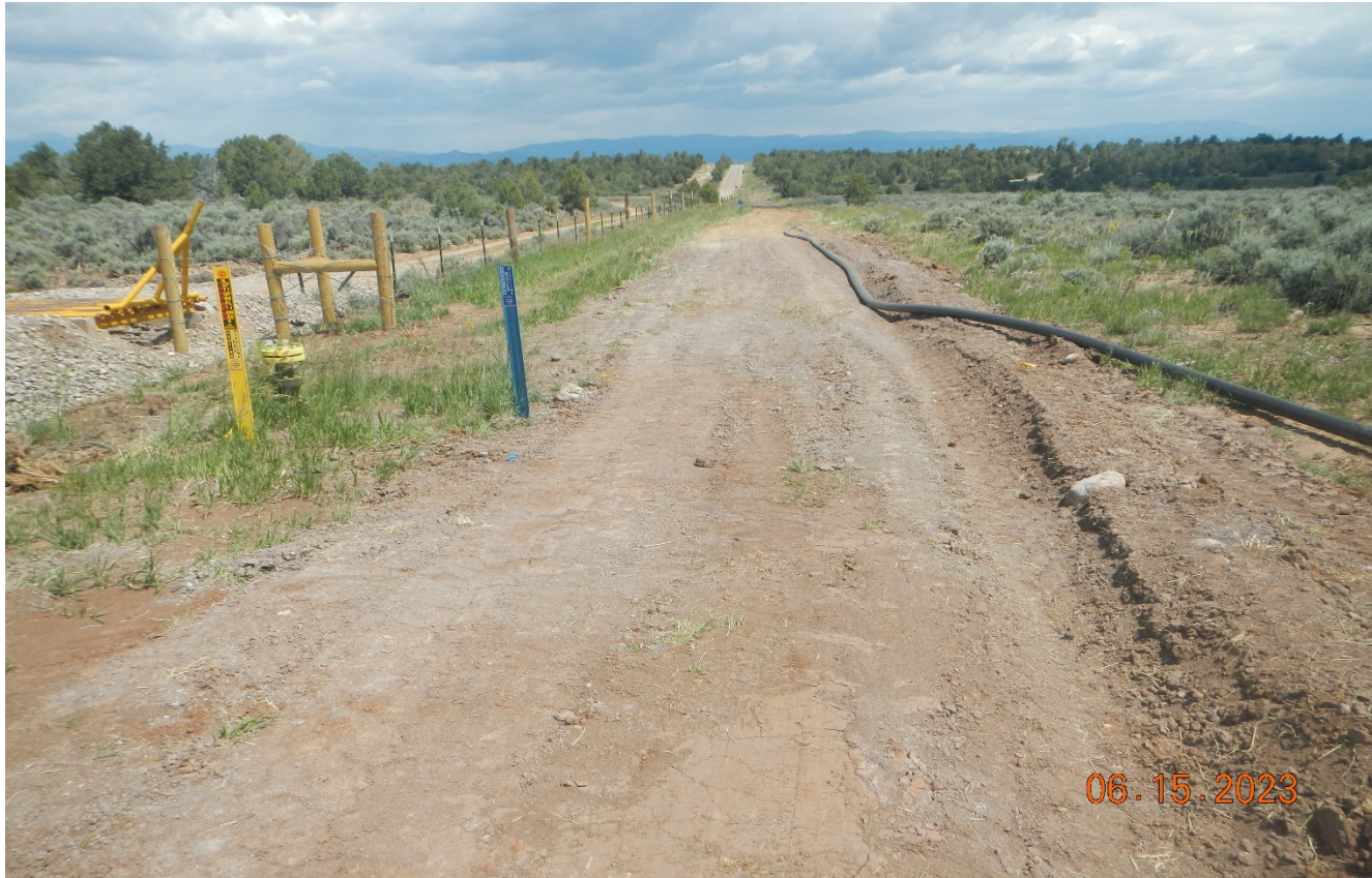
Photo 11. Facing north along the flowline disturbance. BMPs need to be installed along the flowline disturbance.
