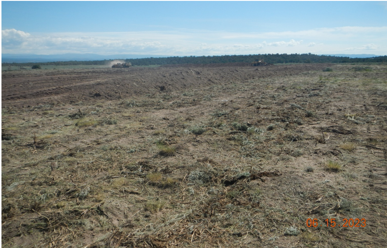
Photo 2. Standing at the southwest corner of the tank pad location facing northeast. Topsoil was in process of being stripped and stockpiled at the south and east side of the location.
