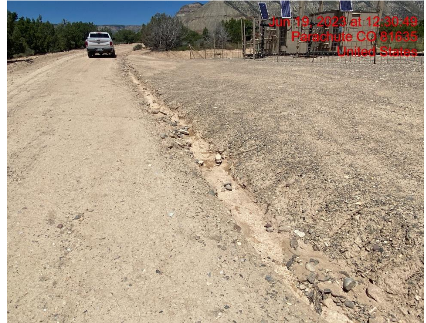
Insufficient Vehicle Tracking BMPs at Location Entrance/Exit – Photo #04603
