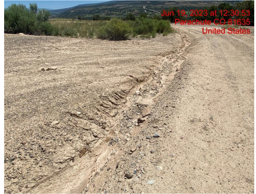
Rill Erosion/Ditch Full of Sediment/Needs Maintenance – Photo #04604
