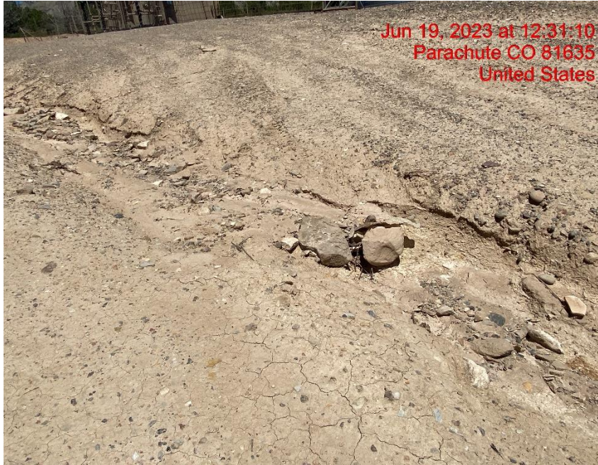
Rill Erosion/Check Dam Needs Maintenance – Photo #04605
