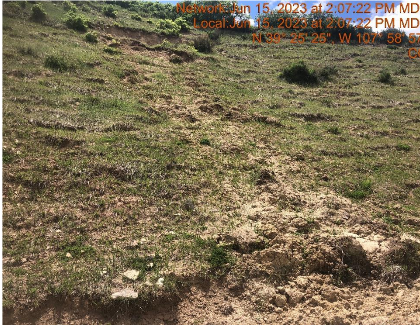
Photo #383 Cut slope lacks stabilization.
