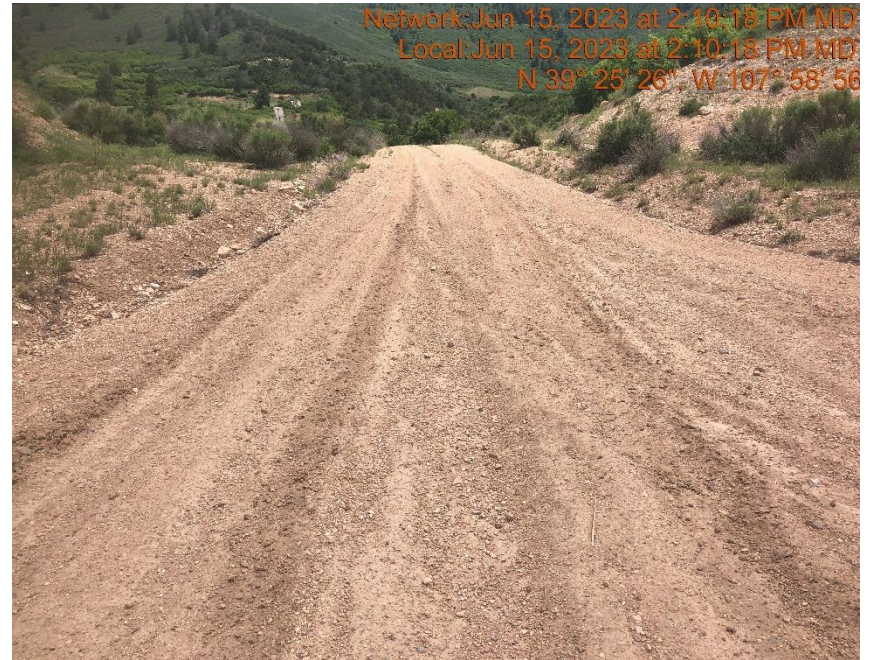
Photo #395 Insufficient tracking BMP at entrance to location to minimize the transport of sediment.
