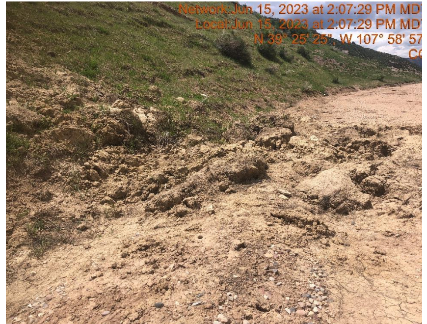
Photo #384 Run on to location not being controlled.
