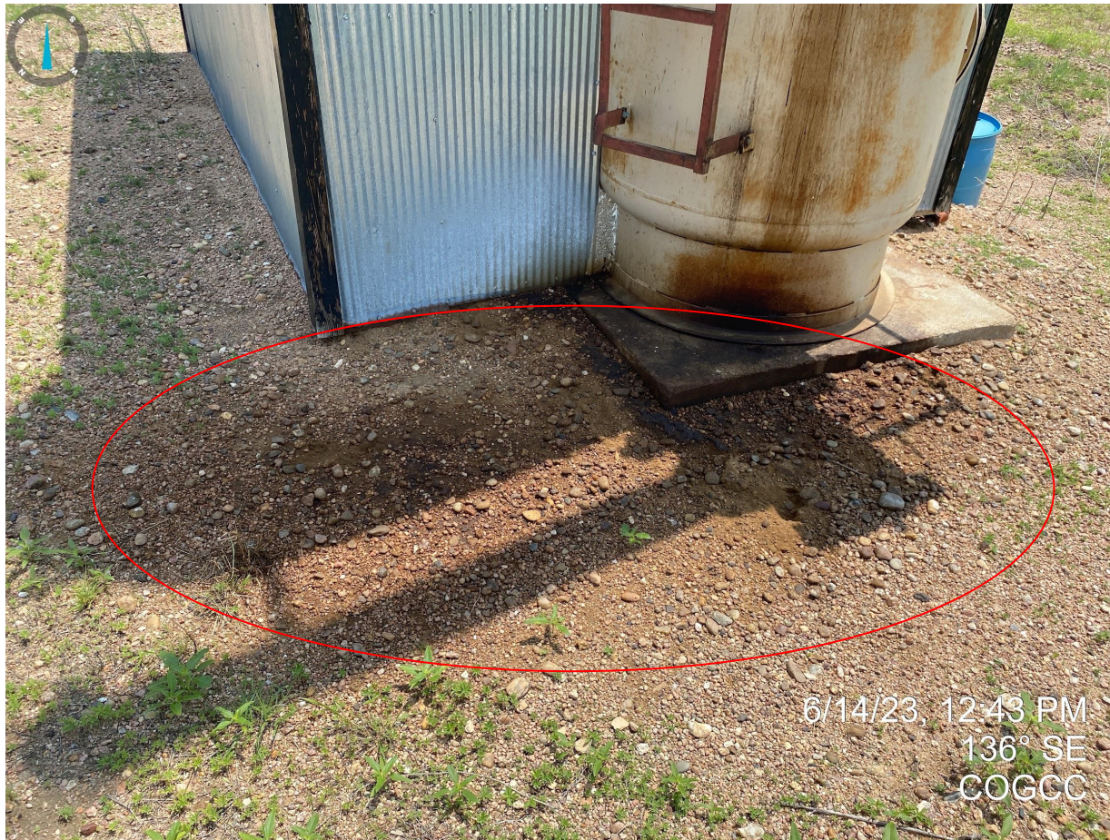
Photo 8. Stained soil observed around vertical heater treater requires proper cleanup and disposal per Rule 905.e.
