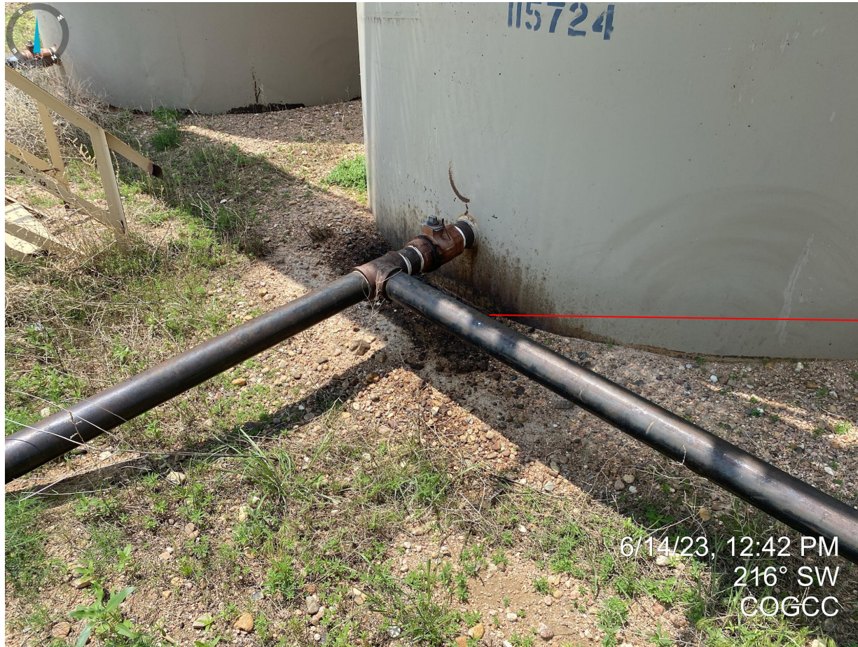
Photo 5. Stained soil was observed underneath connections at vertical tanks and will need to be properly cleaned up and disposed of per Rule 905.e.
