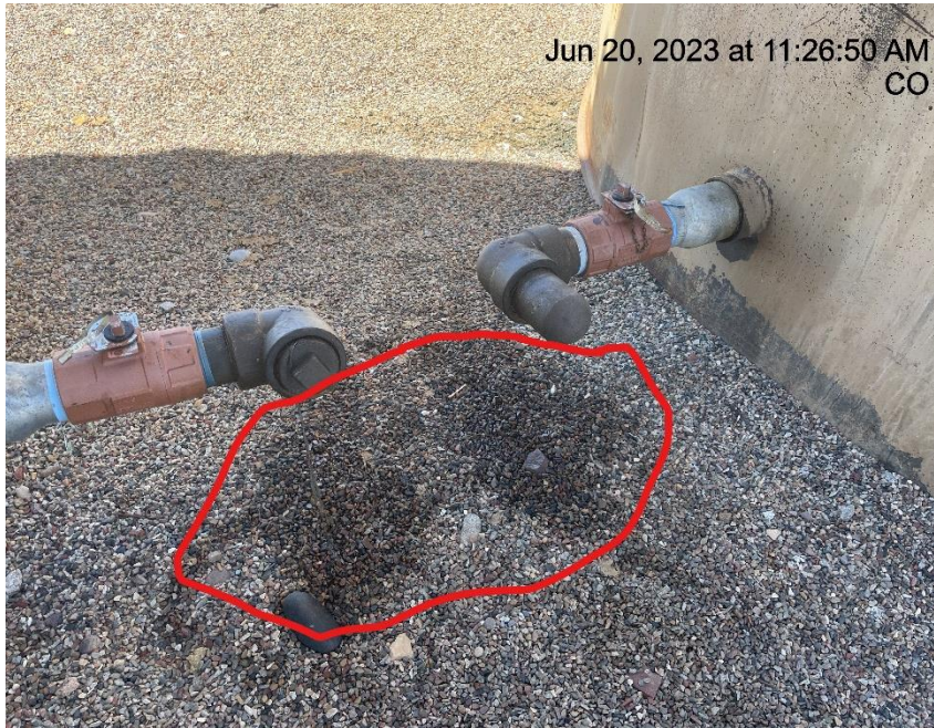
Photo # 1211 Stained gravel in secondary containment
