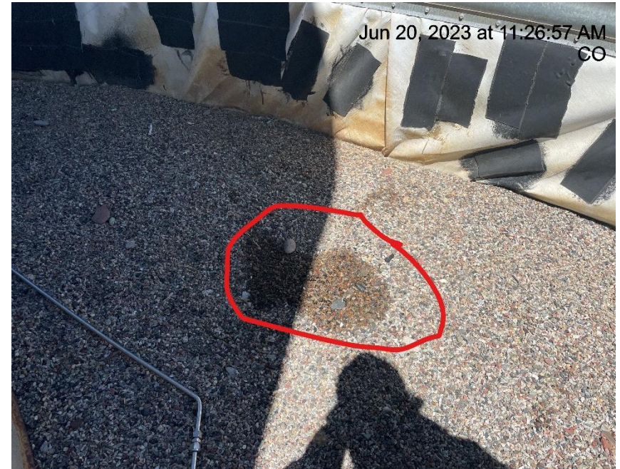
Photo # 1212 Stained gravel in secondary containment
