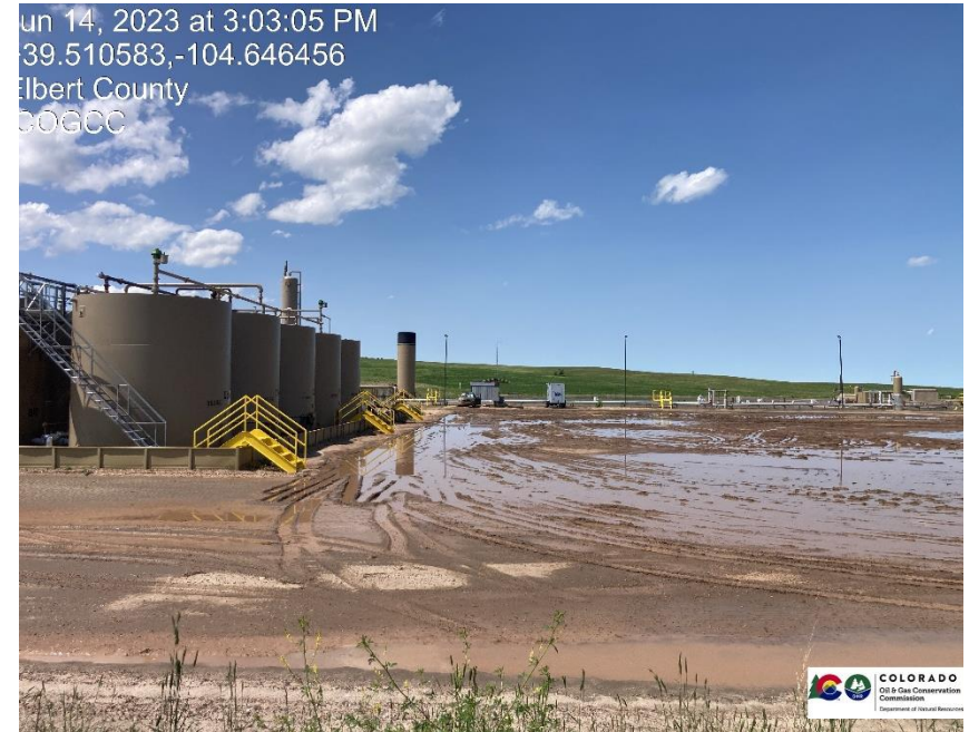
Pic 2 tanks, BMP failure on location, stormwater mitigation failure.
