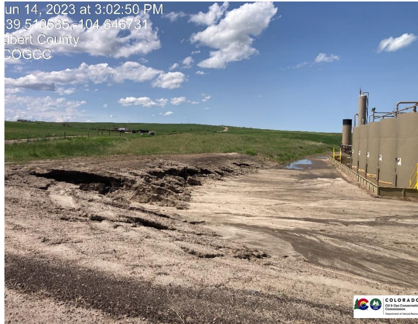
Pic 1 entrance to location, BMP failure, stormwater erosion on locaiton
