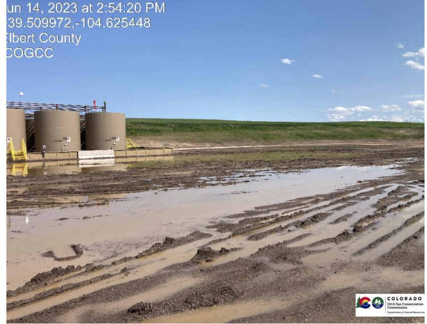
Pic 8 location BMP appear to be failing to control storm water.
