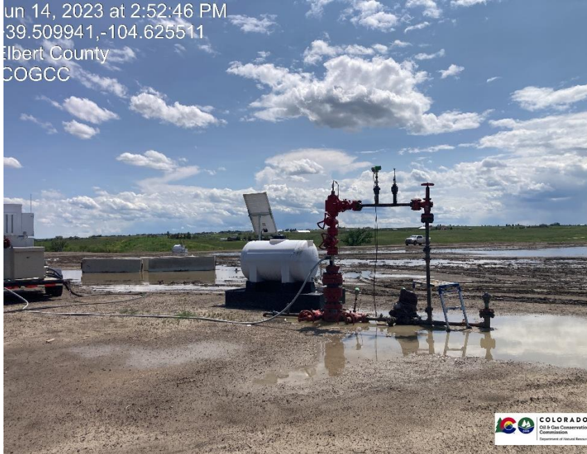
Pic 3 wellhead, no wellhead sign observed on wellhead
