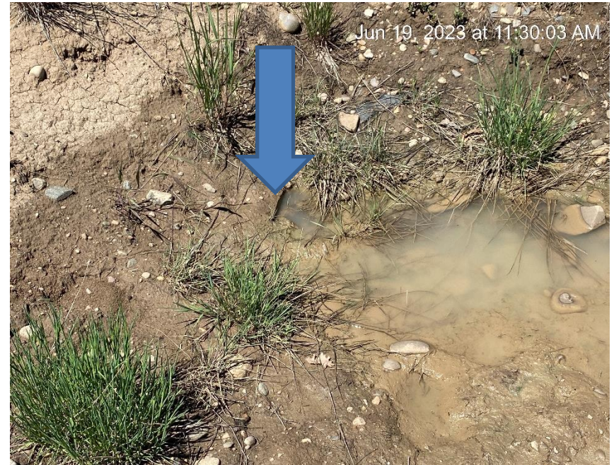
End of culvert plugged up
