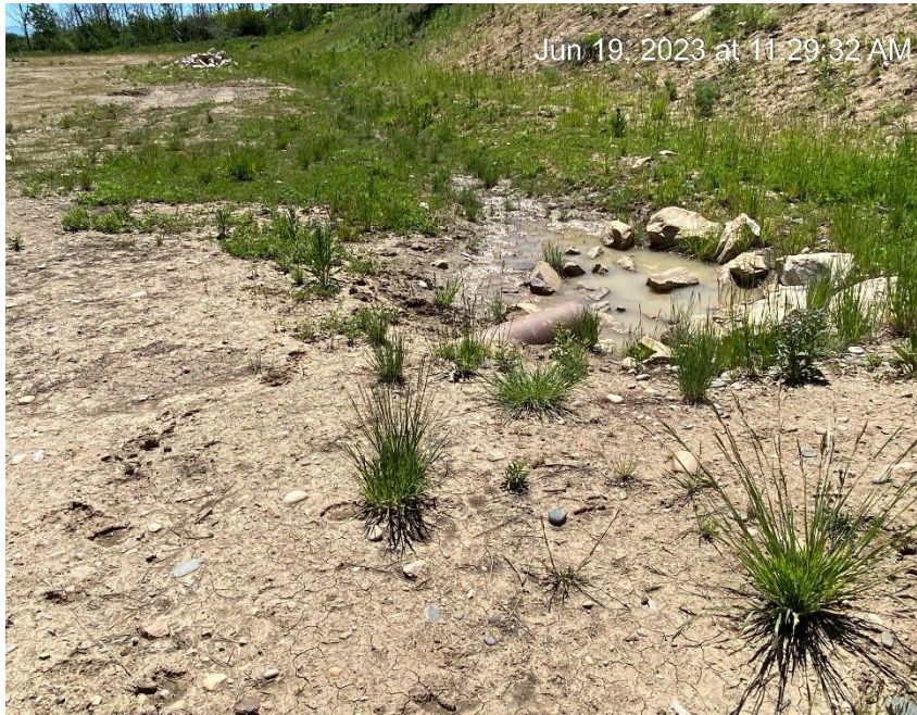
Culvert not maintained
