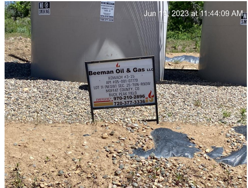
Tank battery sign missing required information
