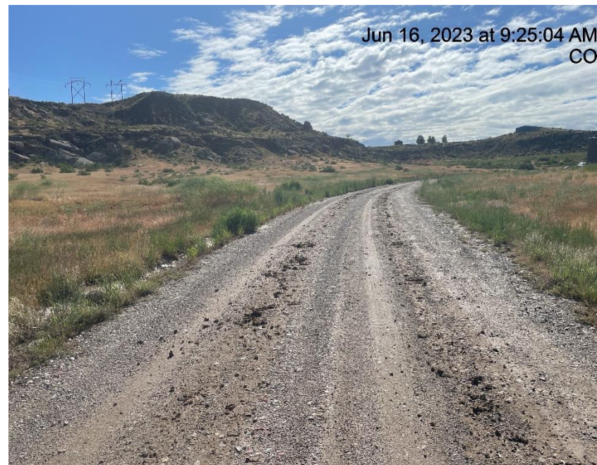
Photo # 713 Tracking on lease road/Insufficient tracking BMP's
