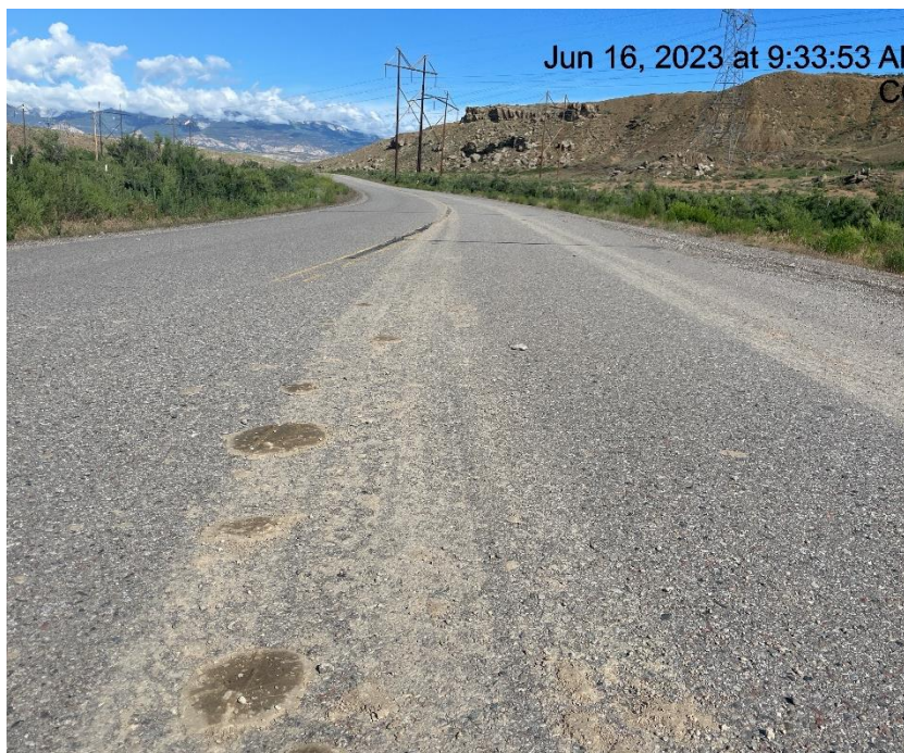
Photo # 726 Tracking on Mamm Creek Road/Insufficient tracking BMP's
