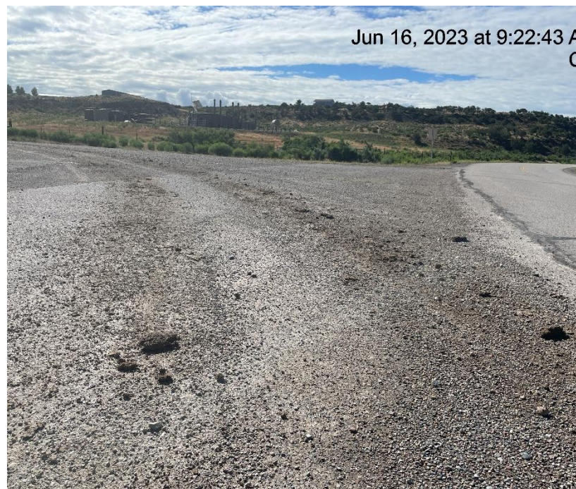
Photo # 704 Tracking from lease road onto Mamm Creek Road/Insufficient tracking BMP's
