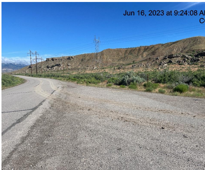
Photo # 711 Tracking from lease road onto Mamm Creek Road/Insufficient tracking BMP's
