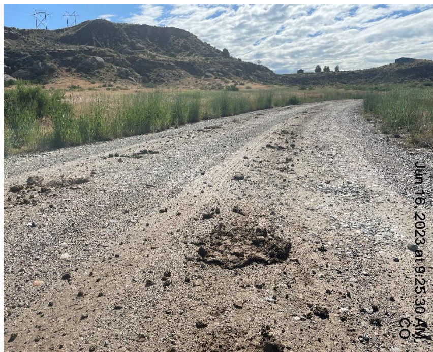
Photo # 716 Tracking on lease road/Insufficient tracking BMP's
