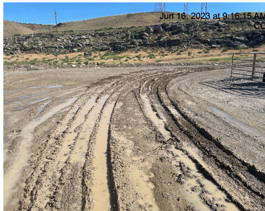
Photo # 678 Lack of stabilization/Compaction/ Insufficient tracking BMP's
