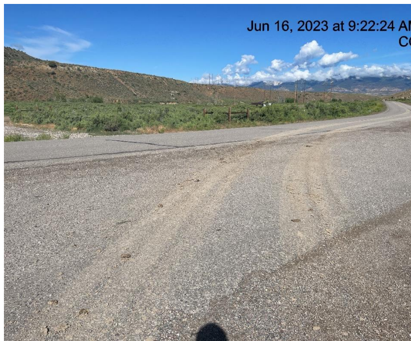
Photo # 703 Tracking from lease road onto Mamm Creek Road/Insufficient tracking BMP's
