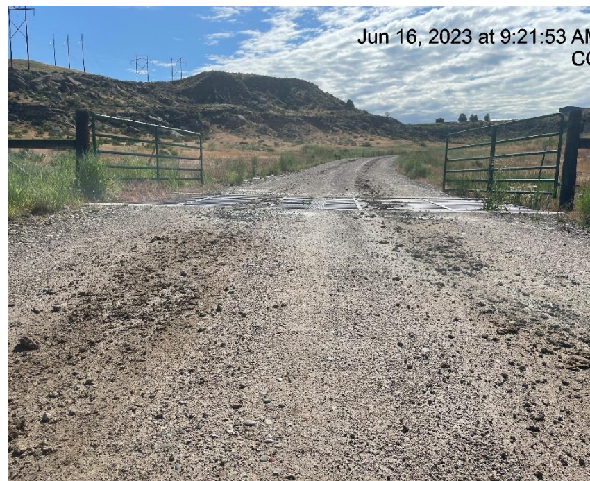
Photo # 700 Tracking on lease road/Insufficient tracking BMP's
