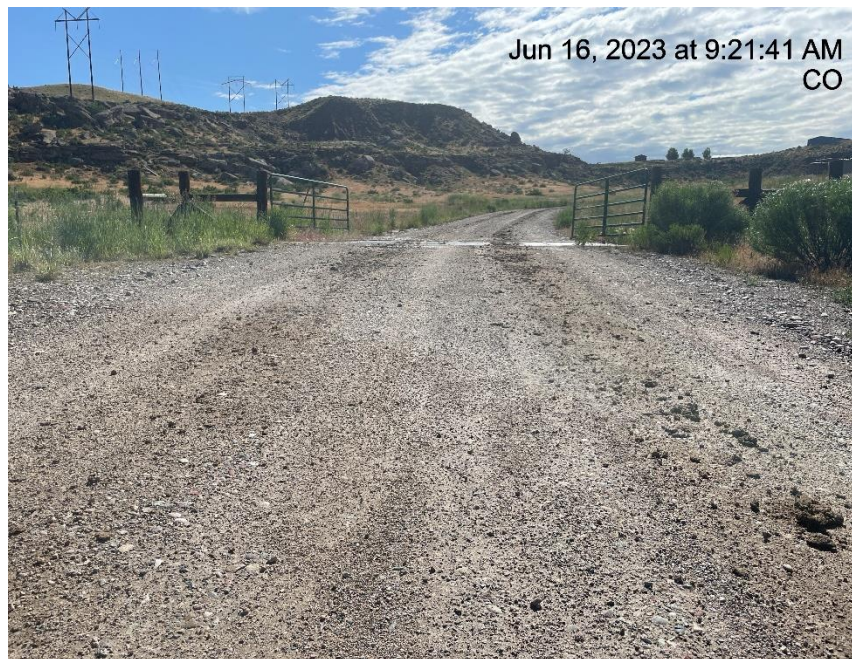
Photo # 701 Tracking on lease road/Insufficient tracking BMP's
