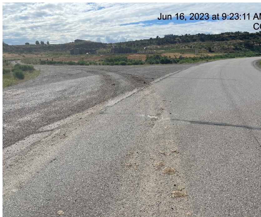
Photo # 707 Tracking from lease road onto Mamm Creek Road/Insufficient tracking BMP's
