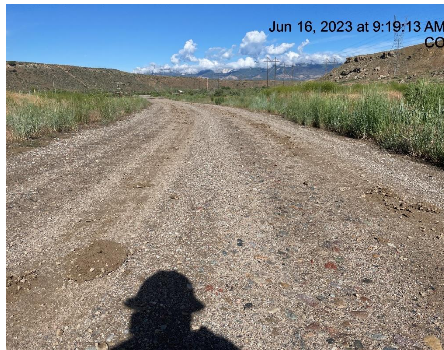
Photo # 692 Tracking on lease road/Insufficient tracking BMP's
