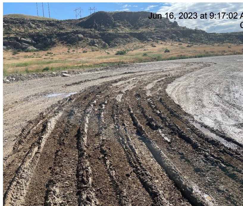
Photo # 682 Lack of stabilization/Compaction/ Insufficient tracking BMP's
