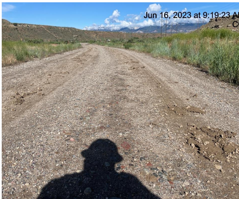
Photo # 693 Tracking on lease road/Insufficient tracking BMP's
