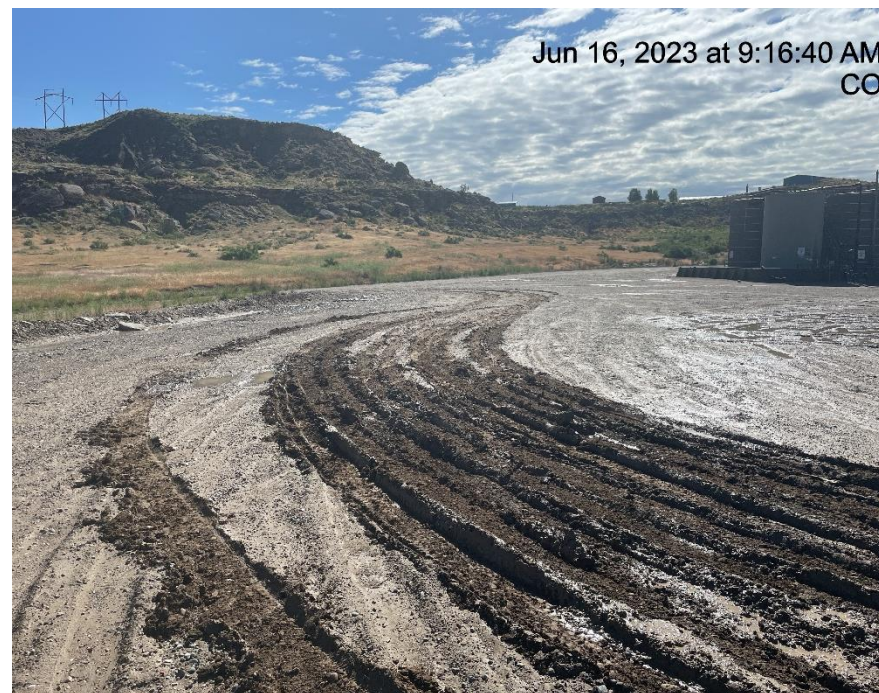
Photo # 680 Lack of stabilization/Compaction/ Insufficient tracking BMP's
