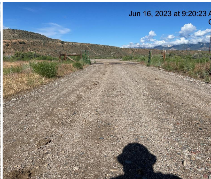
Photo # 697 Tracking on lease road/Insufficient tracking BMP's
