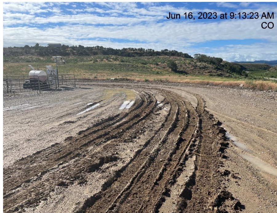
Photo # 675 Lack of stabilization/Compaction/ Insufficient tracking BMP's
