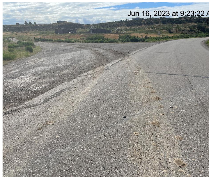
Photo # 708 Tracking from lease road onto Mamm Creek Road/Insufficient tracking BMP's
