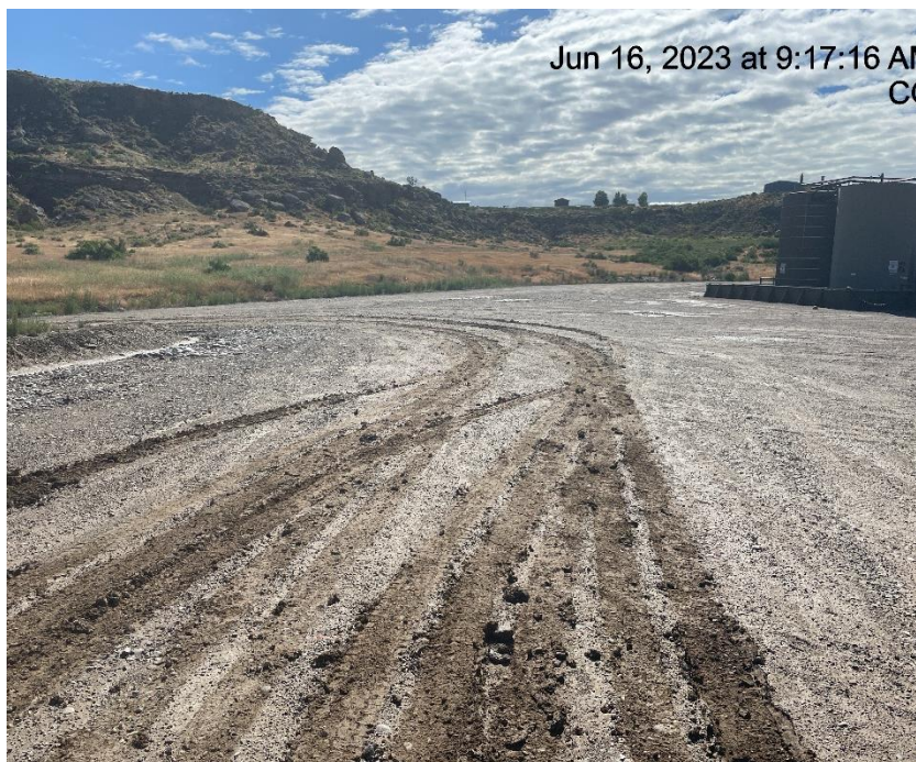
Photo # 683 Lack of stabilization/Compaction/ Insufficient tracking BMP's
