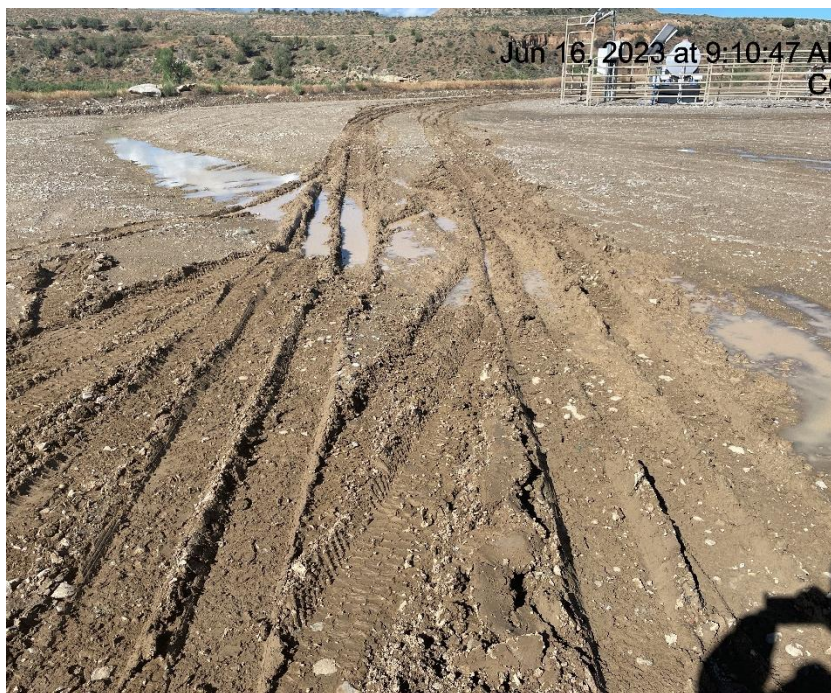
Photo # 664 Lack of stabilization/Compaction/ Insufficient tracking BMP's
