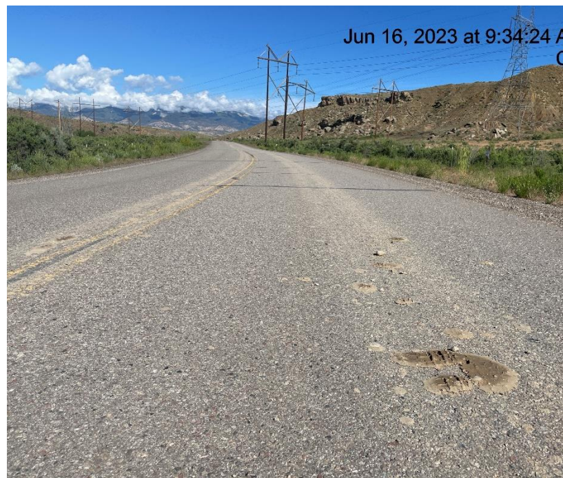
Photo # 729 Tracking on Mamm Creek Road/Insufficient tracking BMP's
