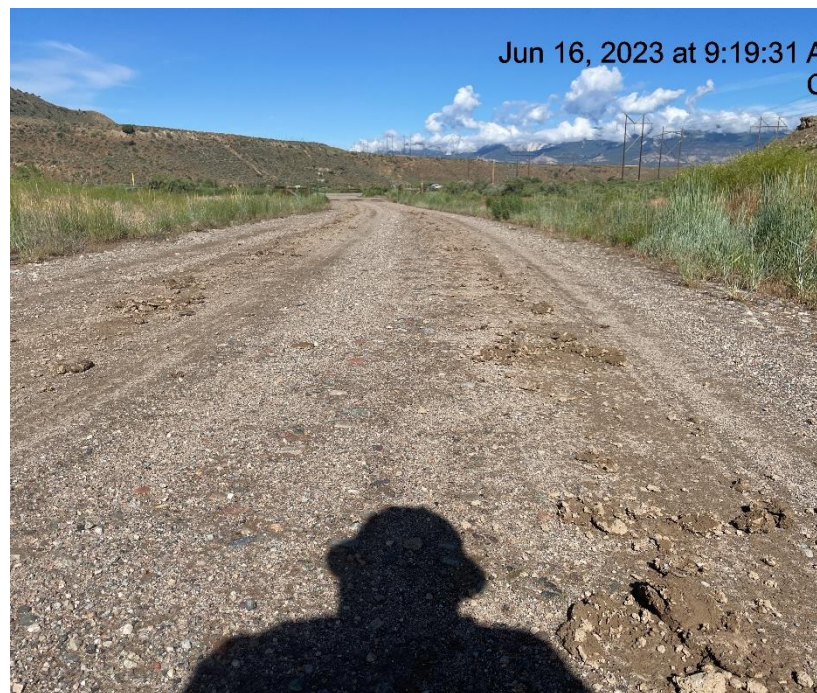
Photo # 694 Tracking on lease road/Insufficient tracking BMP's
