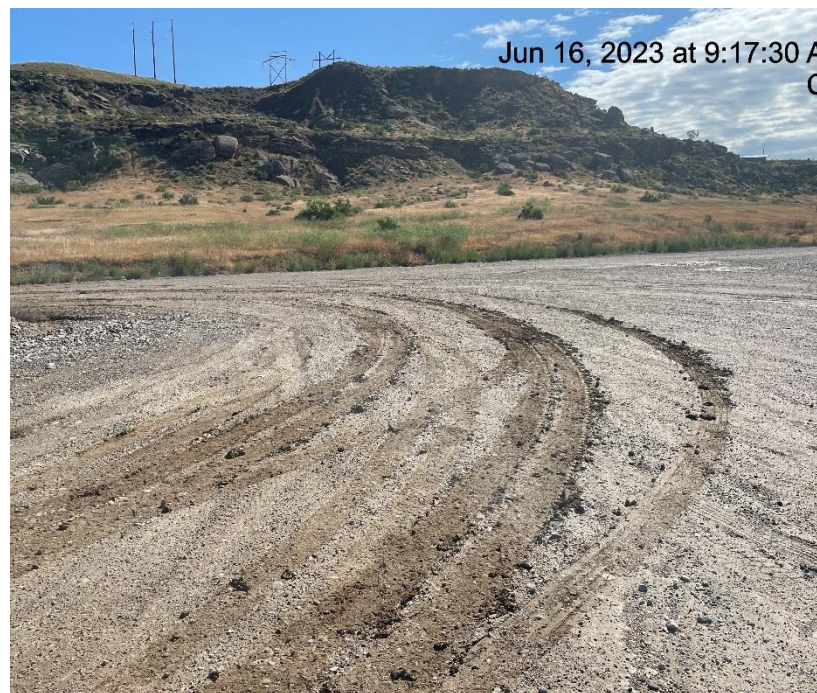
Photo # 684 Lack of stabilization/Compaction/ Insufficient tracking BMP's/Tracking from location onto lease road
