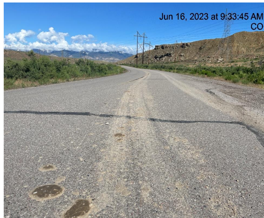
Photo # 725 Tracking on Mamm Creek Road/Insufficient tracking BMP's
