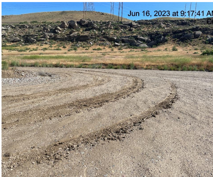
Photo # 685 Lack of stabilization/Compaction/ Insufficient tracking BMP's/Tracking from location onto lease road
