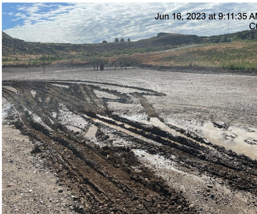
Photo # 666 Lack of stabilization/Compaction/ Insufficient tracking BMP's
