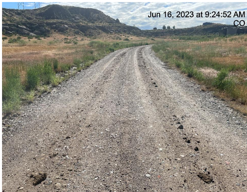
Photo # 712 Tracking on lease road/Insufficient tracking BMP's
