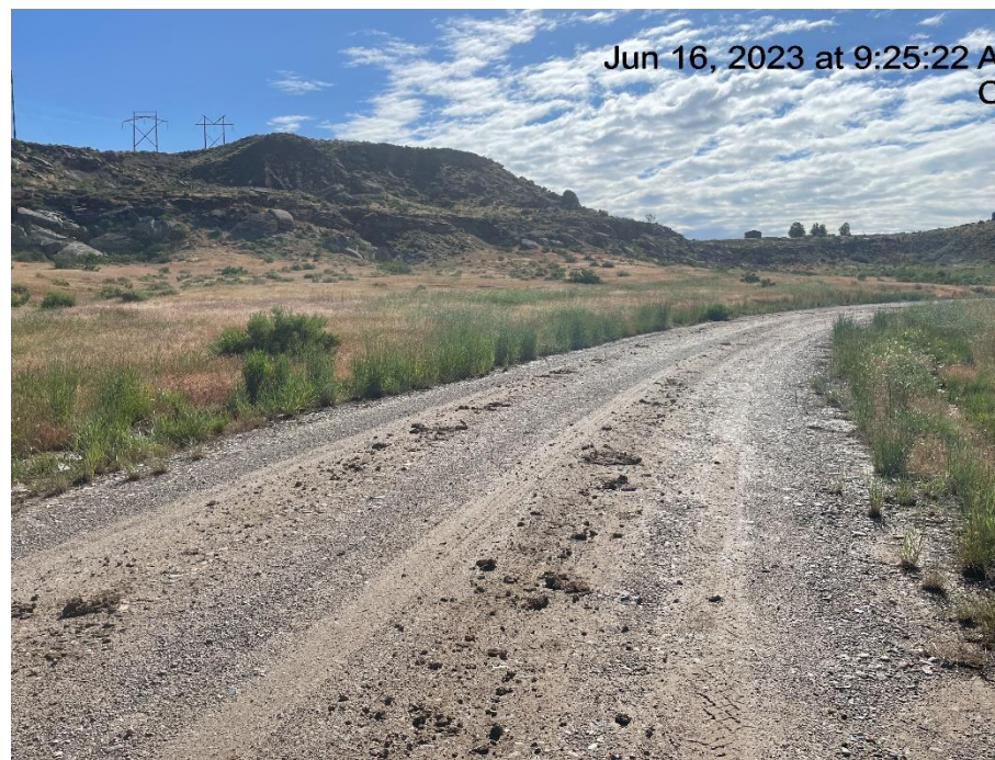
Photo # 715 Tracking on lease road/Insufficient tracking BMP's
