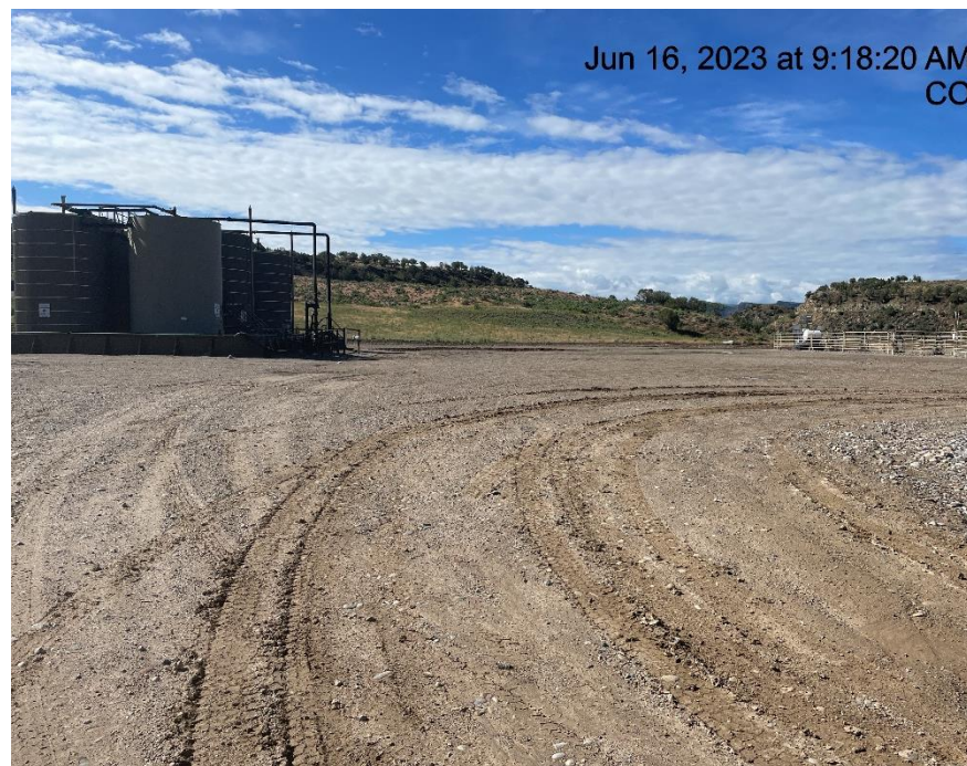
Photo # 688 Lack of stabilization/Compaction/ Insufficient tracking BMP's/Tracking from location onto lease road
