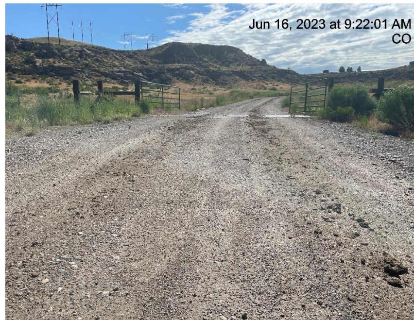
Photo # 702 Tracking on lease road/Insufficient tracking BMP's
