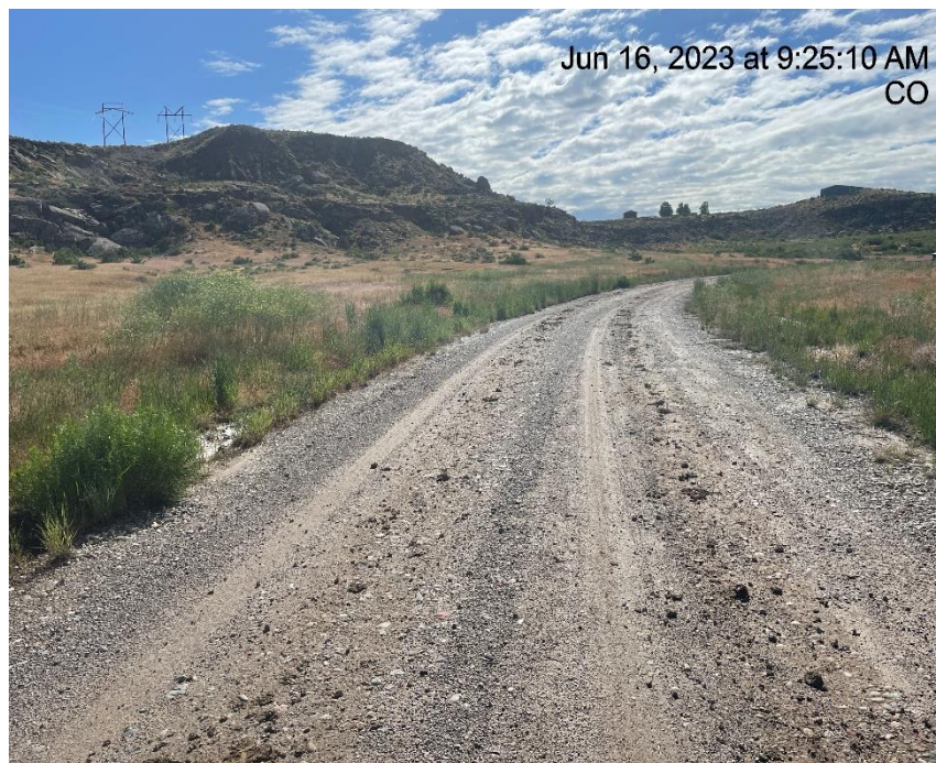
Photo # 714 Tracking on lease road/Insufficient tracking BMP's
