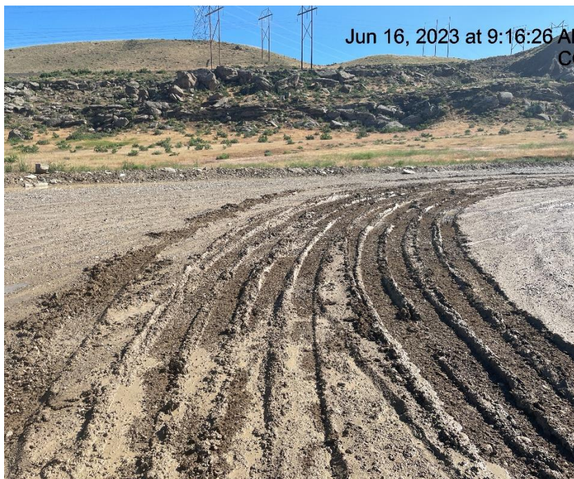
Photo # 679 Lack of stabilization/Compaction/ Insufficient tracking BMP's
