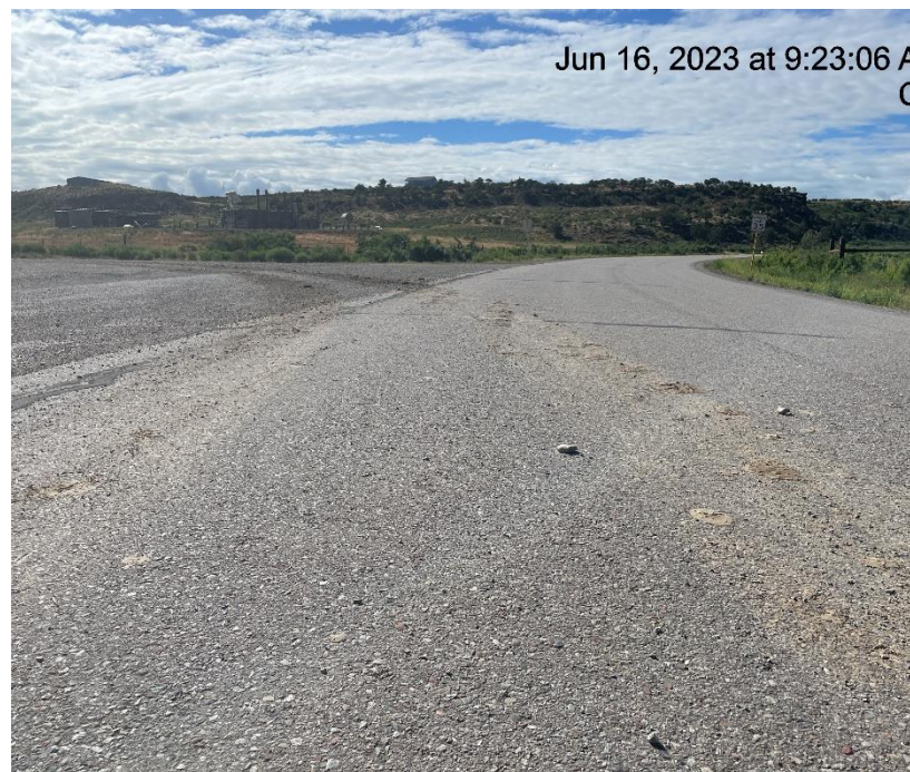
Photo # 706 Tracking from lease road onto Mamm Creek Road/Insufficient tracking BMP's
