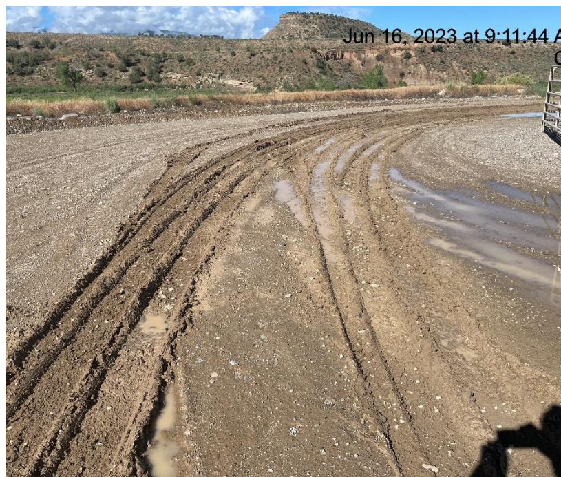
Photo # 667 Lack of stabilization/Compaction/ Insufficient tracking BMP's
