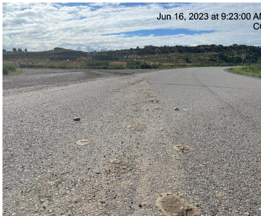
Photo # 705 Tracking from lease road onto Mamm Creek Road/Insufficient tracking BMP's
