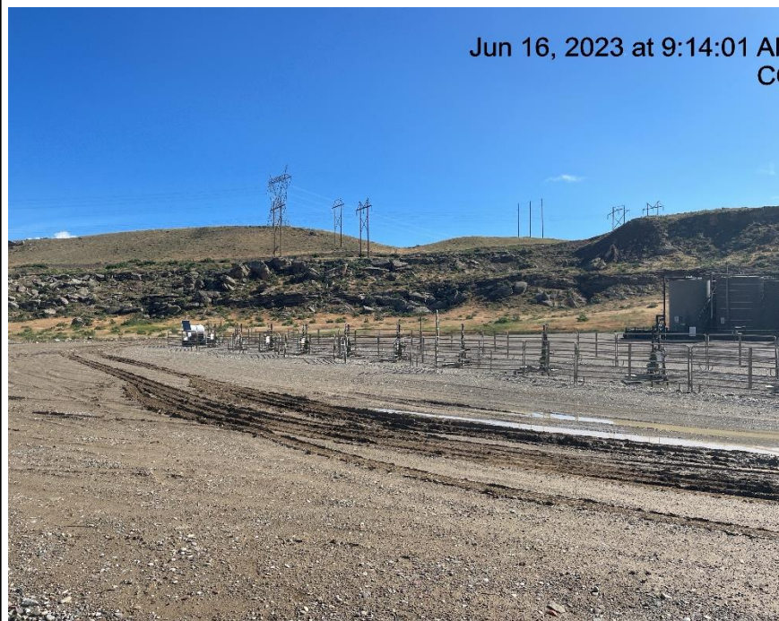
Photo # 676 Lack of stabilization/Compaction/ Insufficient tracking BMP's
