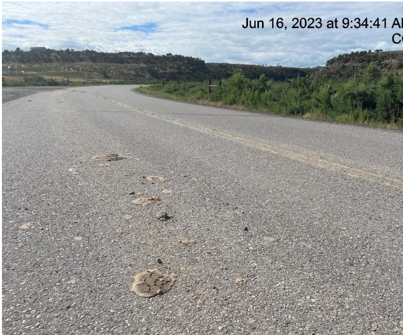
Photo # 730 Tracking on Mamm Creek Road/Insufficient tracking BMP's
