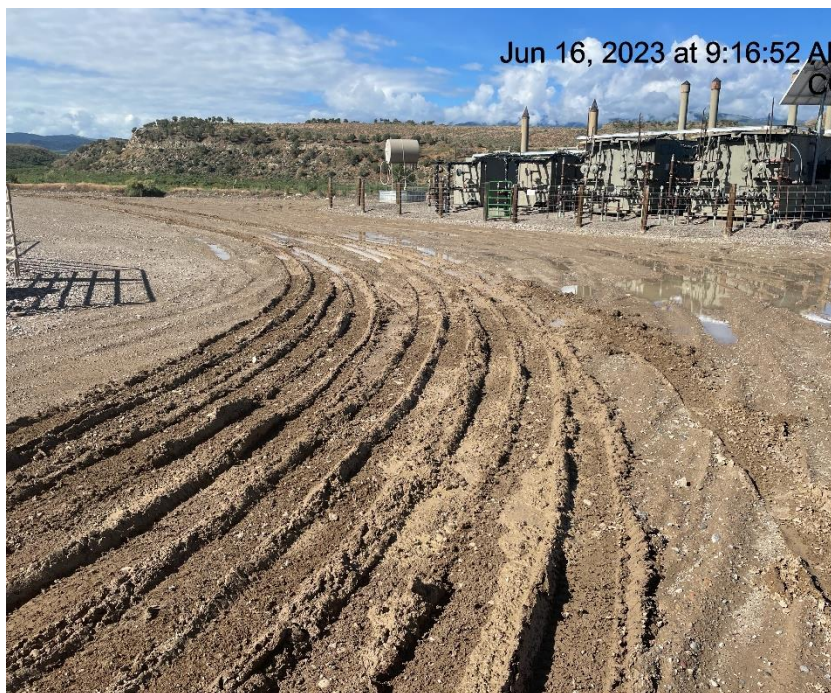
Photo # 681 Lack of stabilization/Compaction/ Insufficient tracking BMP's
