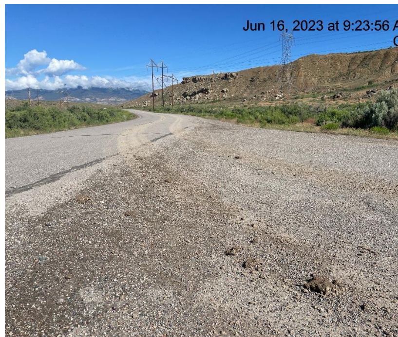
Photo # 710 Tracking from lease road onto Mamm Creek Road/Insufficient tracking BMP's
