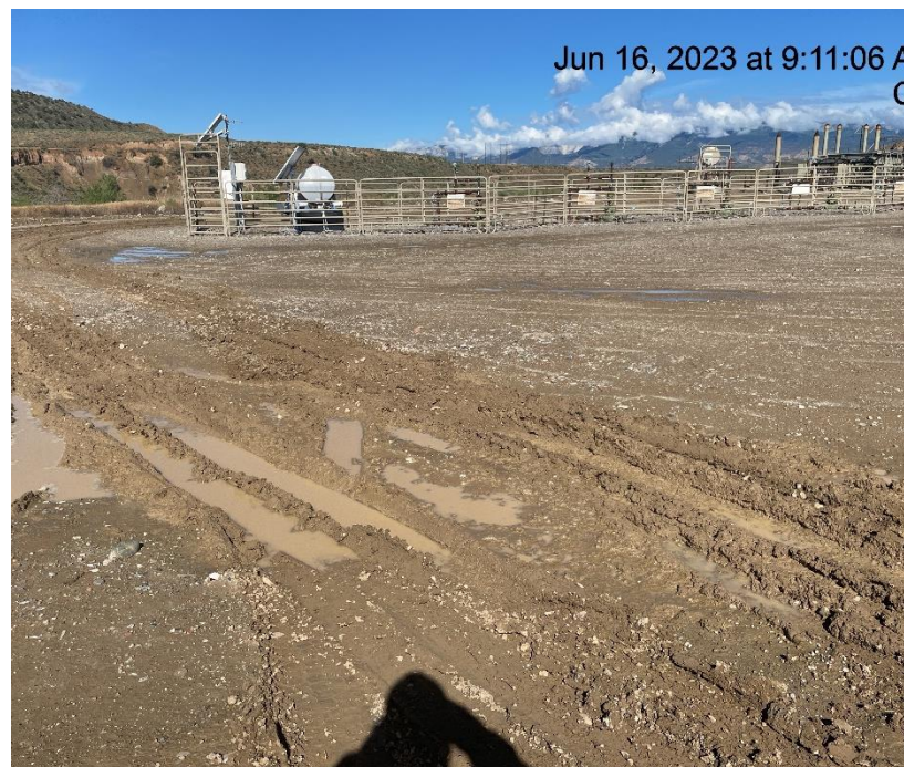
Photo # 665 Lack of stabilization/Compaction/ Insufficient tracking BMP's
