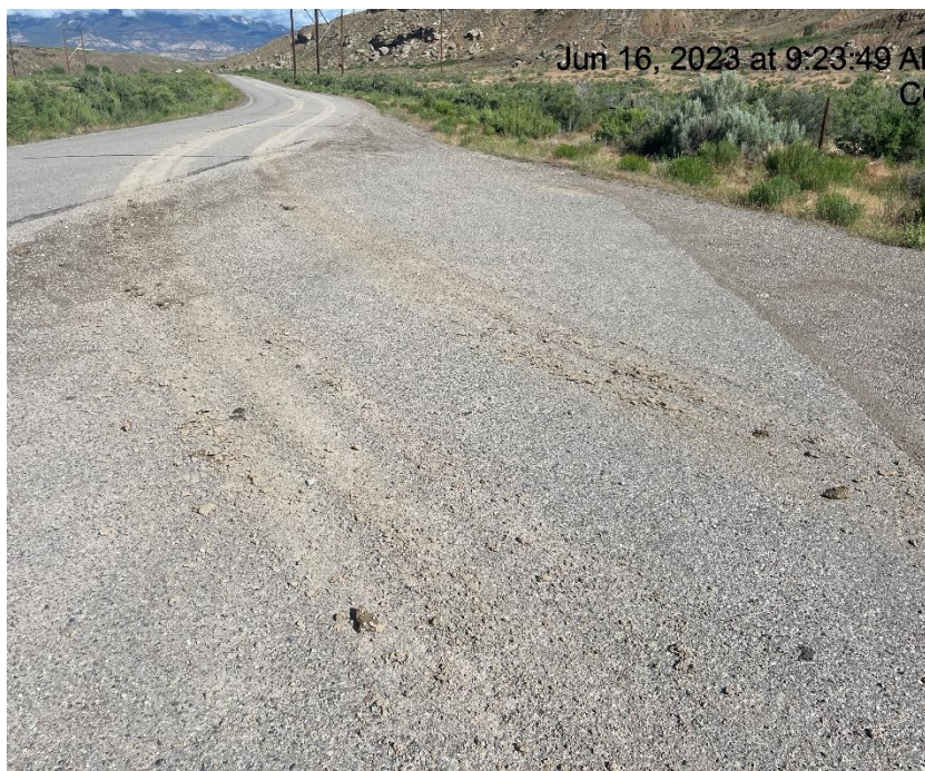
Photo # 709 Tracking from lease road onto Mamm Creek Road/Insufficient tracking BMP's
