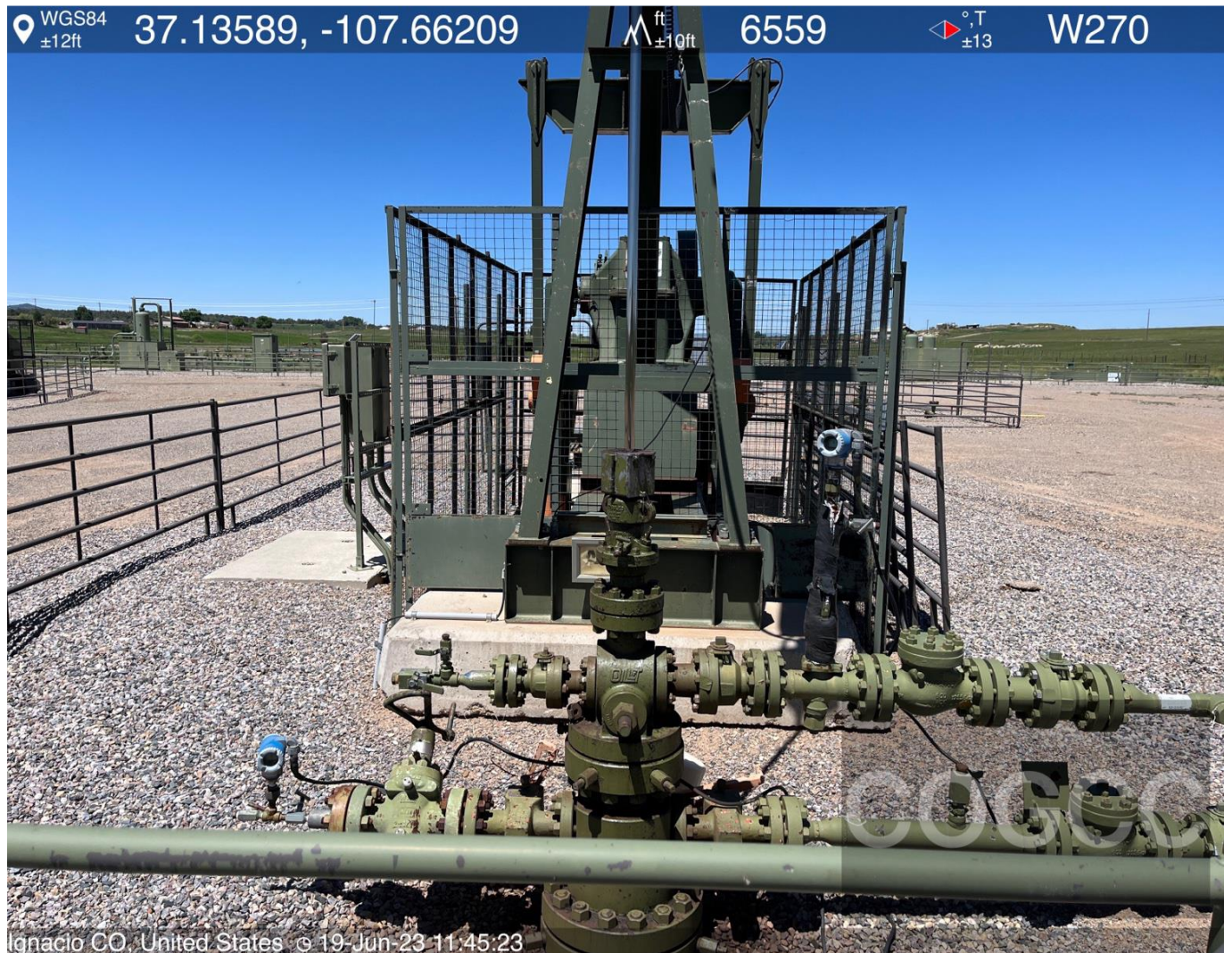
Photo #3 View of the A2 wellhead assembly.
