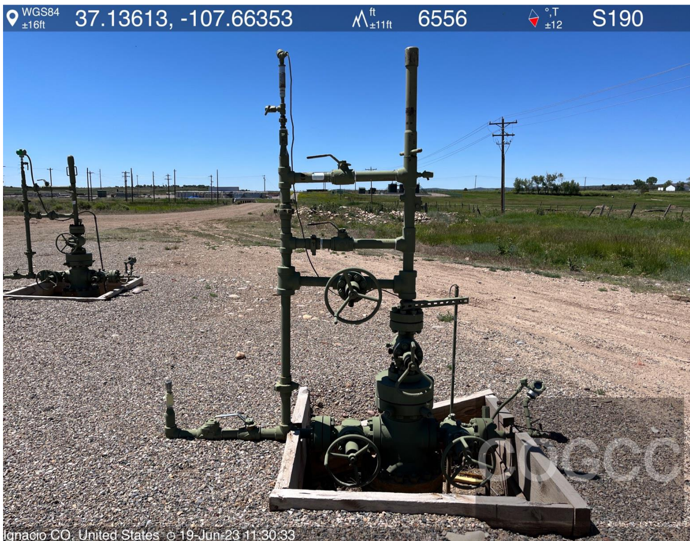
Photo #2 View of a wellhead assembly.
