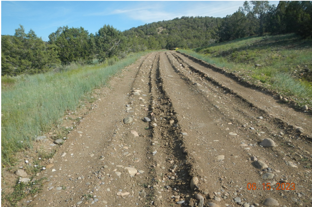
Photo 2. Facing northwest along the access road. There is vehicle rutting and tracking along the road that needs to be repaired and stabilized. Previous corrective action was not completed.
