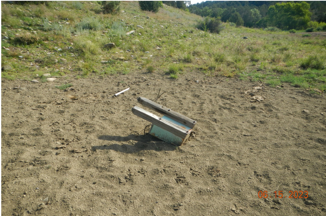
Photo 7. There is an electric utility that has fallen over at the northside of the location hand needs to be removed or repaired.
