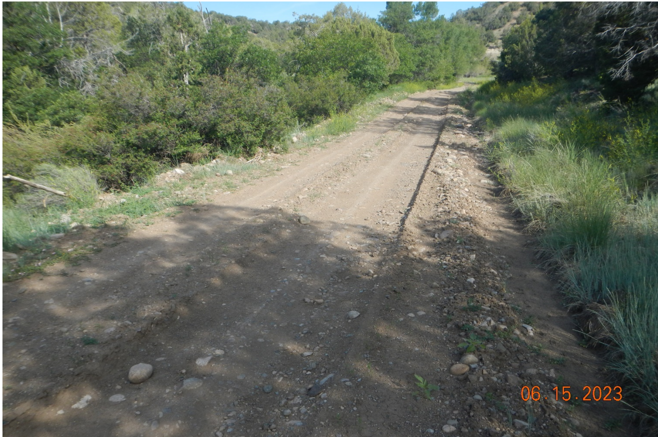
Photo 3. Facing northwest along the access road. This area had previously washed out and was repaired however, stormwater is directed down this area and there are no BMP's to divert off the road e.g. culvert water bar ect.
