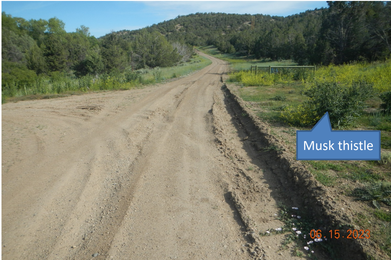
Photo 1. Facing northwest along the access road. There is vehicle rutting and tracking along the road that needs to be repaired and stabilized. There are also noxious weeds along the roadside that need to be controlled.
