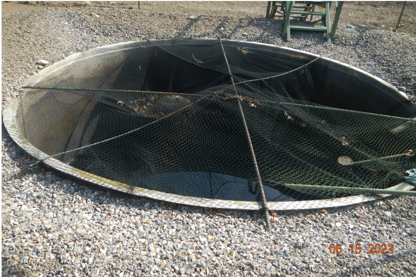
Photo 5. The netting on the buried tank is not maintained to prevent wildlife entry.
