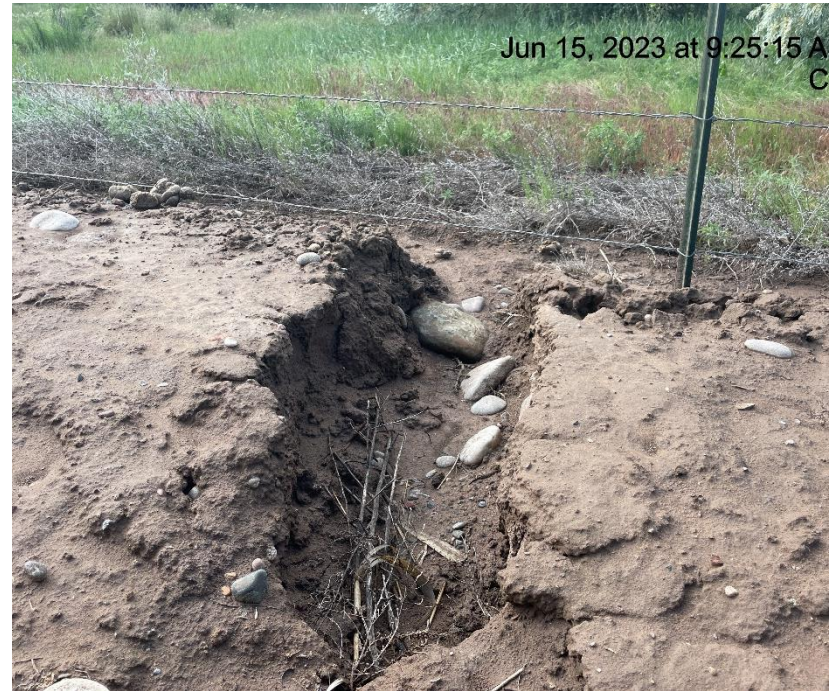
Photo # 503 Berm needs maintenance - erosion through berm & transport of sediment off location
