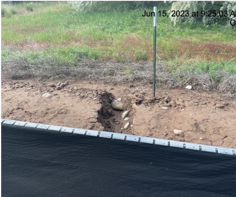
Photo # 502 Berm needs maintenance - erosion through berm & transport of sediment off location
