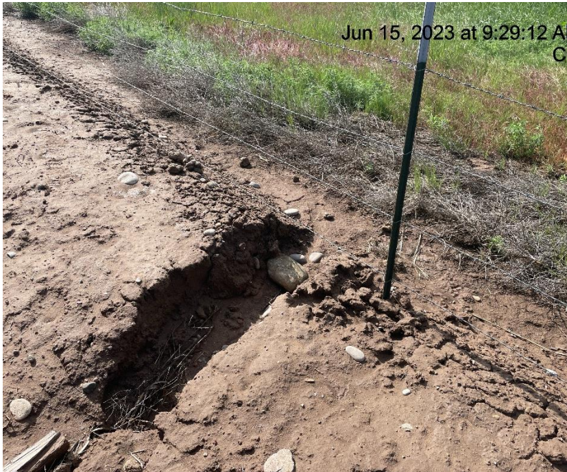
Photo # 510 Berm needs maintenance - erosion through berm & transport of sediment off location
