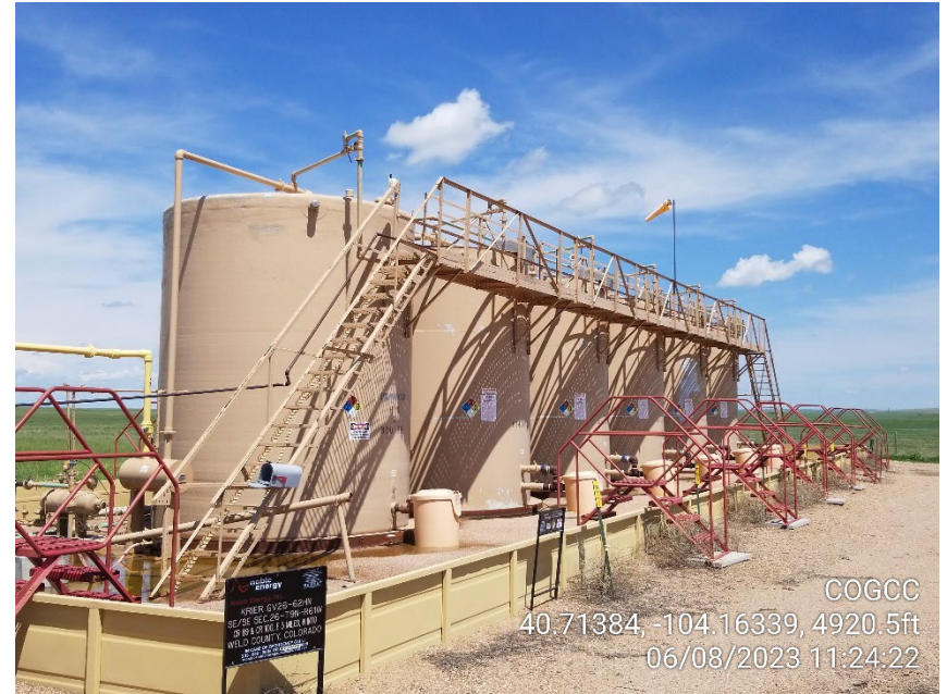
Photo 6 – Tank Battery
