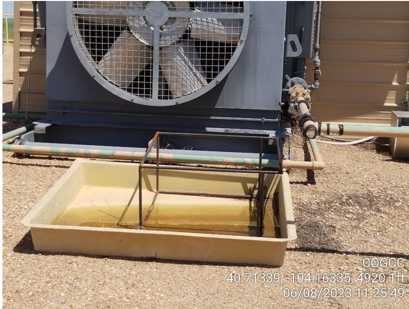
Photo 9 – Unused Stand and Secondary Containment
