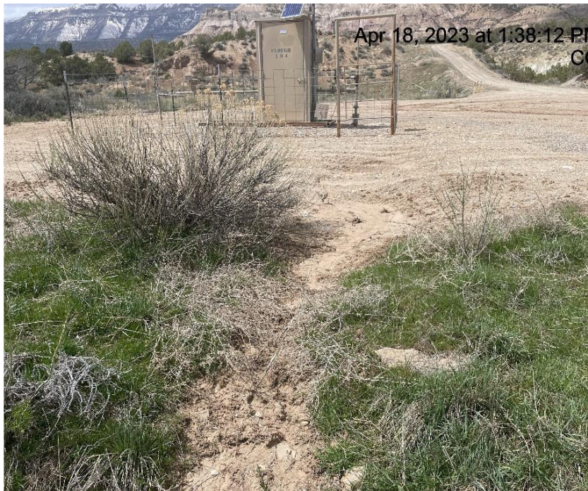
Photo # 5695 From Inspection 708900299 conducted on 04/18/2023 Erosion & transport of sediment off location
