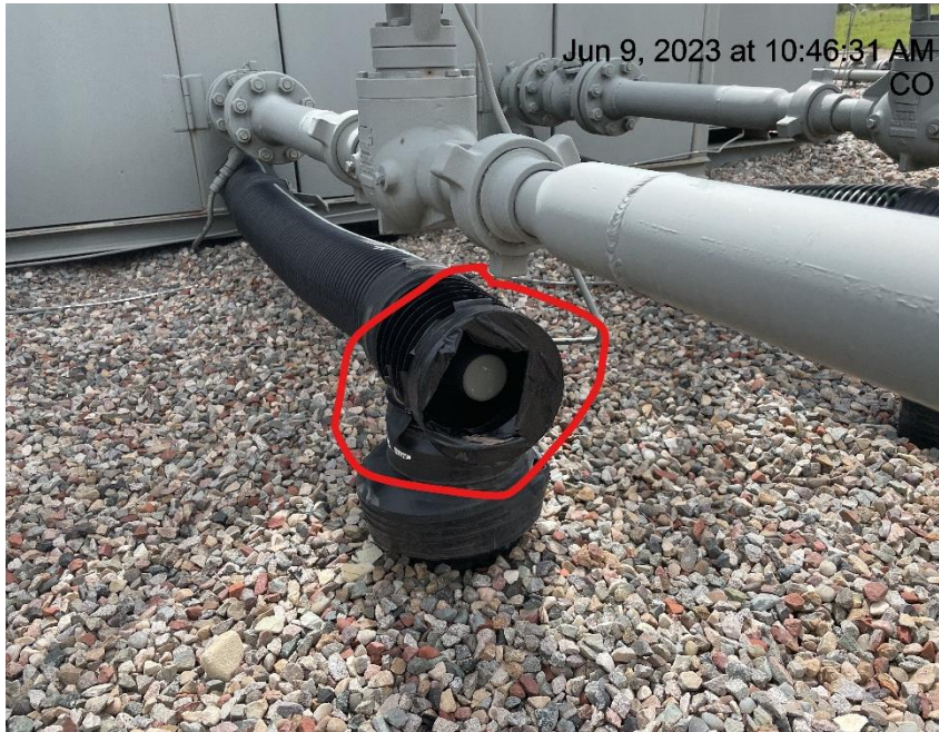
Photo # 9987 Flowline heating insulation open ended
