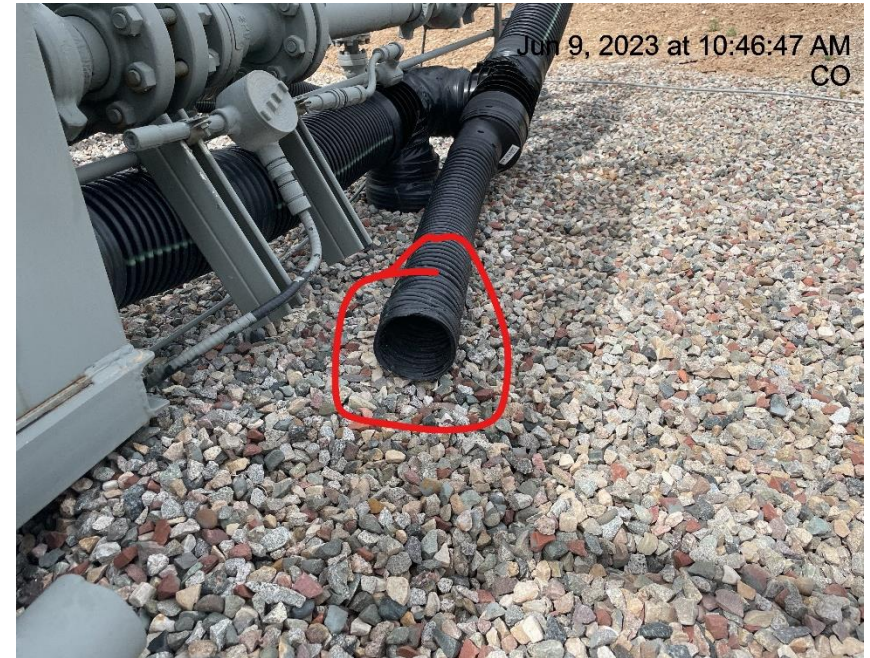
Photo # 9989 Flowline heating insulation open ended
