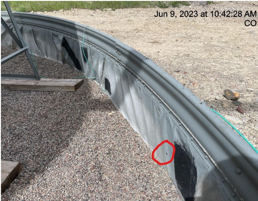
Photo # 9980 Containment liner needs maintenance
