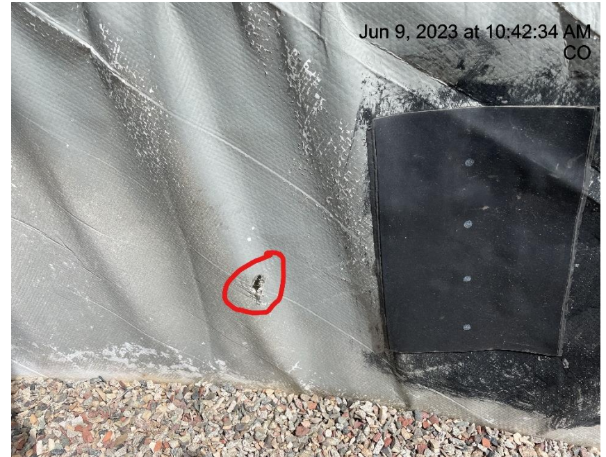
Photo # 9981 Containment liner needs maintenance
