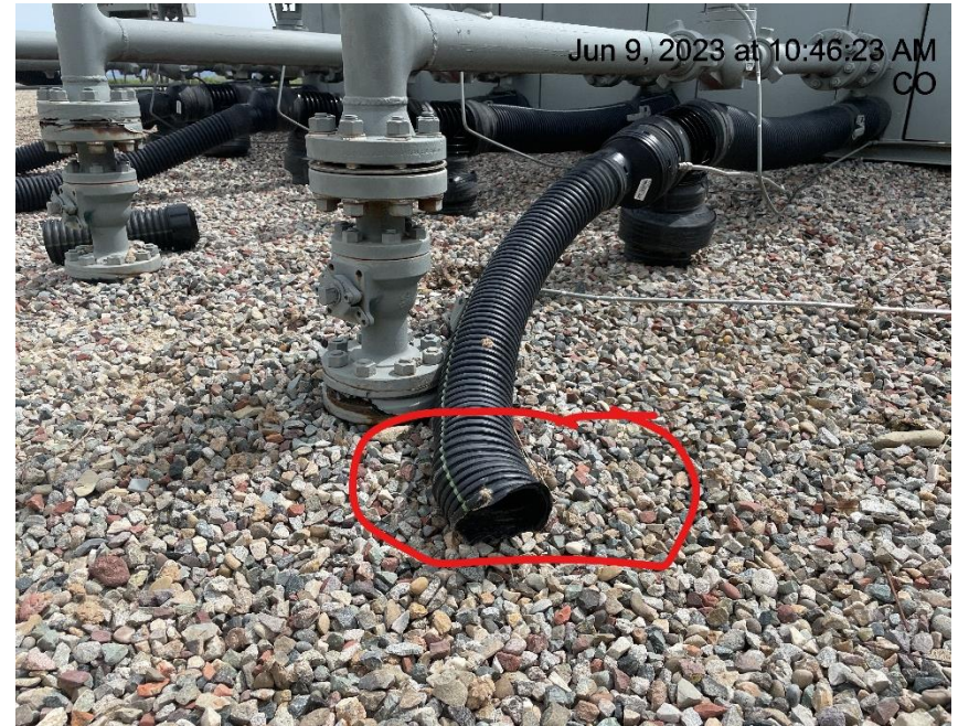
Photo # 9986 Flowline heating insulation open ended
