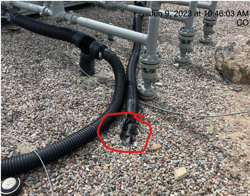
Photo # 9985 Flowline heating insulation open ended
