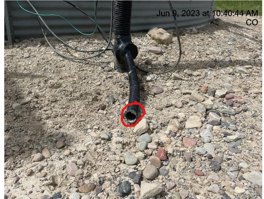
Photo # 9978 Flowline heating insulation open ended
