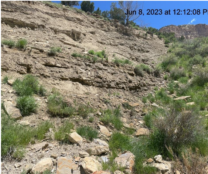
Photo # 9839 Lack of stabilization on cut slope
