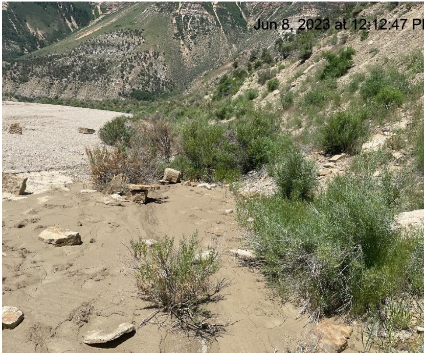
Photo # 9842 Transport of sediment onto location/ insufficient run on controls/BMP's
