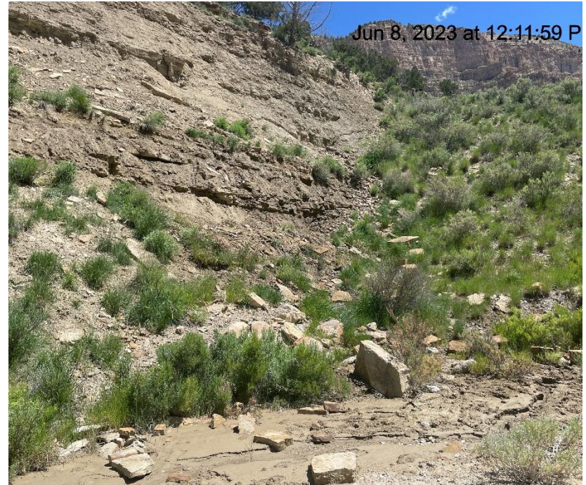
Photo # 9838 Lack of stabilization on cut slope
