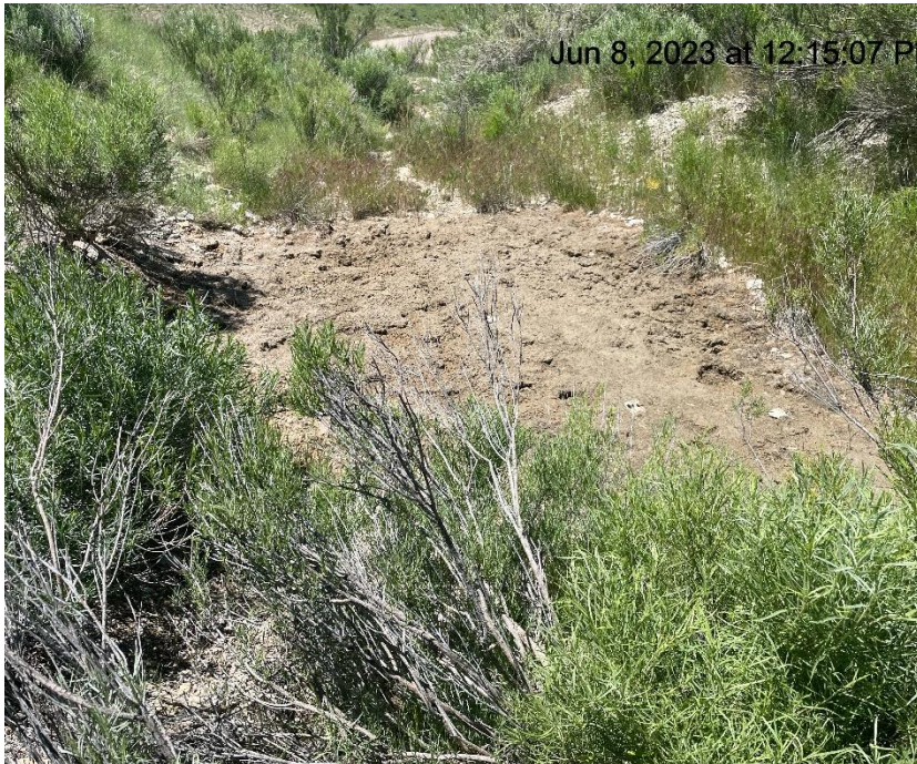
Photo # 9847 Sediment trap needs maintenance
