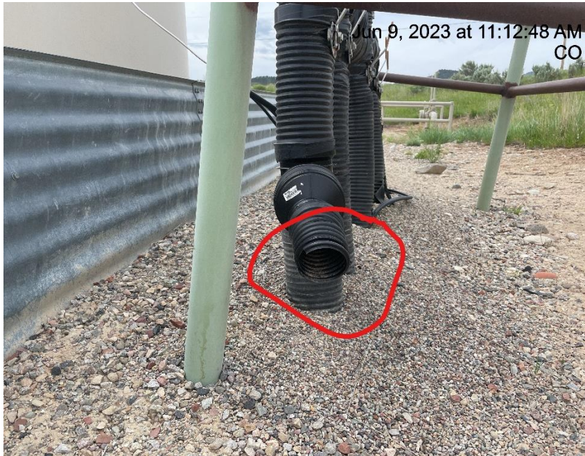
Photo # 16 Flowline heating insulation open ended
