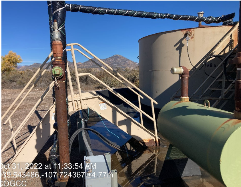
Disconnected lines to stored equipment from last inspections document # 700704665
