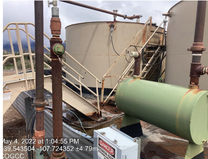
Disconnected lines to stored equipment from 2 inspections ago document # 700704160
