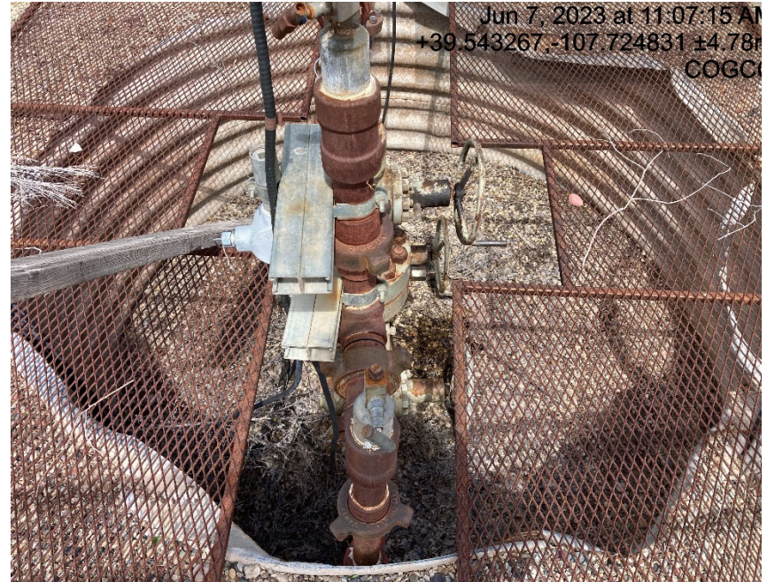
Open cellars and staining under valves
