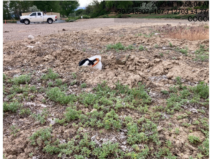
Recent inspection of interm reclamation driven on. Hard hat for reference of how deep tracks are.
