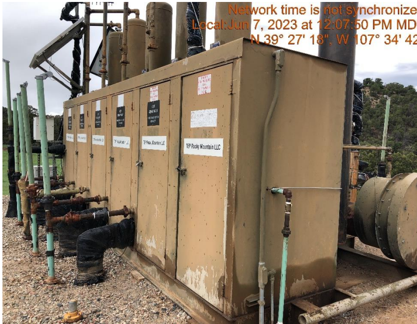
Photo #285 Meter calibration cards not conspicuously posted.
