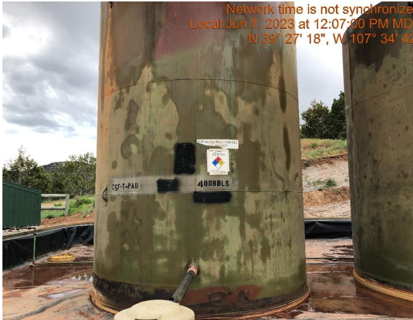
Photo #282 Tank label weathered and not legible.
