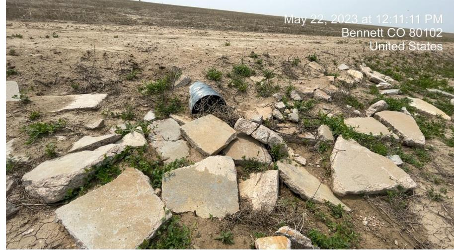
**Photo 4. Photo of concrete used as riprap on access road culvert.**
