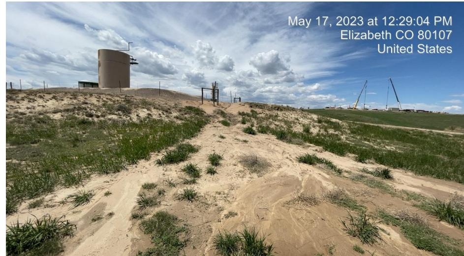
**Photo 5. Photo taken of access road ditch, erosion, No BMP's present to slow or filter run off.**
