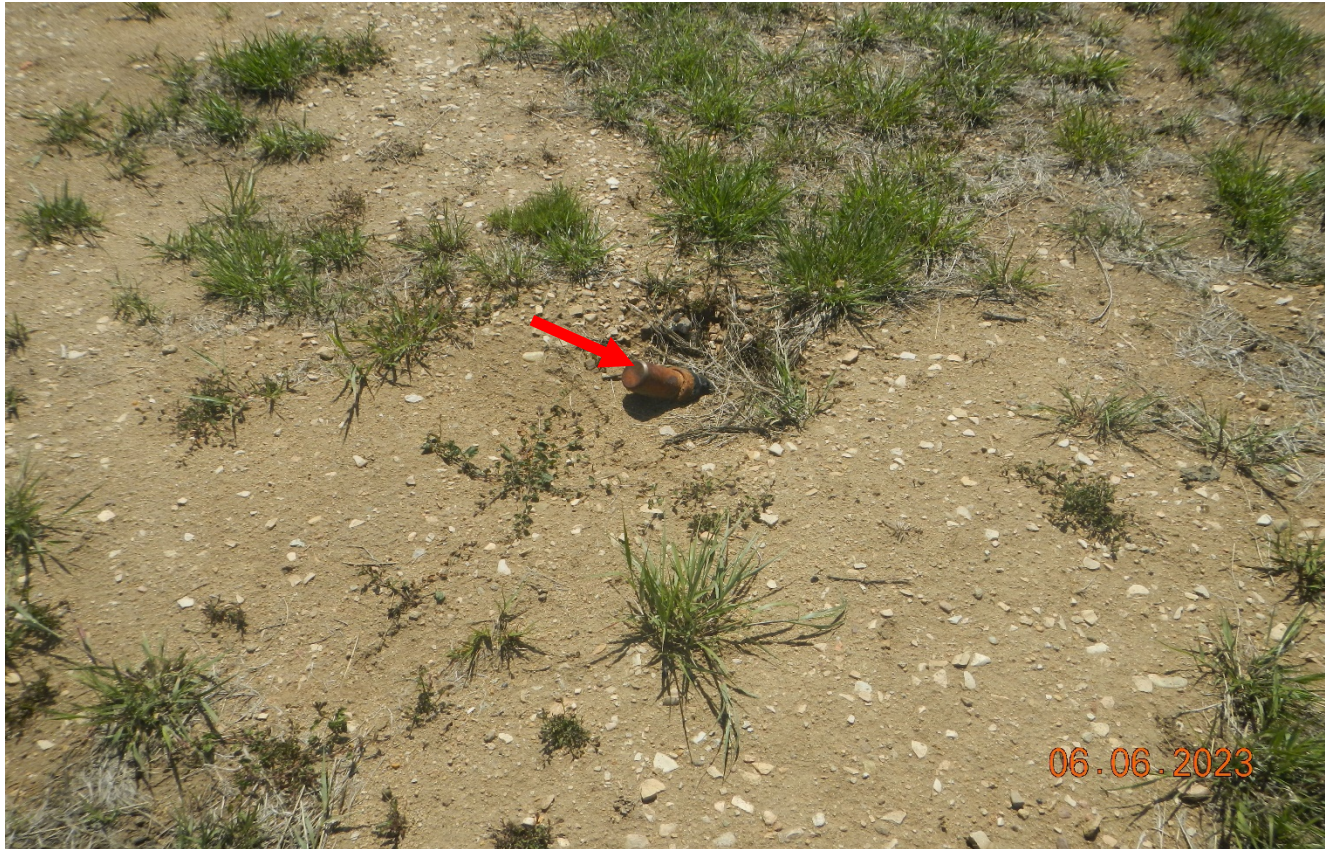
Photo 5. There is a pipe riser that remains at the surface of the location that needs to be properly abandoned.
