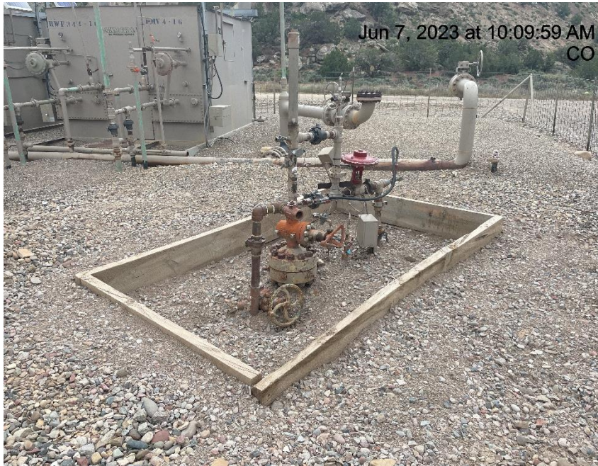
Photo # 9710 Wellhead cellar lacks wildlife egress
