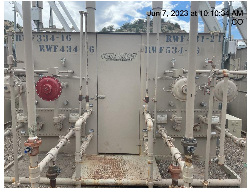
Photo # 9713 Meter calibration info not conspicuously posted
