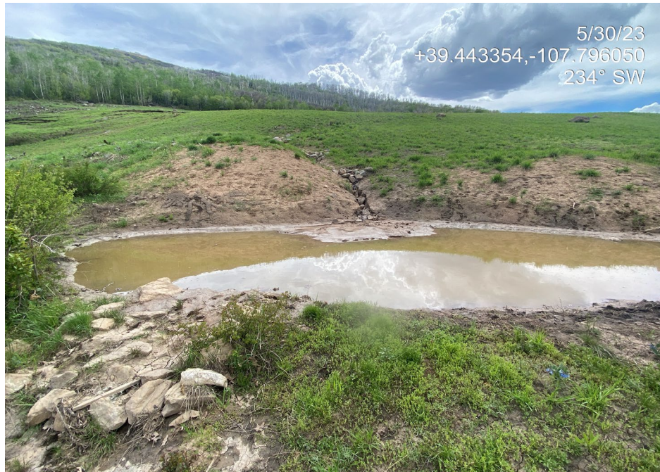
Photo 8. Photos show sediment transport and offsite degradation from the sediment trap at the southeast.
