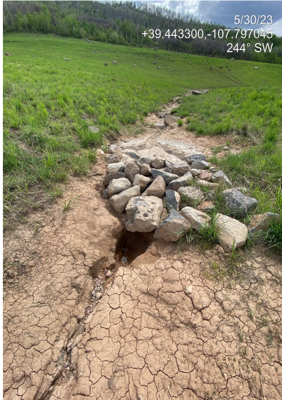
Photo 7. Photos show a stormwater ditch to the south of the working pad. Stormwater is eroding the ditch and cutting beneath rock check dams degrading the BMPs and resulting in increased sediment loads.
