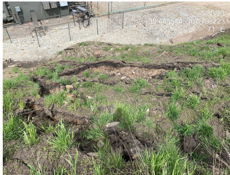
Photo 4. Photos show slumping in the interim area directly to west of the separators.
