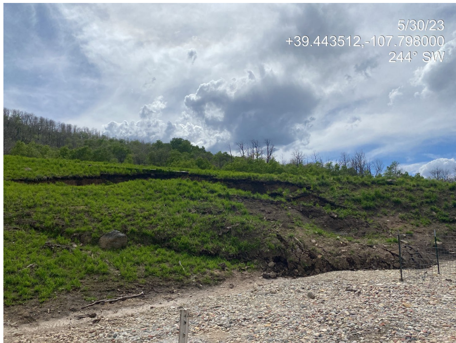
Photo 4. Photos show slumping in the interim area directly to west of the separators.
