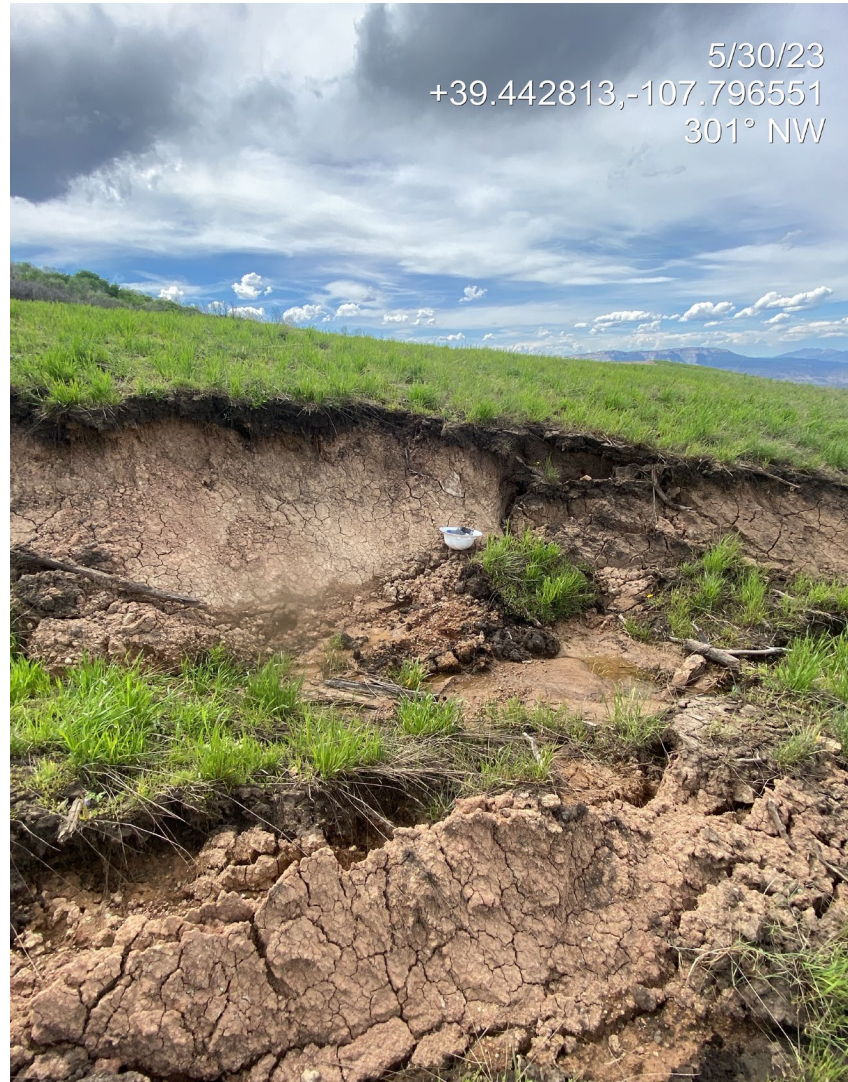
Photo 6. Photo shows slumping in the southern interim area.
