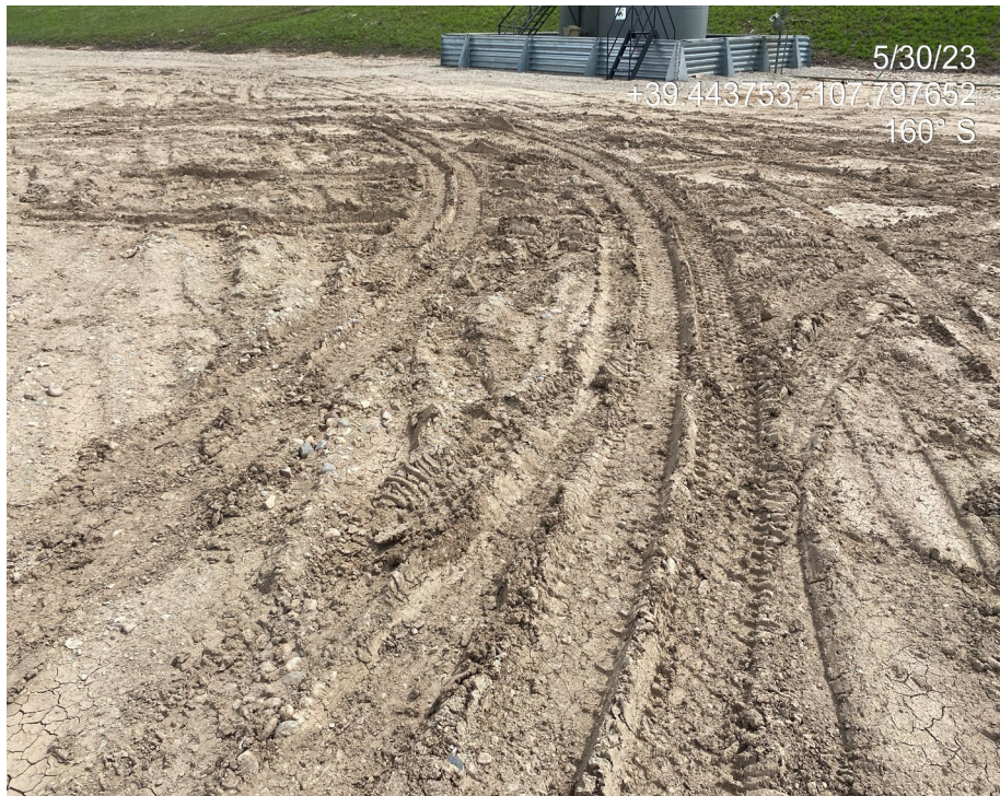
Photo 3. Photos show lack of stabilization of the working pad surface.
