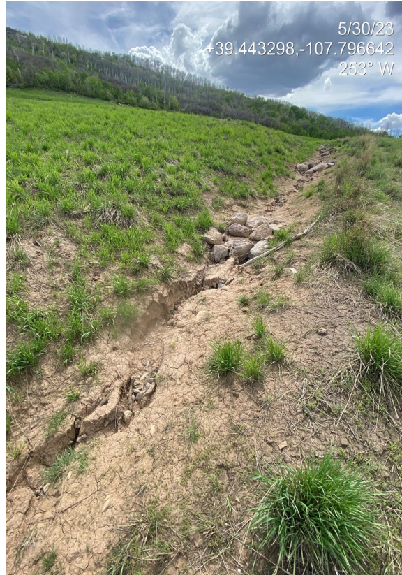
Photo 7. Photos show a stormwater ditch to the south of the working pad. Stormwater is eroding the ditch and cutting beneath rock check dams degrading the BMPs and resulting in increased sediment loads.
