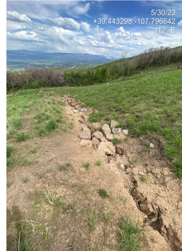
Photo 7. Photos show a stormwater ditch to the south of the working pad. Stormwater is eroding the ditch and cutting beneath rock check dams degrading the BMPs and resulting in increased sediment loads.
