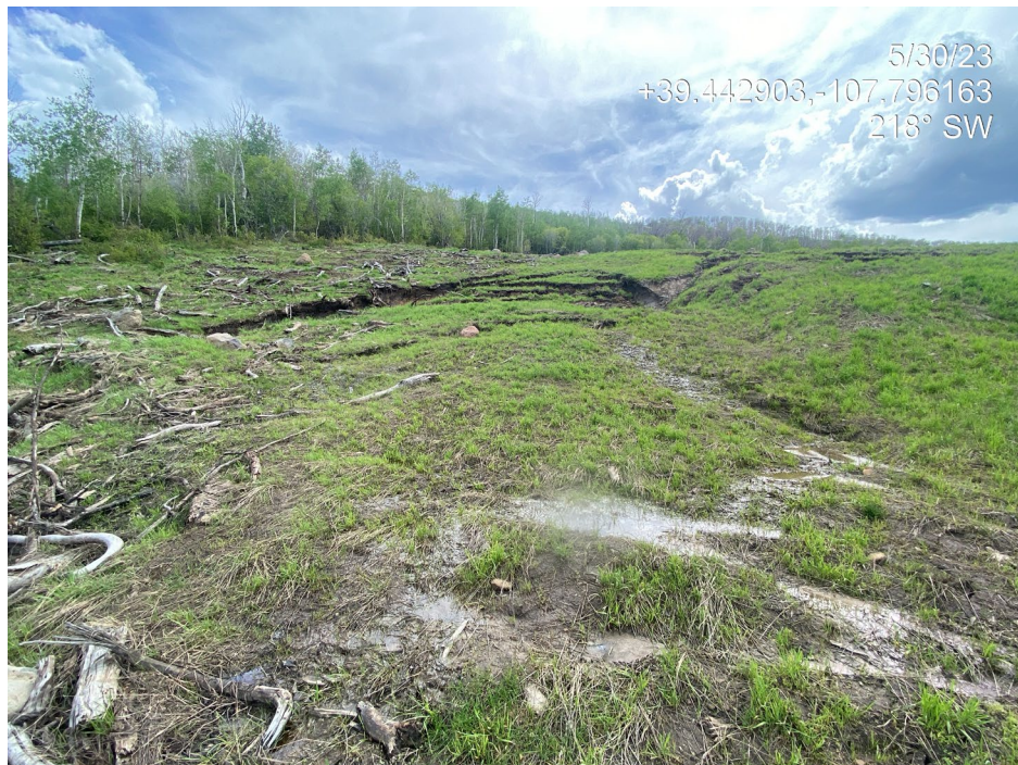
Photo 5. Photos show slumping in the southern interim area.
