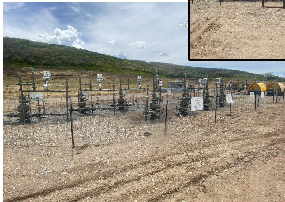
Photo 9. Photos show production areas and the lack of stabilization of the working pad surface.
