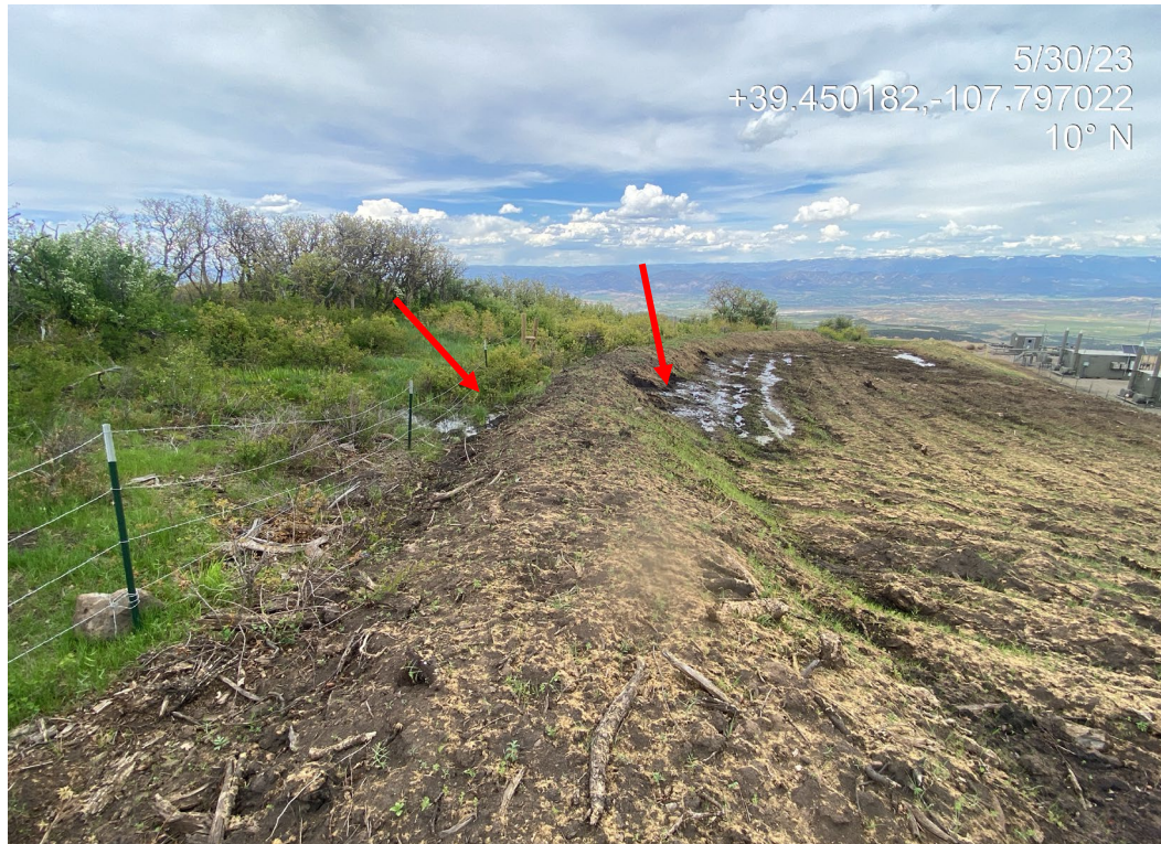
Photo 5. Photos show an area to the northwest where stormwater concentrates and is breaking through the perimeter berm causing degradation to the berm and rill erosion in the northern interim areas.
