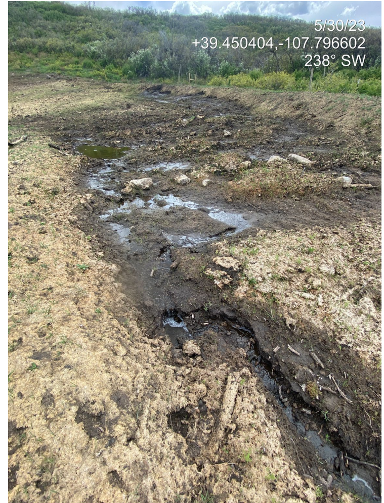
Photo 5. Photos show an area to the northwest where stormwater concentrates and is breaking through the perimeter berm causing degradation to the berm and rill erosion in the northern interim areas.
