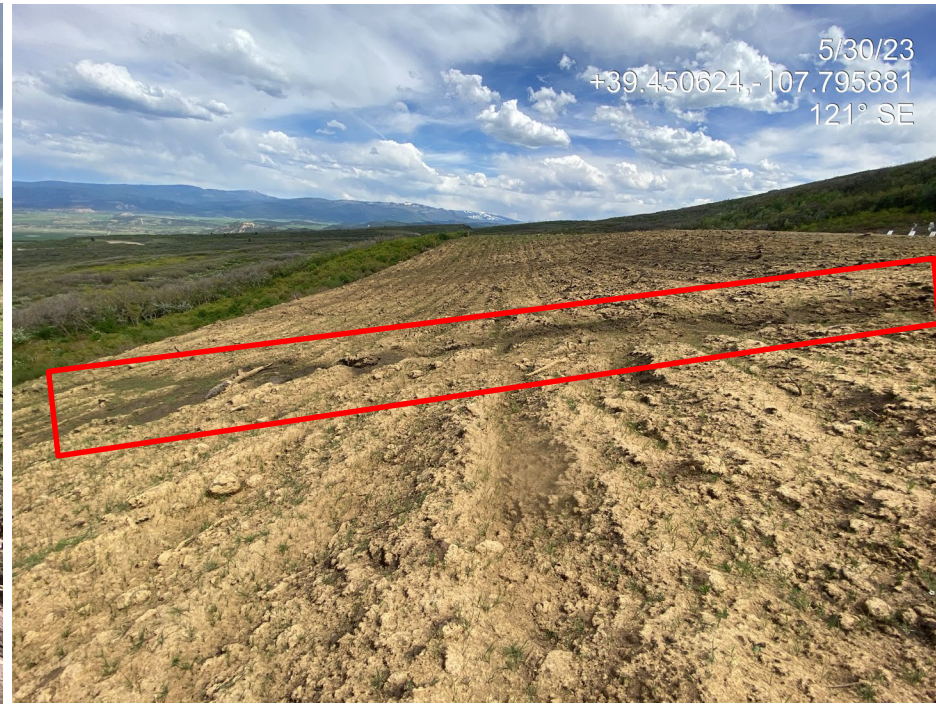
Photo 4. Photos show the southern (left) and eastern (right) interim areas. Areas of gully erosion are outlined.
