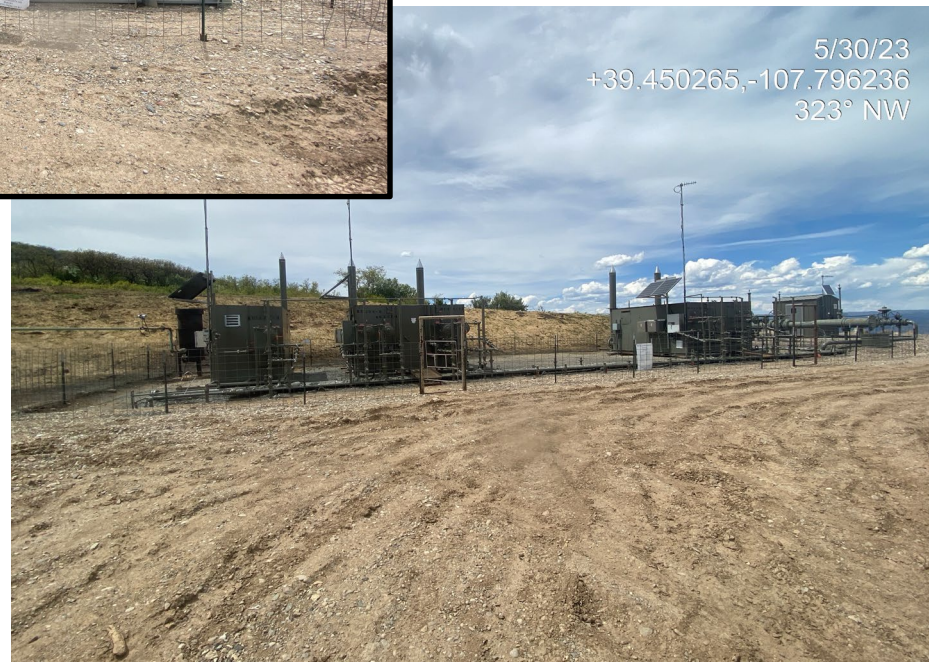
Photo 9. Photos show production areas and the lack of stabilization of the working pad surface.
