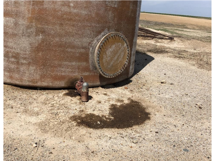
Photo# 4 Stained soil on east side of P/W tank/
