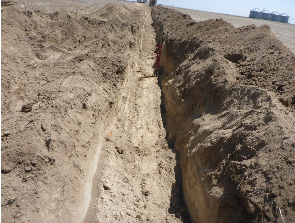
Gulley #1-D Flowline Excavation
