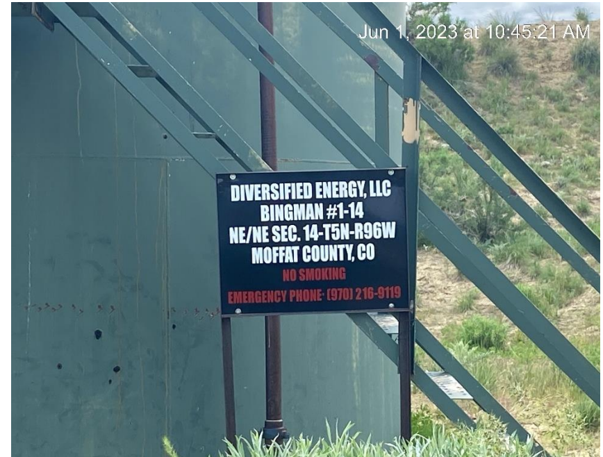
Tank battery sign missing required information
