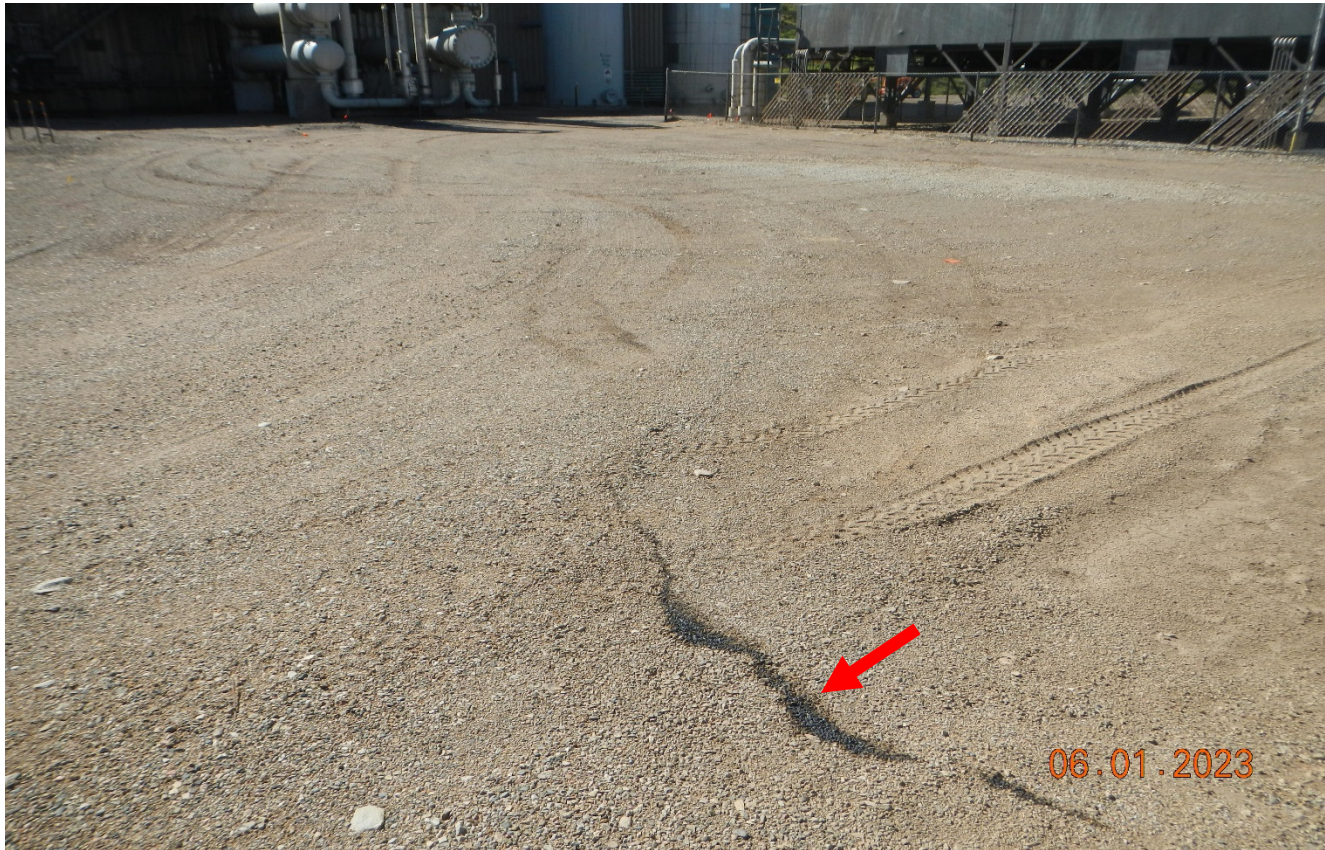
Photo 6. Facing toward the west side of the facility. It appears stormwater has moved impacted material down gradient. There is a line of oil staining at red arrow.
