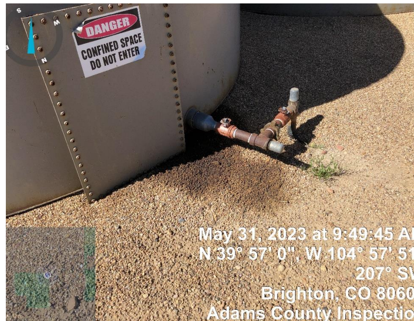
Photo#2 Stained Soil on backside of furthest east production tank
