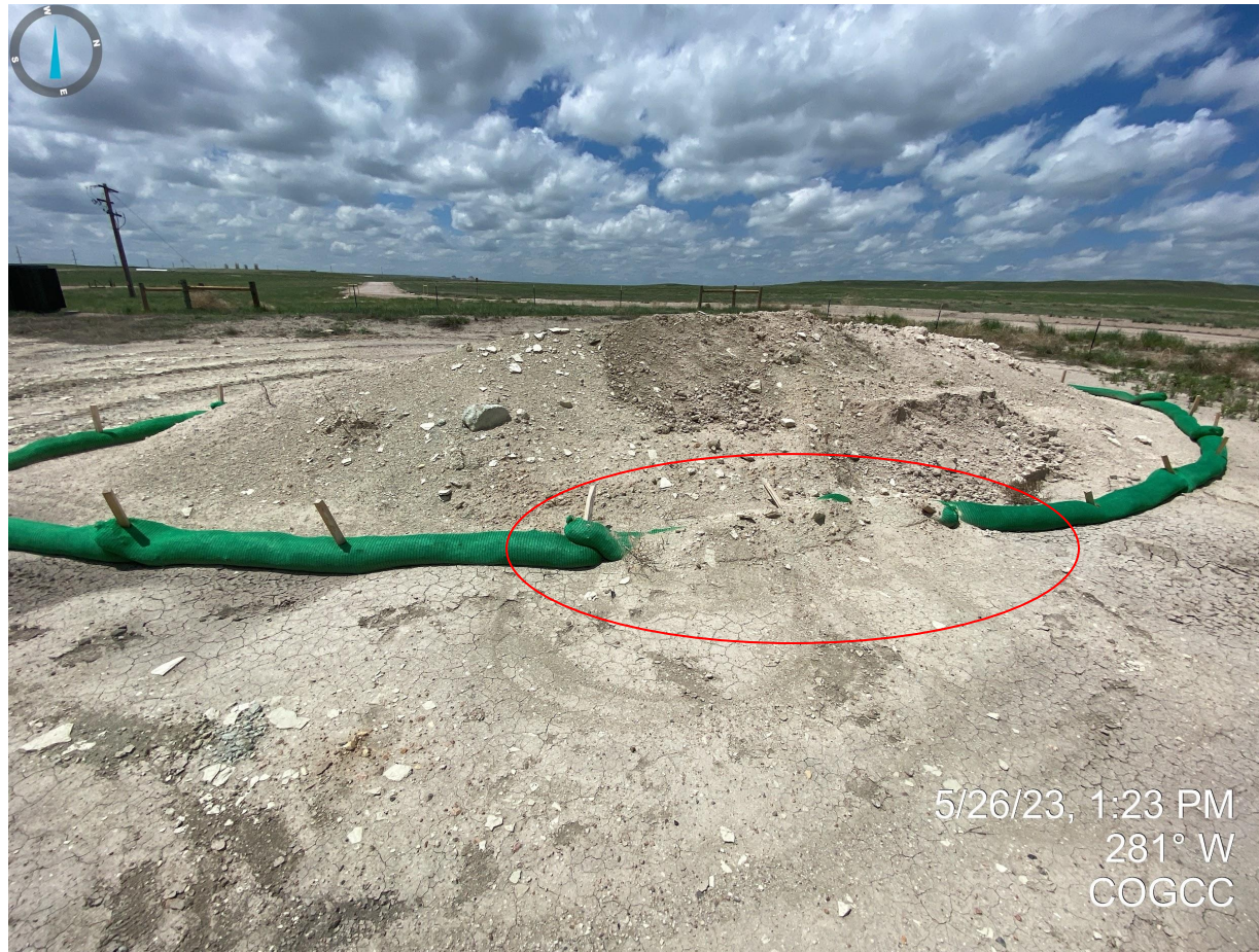
Photo 4. Northern portion of production area. Apparent impacted material being stored on the north end of the location, possibly associated with Remediation Project #29364, was not placed on a impervious liner and sediment control logs appeared inadequate with evidence of sediment transport outside of BMPs. More robust BMPs will need to be implemented to prevent impacted material from migrating outside of containment.
