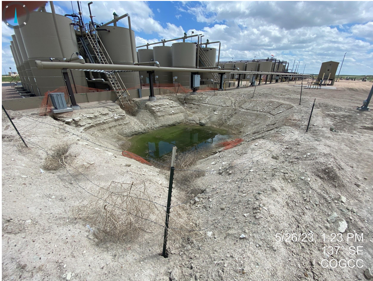
Photo 6. Perimeter fencing around open excavation associated with Remediation Project #29346 appears inadequate to exclude wildlife entry.
