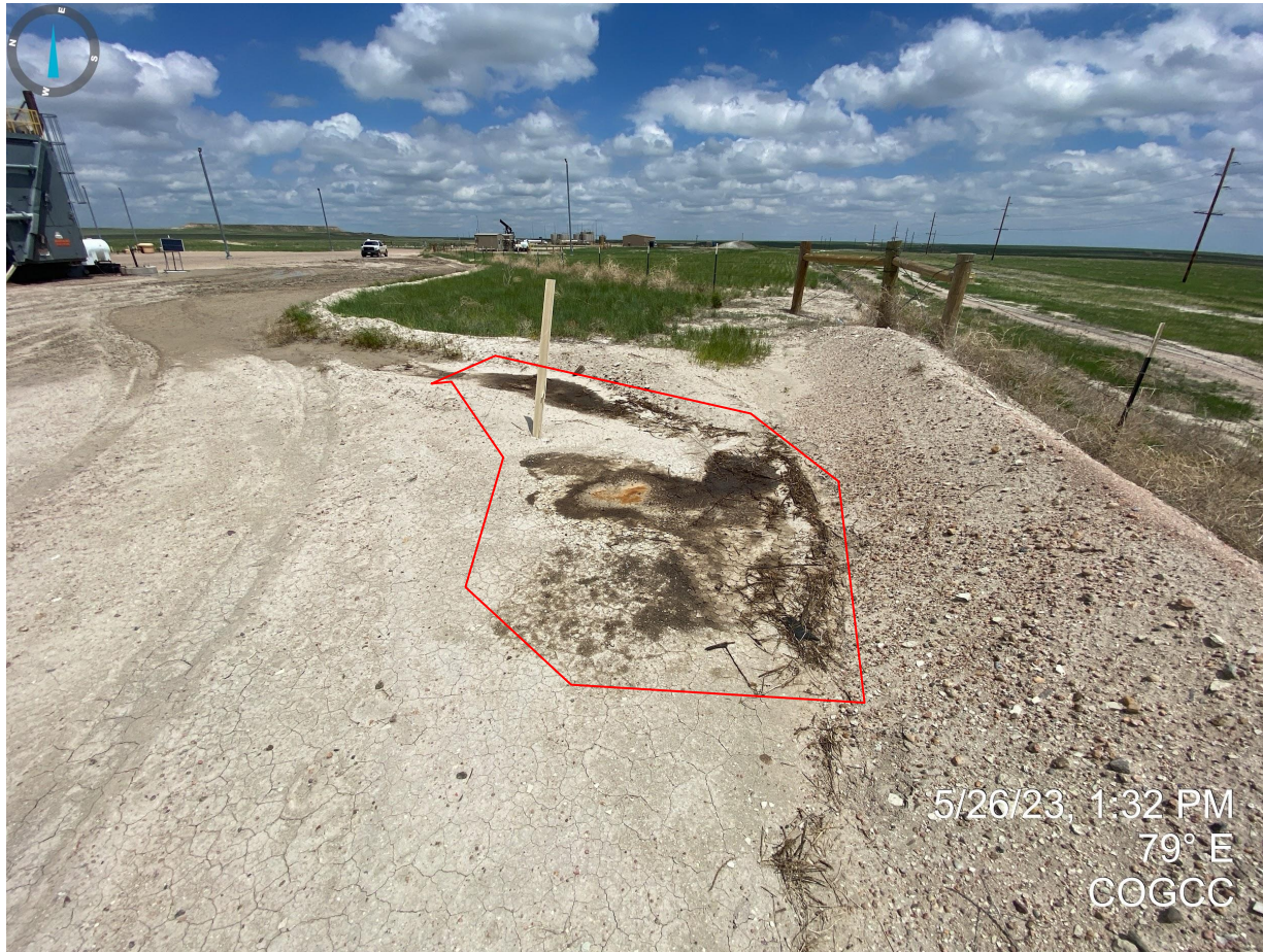
Photo 7. Stained soil observed on the southern end of the location, south of compressors, will need to be properly disposed of in accordance with 905.e.
