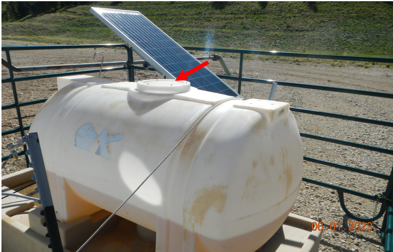
Photo 4. There is no labeling at the tank and there is no lid on the tank
