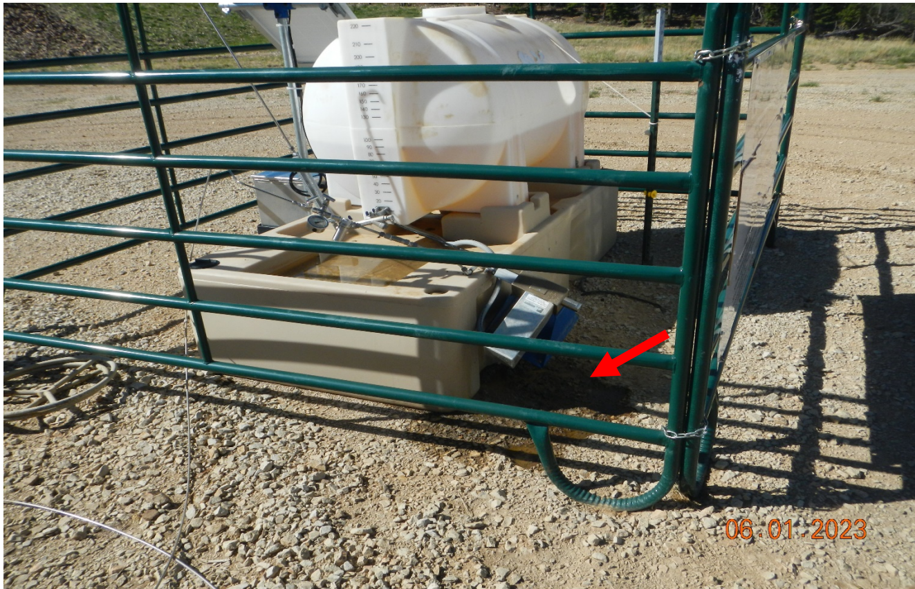
Photo 3. There is a dripping leak coming from the chemical tank line.
