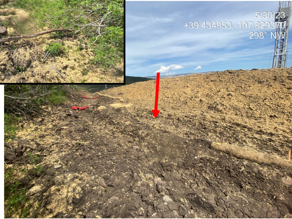
Photo 22. Photos show the topsoil stockpile at the south of the location. Wattles are trenched and backfilled (left). However one wattle is in disrepair and no longer functioning (center, right).
