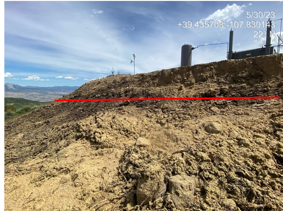
Photo 15. Photo shows the western fill slope during the current inspection. Although Hydromulch has been applied to stabilize topsoil (approximately below the line) BMPs to segregate and protect topsoil from mixing/contamination with the subsoil berm (approximately above the line) are missing/insufficient.
