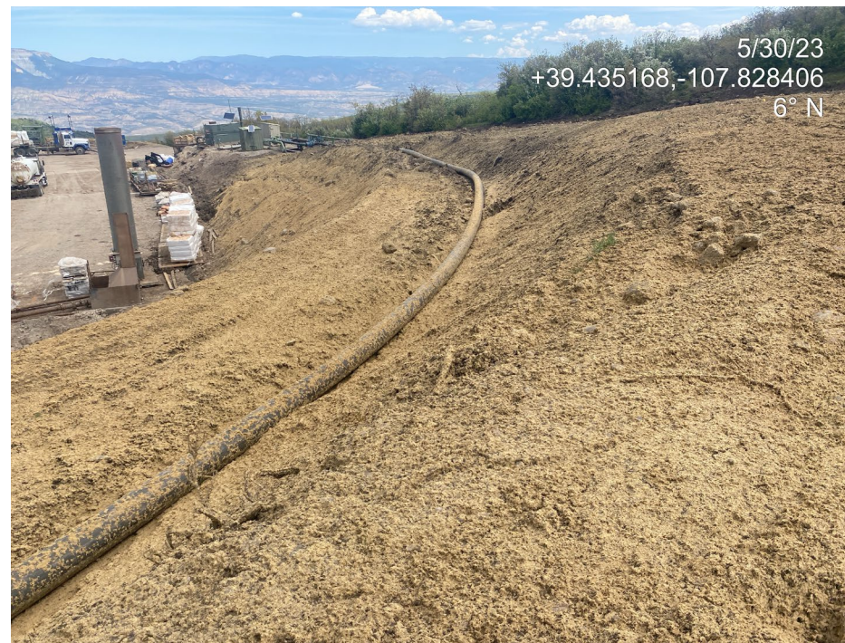
Photo 31. Photos taken from the south shows rill erosion occurring on bare, unprotected, unstabilized slopes in the previous inspection (left) have been stabilized with Hydromulch (right).
