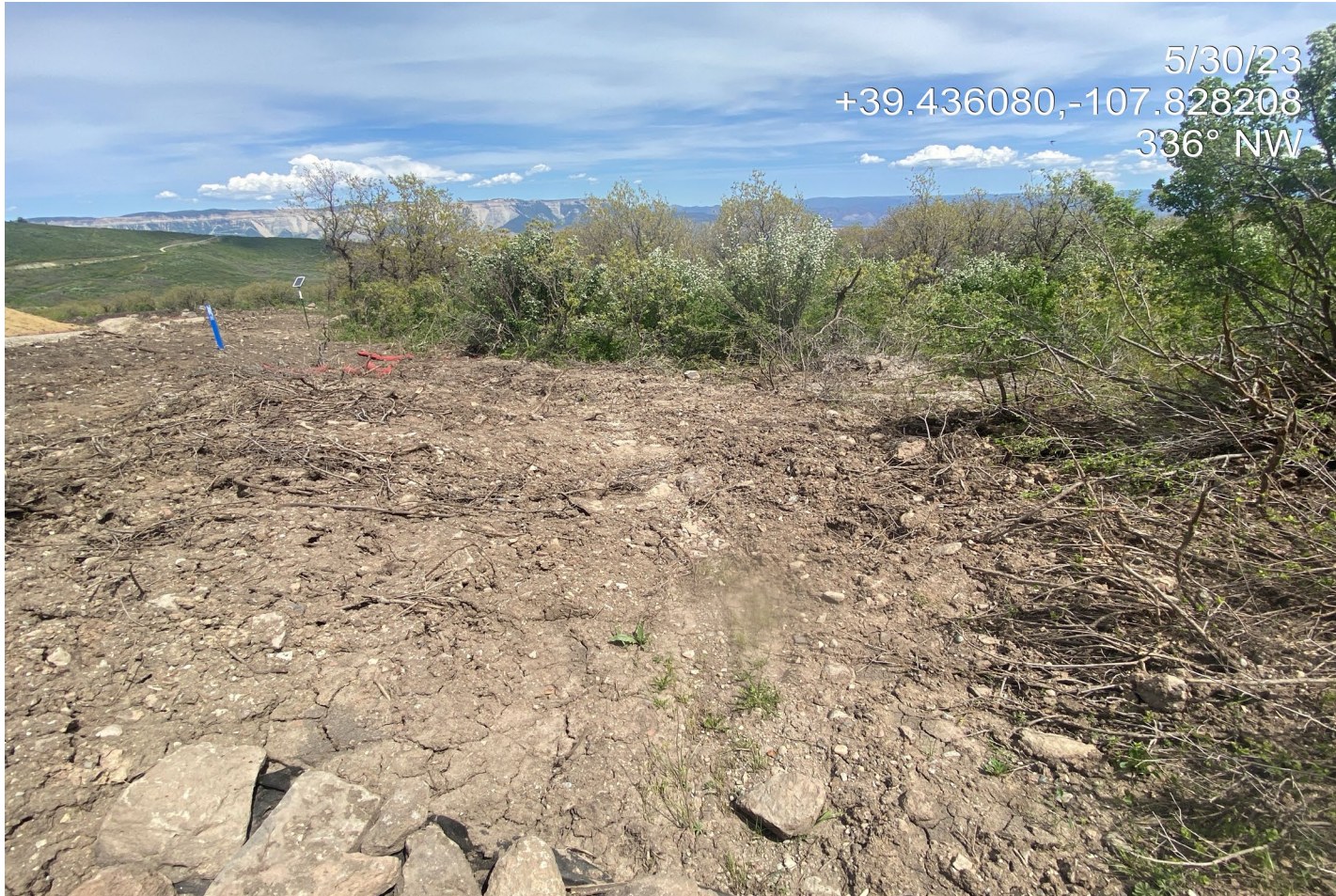
Photo 29. Photo shows the outlet for the sediment trap pictured on the previous slide is discharging stormwater into loose, unconsolidated soil subject to erosion. Photo also shows what appears to be an unpermitted area of disturbance to the east of the access road.
