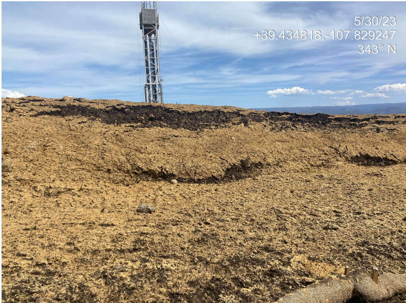
Photo 21. Photo shows degradation of the Hydromulch on a portion of the topsoil stockpile at the south of the location. The Hydromulch is evenly and thoroughly applied to the rest of the topsoil pile.
