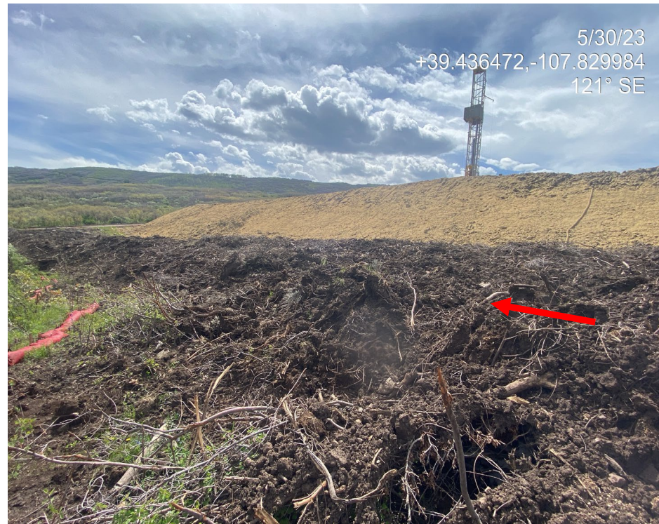
Photo 5. Photo taken from the northern edge of the location during the 5/30/23 inspection shows lack of erosion protections for unconsolidated topsoil.
