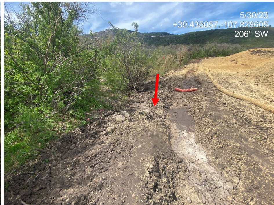
Photo 27. Photos taken from the southeast shows where run-on is breaking through a berm into the perimeter run-on diversion ditch causing degradation to the ditch and berm BMPs. Note also the ditch appears to be constructed from topsoil and is built from loose, unconsolidated martial which is susceptible to erosion from concentrated flows in the ditch.
