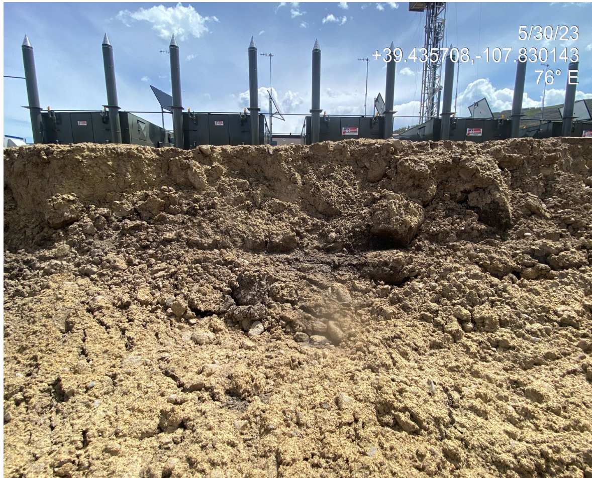
Photo 16. Photo taken from the northwest shows the location perimeter berm is not constructed in accordance with good engineering practice. The berm is loose, unconsolidated, and portions are vertical.
