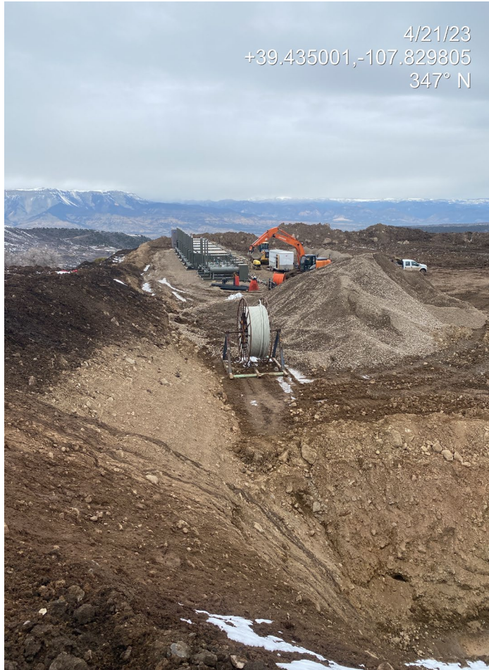
Photo 19. Photo taken from the southwest shows unstabilized and eroding slopes during the previous inspection (left) have been stabilized with Hydromulch (right).
