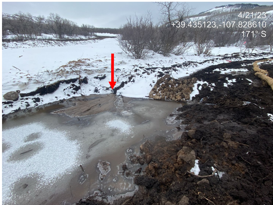
Photo 25. Photo taken from the southeast during the previous inspection shows degradation where stormwater was bypassing an armored inlet to a sediment trap.
