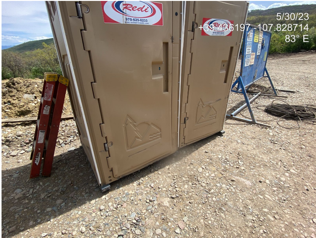
Photo 32. Photos taken from the Location entrance show portable toilets have not been secured to prevent a spill.
