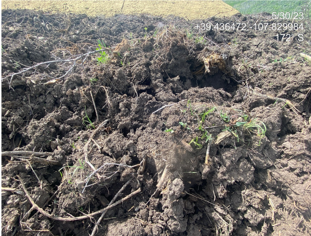
Photo 6. Photo taken from the north shows a close-up of the soil in Photos 4 and 5. The pile appears to contain topsoil. BMPs to protect topsoil from erosion degradation are missing/insufficient.
