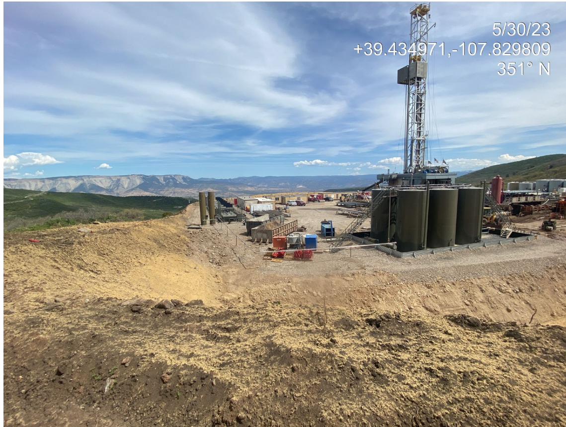
Photo 19. Photo taken from the southwest shows unstabilized and eroding slopes during the previous inspection (left) have been stabilized with Hydromulch (right).
