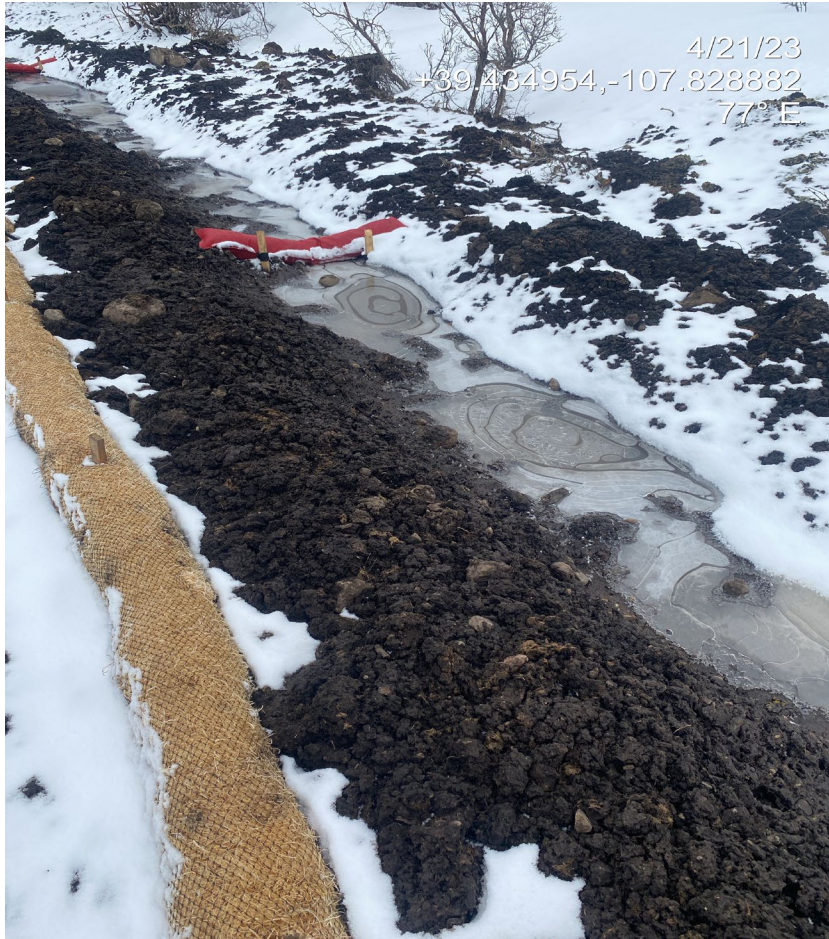
Photo 10. Photo taken from the south during the previous (left) and current (right) inspection. Topsoil does not appear to have been salvaged. Stormwater BMPs appear to be constructed from topsoil. Additionally, the ditch is constructed from loose, unconsolidated material susceptible to erosion from concentrated flows.
