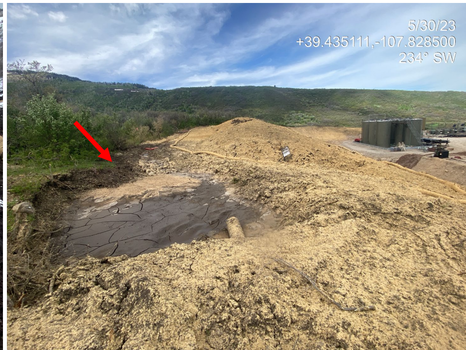
Photo 26. Photo shows the sediment trap pictured in Photo 25 during the current inspection. No controls present to manage run-on which is bypassing an armored inlet to the sediment trap.
