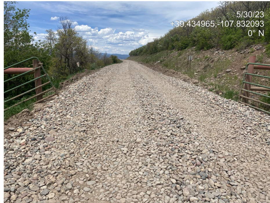
Photo 34. Photos show the location access road directly north of the pad (left) and before it merges with county road 317 (right). Surfaces are stabilized. There is no evidence of sediment tracking.
