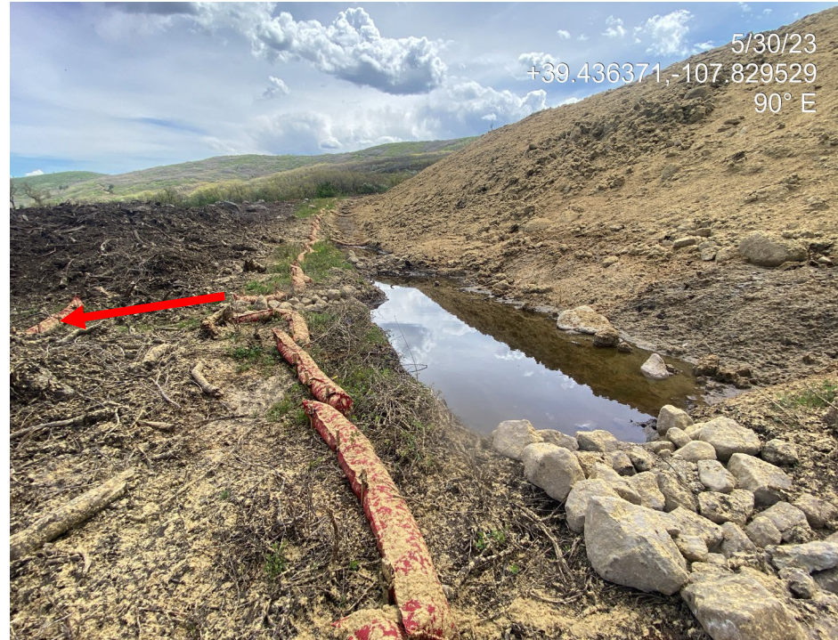
Photo 8. Photos taken from the north during the previous inspection (left) and current inspection (right). Topsoil does not appear to have been salvaged at stormwater BMPs (note presence of intact vegetation). Note also stormwater discharges from a sediment trap into stockpiles which appear to contain topsoil (arrow).
