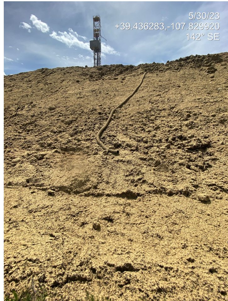
Photo 12. Photos show examples of two (2) slope drains which have not been installed per good engineering practices; the pipe is not properly anchored, the pipe is discharging mid-slope/does not extend beyond the toe of the slope and lacks proper outlet protections.
