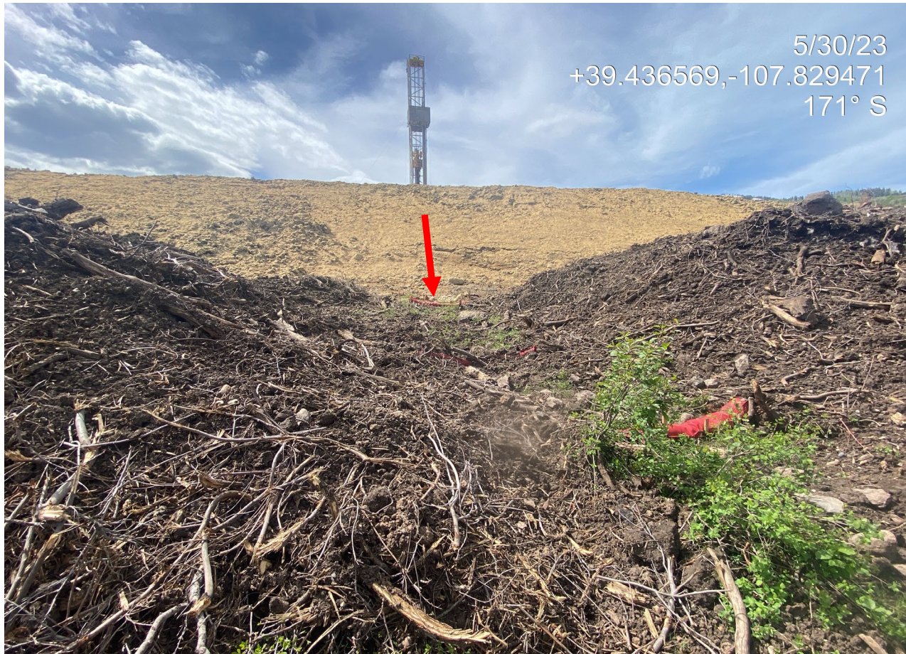
Photo 9. Photo shows where stormwater from a sediment trap (indicated by arrow and shown on previous slide) discharges into a ditch between two stockpiles which appear to contain topsoil. No BMPs present to protect unconsolidated topsoil from concentrated stormwater flows.
