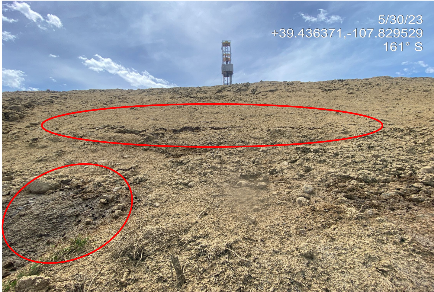
Photo 20. Photo shows fill slopes have been stabilized with Hydromulch. However, slumping of slopes is occurring indicating a lack of stabilization and degrading the Hydromulch coverage.
