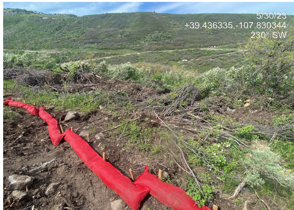
Photo 13. Photo shows perimeter stormwater BMPs at the west of the location previously in disrepair (left) have been properly installed and are in proper functioning condition during the current inspection (right).
