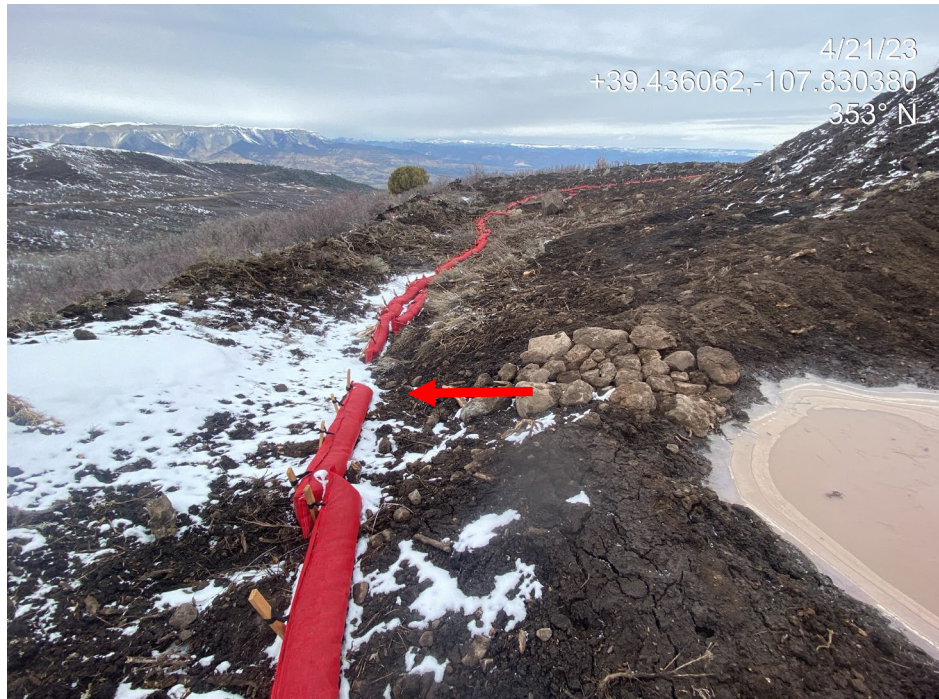
Photo 23. Photo taken during the previous inspection shows a sediment trap to the northwest was designed to discharge stormwater directly into an unvegetated, unstabilized topsoil berm.
