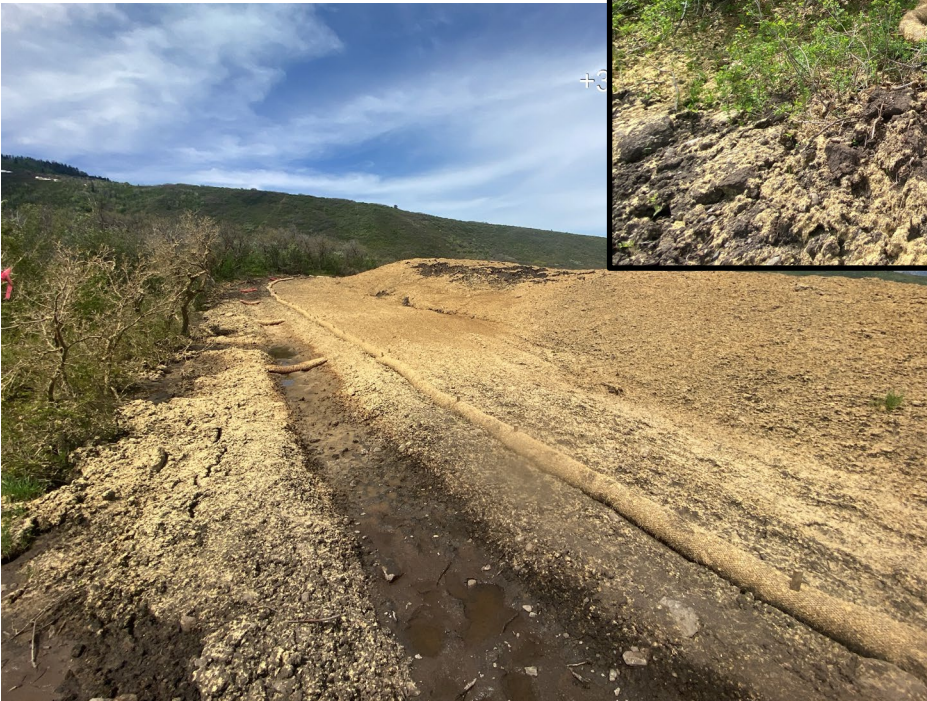
Photo 22. Photos show the topsoil stockpile at the south of the location. Wattles are trenched and backfilled (left). However one wattle is in disrepair and no longer functioning (center, right).
