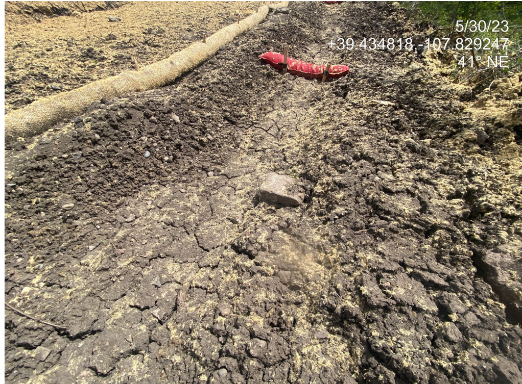
Photo 10. Photo taken from the south during the previous (left) and current (right) inspection. Topsoil does not appear to have been salvaged. Stormwater BMPs appear to be constructed from topsoil. Additionally, the ditch is constructed from loose, unconsolidated material susceptible to erosion from concentrated flows.
