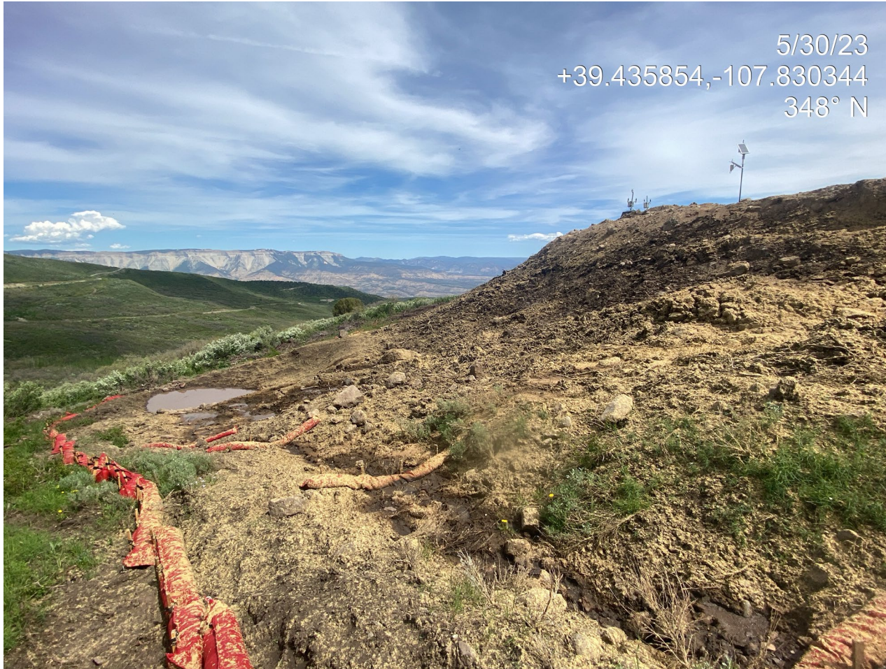
Photo 7. Photo taken from the northwest. Topsoil does not appear to have been salvaged at stormwater BMPs (note presence of intact vegetation).
