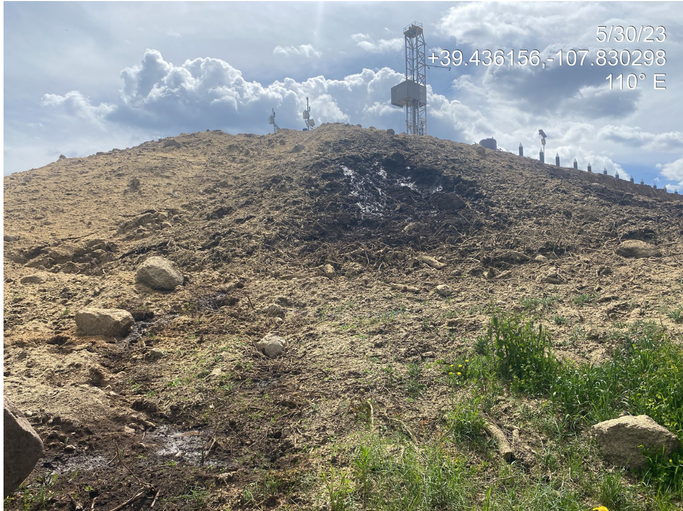
Photo 17. Photo shows a slump that has occurred in the northwest fill slope of the location.
