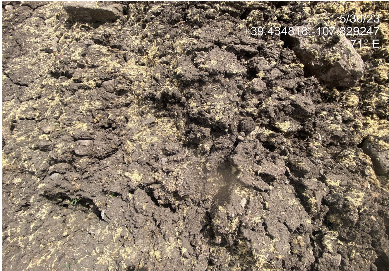
Photo 11. Photo shows a close-up of the ditch pictured on the previous slide. The ditch has not been stabilized and constructed per good engineering practices; soils are loose and unconsolidated and susceptible to erosion from concentrated flows.
