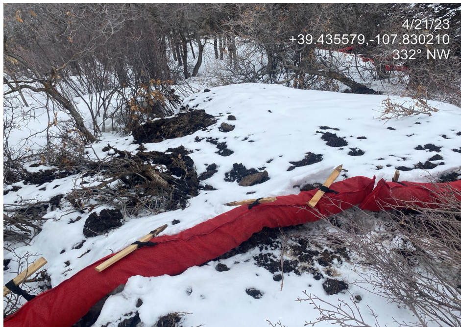
Photo 13. Photo shows perimeter stormwater BMPs at the west of the location previously in disrepair (left) have been properly installed and are in proper functioning condition during the current inspection (right).
