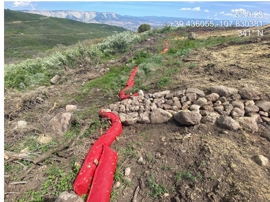
Photo 24. Photo taken during the current inspection shows the sediment trap is now discharging stormwater offsite into a vegetated, stabilized area.
