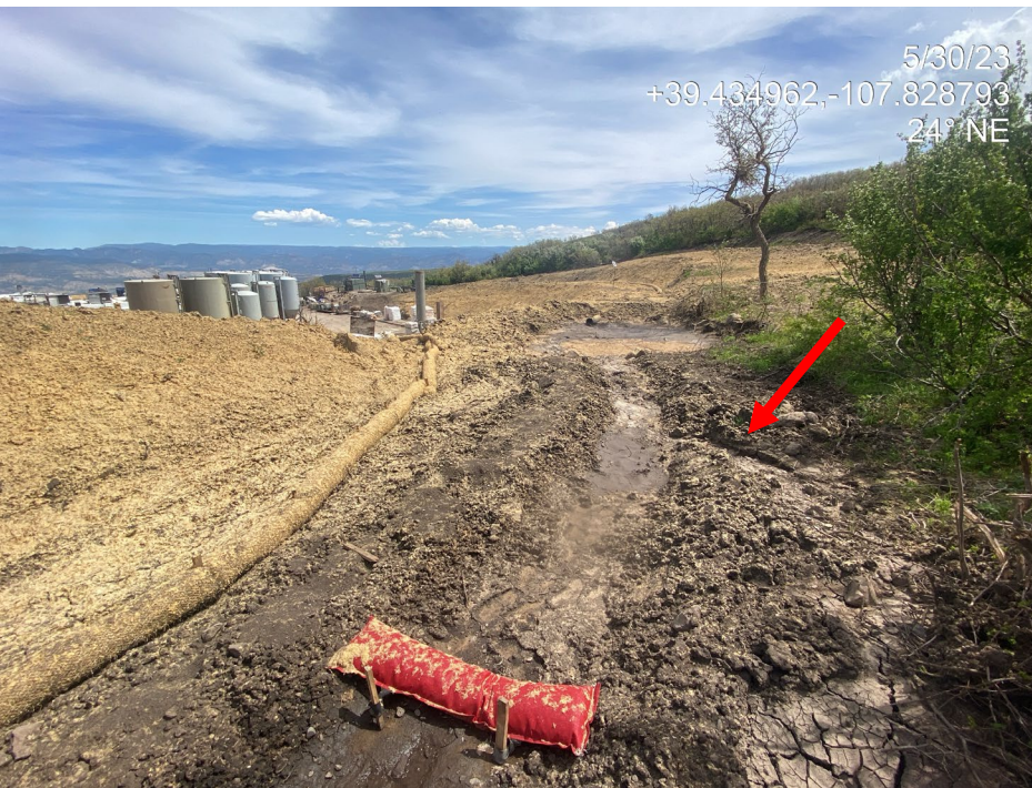
Photo 27. Photos taken from the southeast shows where run-on is breaking through a berm into the perimeter run-on diversion ditch causing degradation to the ditch and berm BMPs. Note also the ditch appears to be constructed from topsoil and is built from loose, unconsolidated martial which is susceptible to erosion from concentrated flows in the ditch.
