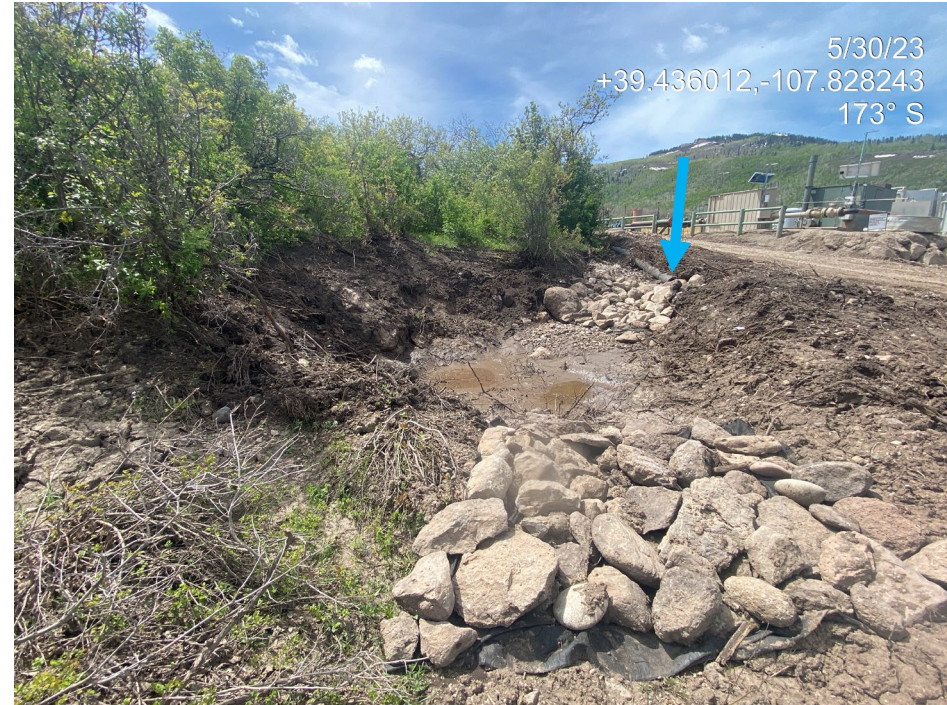
Photo 28. Photo taken from the east shows a drain discharging concentrated stormwater flows without outlet protections during the previous inspection (left). During the current inspection, flows are diverted under the road and discharged to the east of the road at an armored outlet into a sediment trap (right). Note also sediment trap walls appear to be constructed from topsoil and are loose and unconsolidated and susceptible to erosion. This pipe diversion, and sediment trap on the east of the road appears to be outside the permitted disturbance area for the location.
