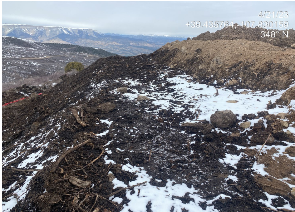
Photo 14. Photo shows the western fill slope during the previous inspection. BMPs to segregate and protect topsoil from mixing with the lighter colored subsoil berm are missing/insufficient. Additionally, topsoil is bare, loose and unconsolidated and susceptible to erosion.
