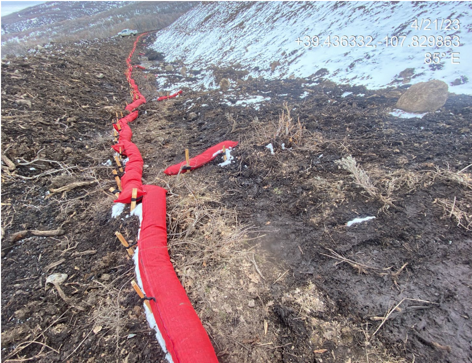
Photo 8. Photos taken from the north during the previous inspection (left) and current inspection (right). Topsoil does not appear to have been salvaged at stormwater BMPs (note presence of intact vegetation). Note also stormwater discharges from a sediment trap into stockpiles which appear to contain topsoil (arrow).
