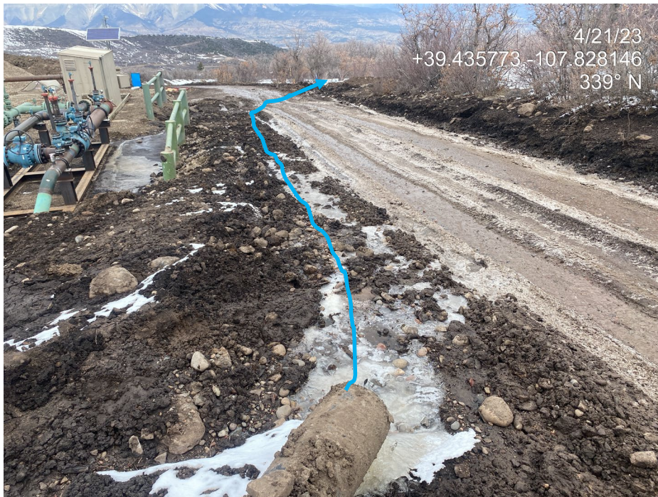
Photo 28. Photo taken from the east shows a drain discharging concentrated stormwater flows without outlet protections during the previous inspection (left). During the current inspection, flows are diverted under the road and discharged to the east of the road at an armored outlet into a sediment trap (right). Note also sediment trap walls appear to be constructed from topsoil and are loose and unconsolidated and susceptible to erosion. This pipe diversion, and sediment trap on the east of the road appears to be outside the permitted disturbance area for the location.
