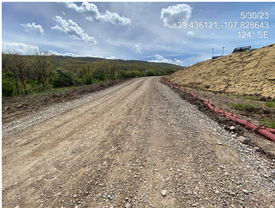
Photo 34. Photos show the location access road directly north of the pad (left) and before it merges with county road 317 (right). Surfaces are stabilized. There is no evidence of sediment tracking.
