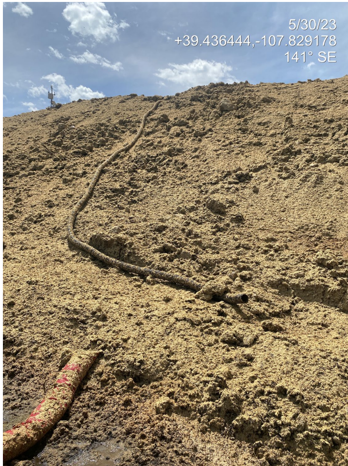
Photo 12. Photos show examples of two (2) slope drains which have not been installed per good engineering practices; the pipe is not properly anchored, the pipe is discharging mid-slope/does not extend beyond the toe of the slope and lacks proper outlet protections.
