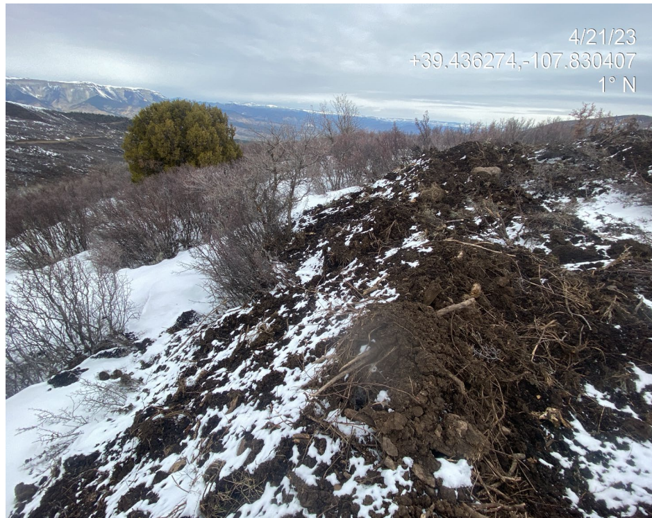
Photo 4. Photo taken from the northwestern edge of the location during the previous inspection shows lack of erosion protections for unconsolidated topsoil.
