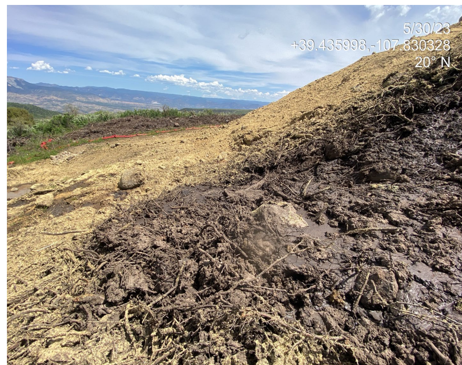
Photo 18. Photos show the top (left) and base (right) of a slump that has occurred in the northwest fill slope of the location.
