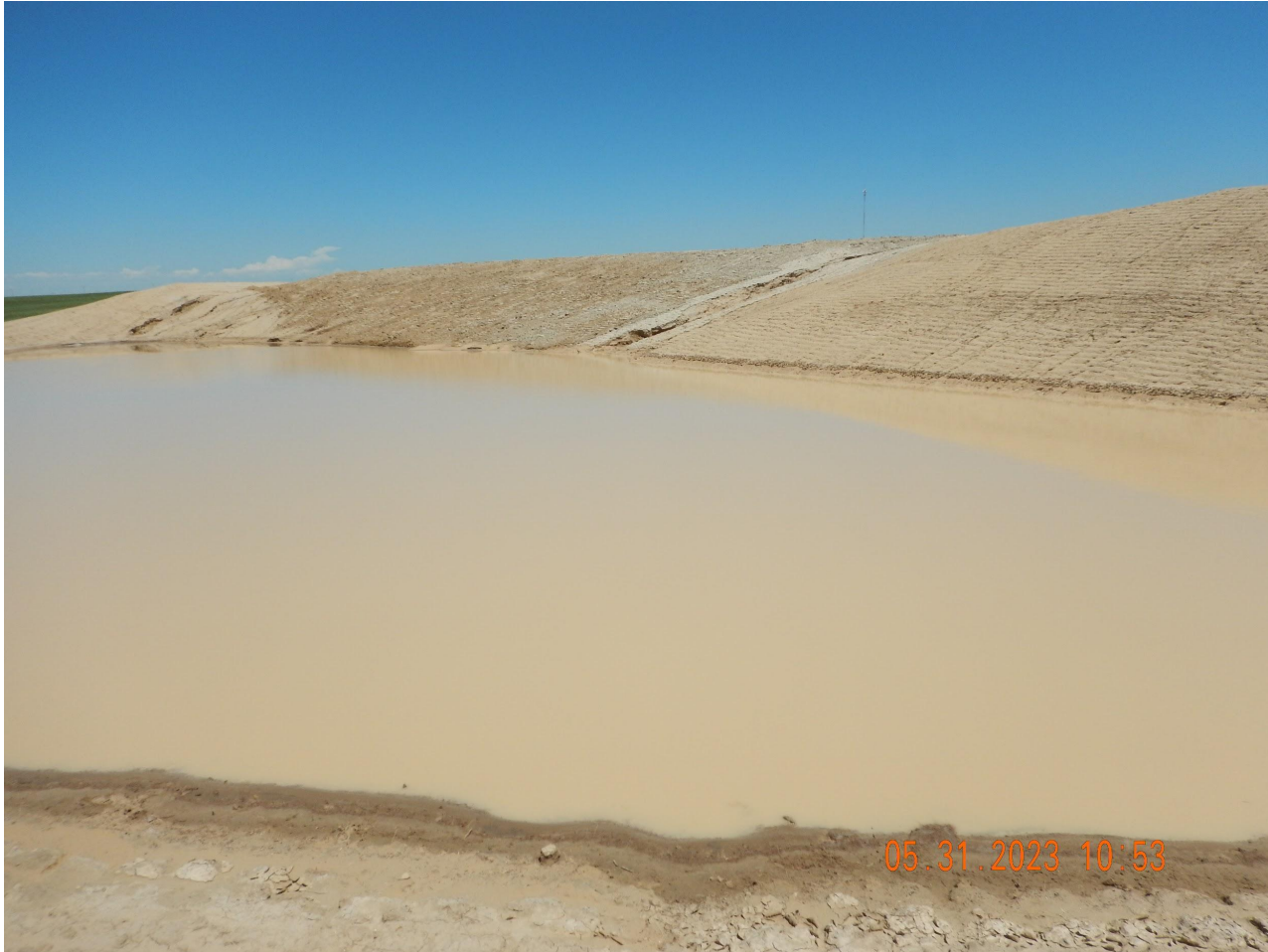
Photo 4. Photo taken from the sediment basin, facing North. Photo illustrates gully erosion is evident and in need of repair.
