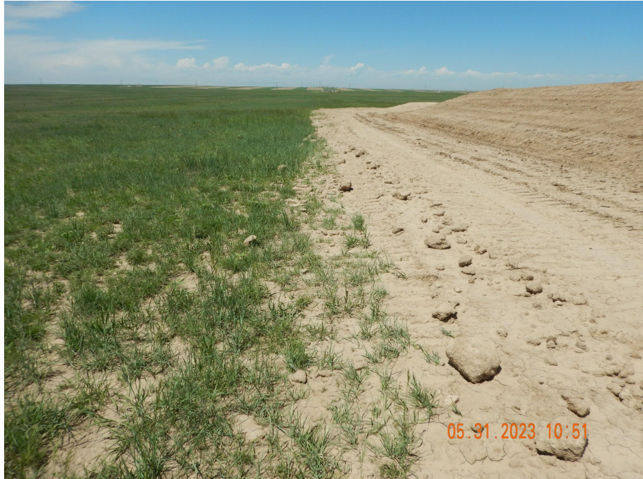
Photo 3. Photo taken from the southern perimeter of location, facing West. Photo illustrates there is no perimeter stormwater BMP.
