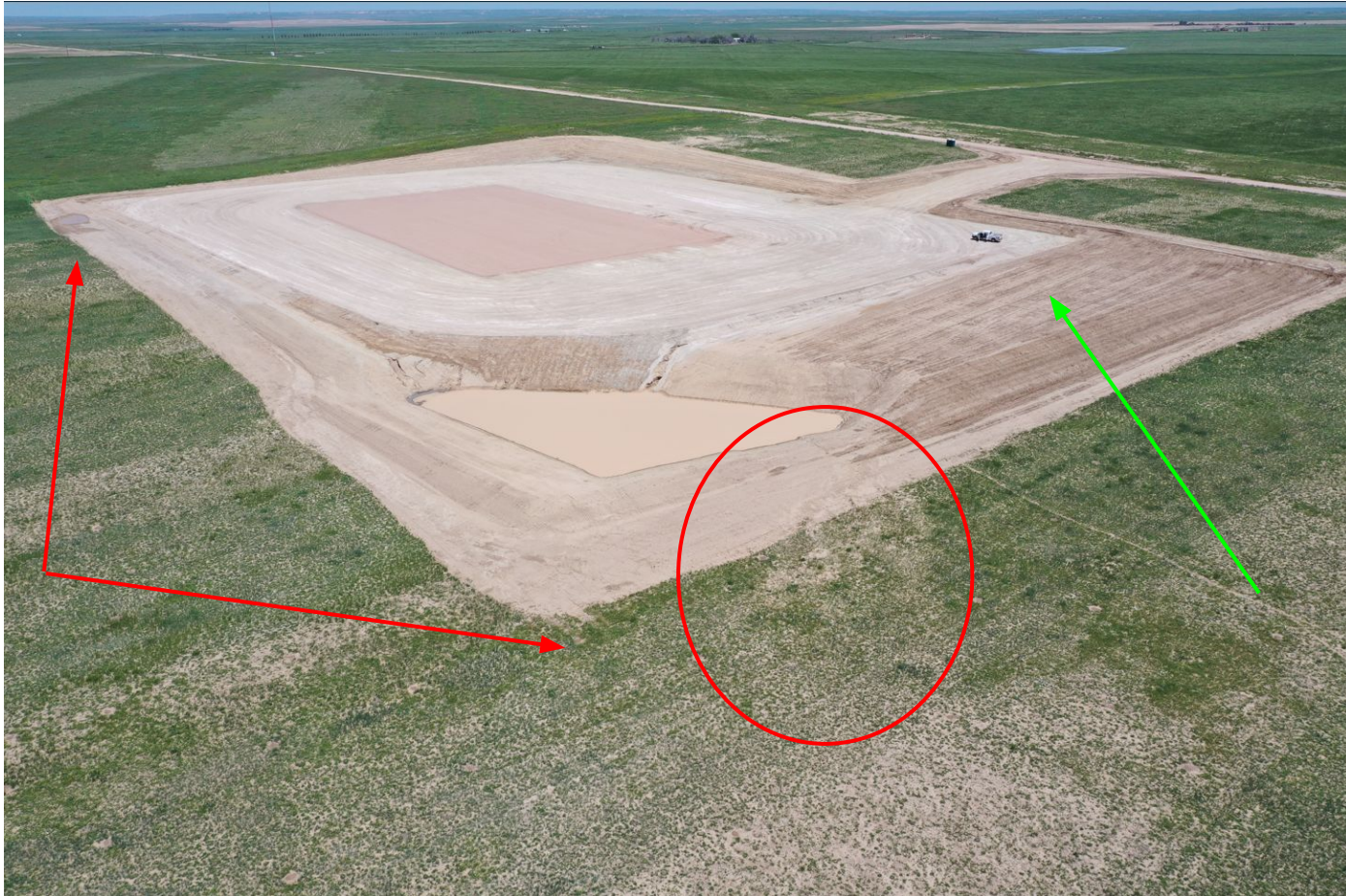
Photo 1. Drone imagery illustrates the location, facing Northeast. At the time of this inspection, there were no perimeter stormwater BMPs along the southern and western perimeter. The sediment basin overflowed and sediment laden stormwater discharged along the southwestern perimeter (red circle). Areas of sediment laden stormwater also discharged along the western perimeter (red arrows). Topsoil has been stockpiled along the southern location- green arrow.
