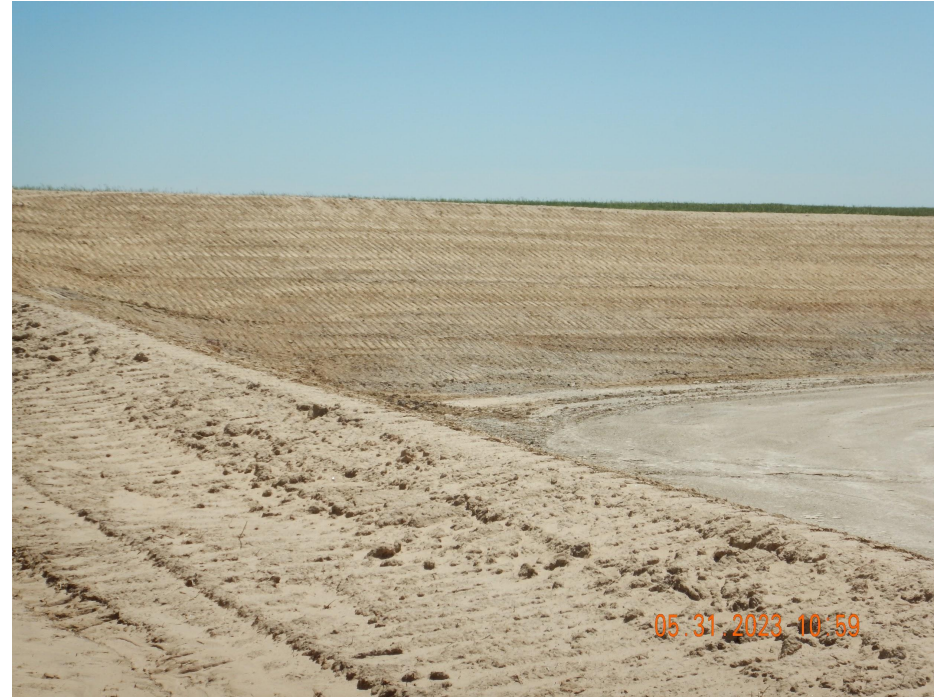
Photo 8. Photo taken from the northern perimeter of location, facing East. Photo illustrates the cut slope has temporarily stabilized; however, the equipment tracking was not conducted perpendicular to the slope.
