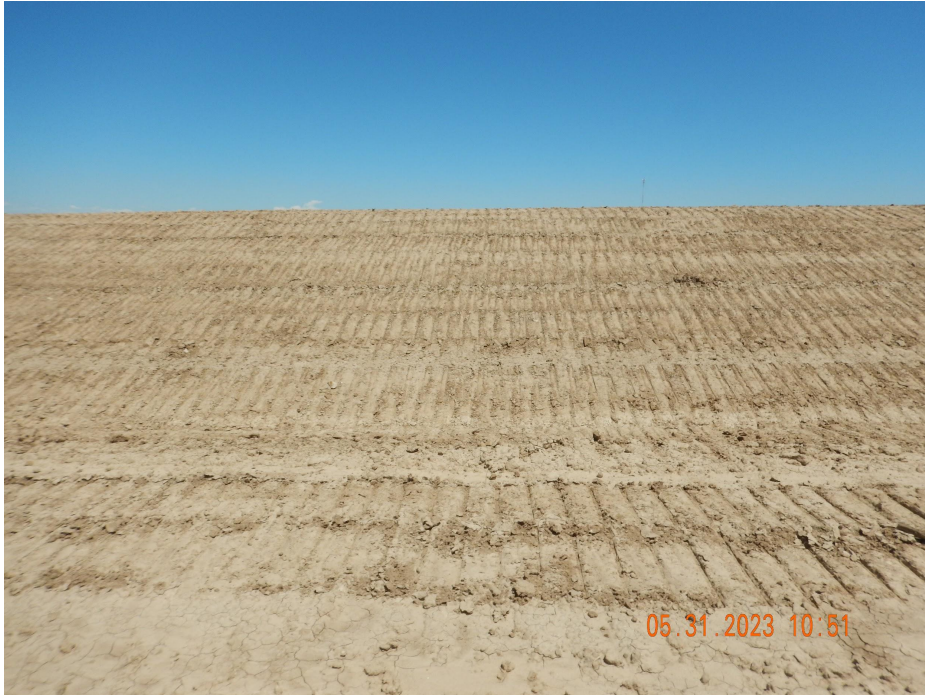
Photo 2. Photo taken from the southern location on the topsoil stockpile, facing North. Photo illustrates the stockpile has been temporarily stabilized; however, the equipment tracking was not conducted perpendicular to the slope.
