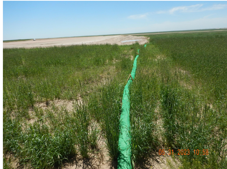
Photo 6. Photo taken from the northwestern perimeter of location, facing South. Photo illustrates a perimeter stormwater BMP that extends along the northern perimeter where there has been no oil and gas disturbance.
